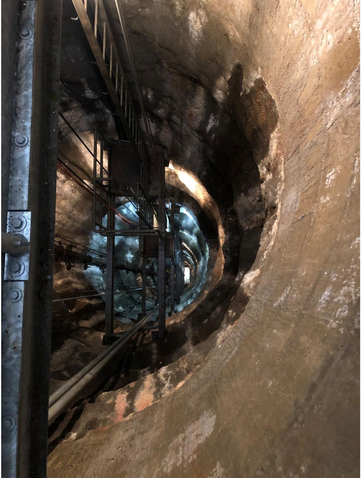
Gate Shaft Access Ladder System
