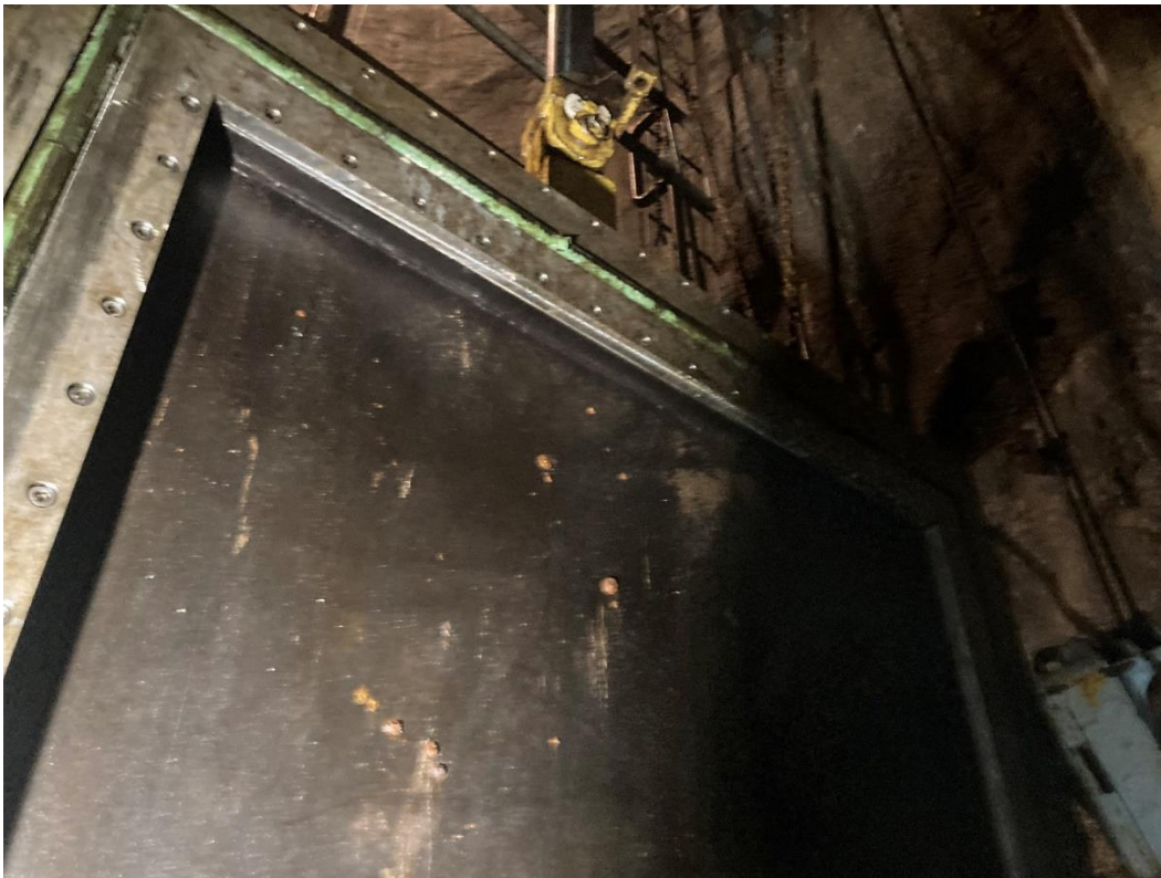
Gate Downstream Face Seal
