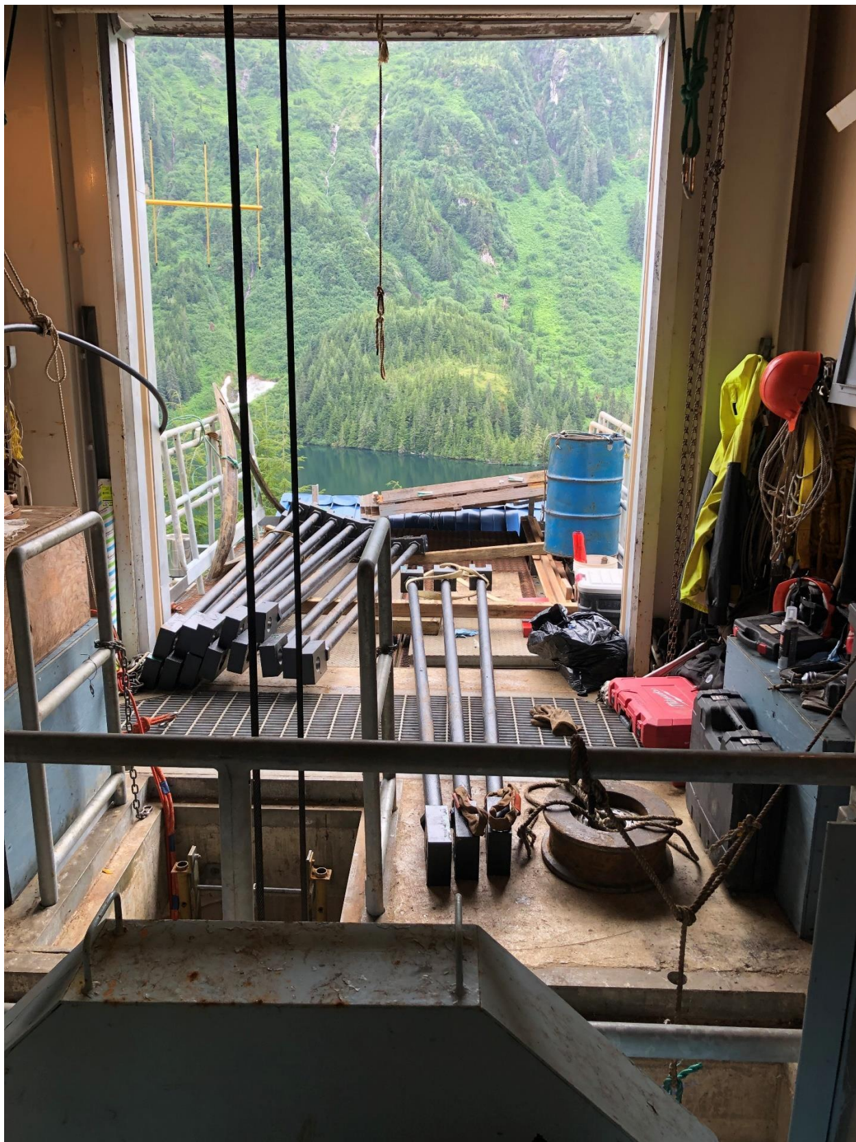
New gate stems staged to lower down gate shaft
