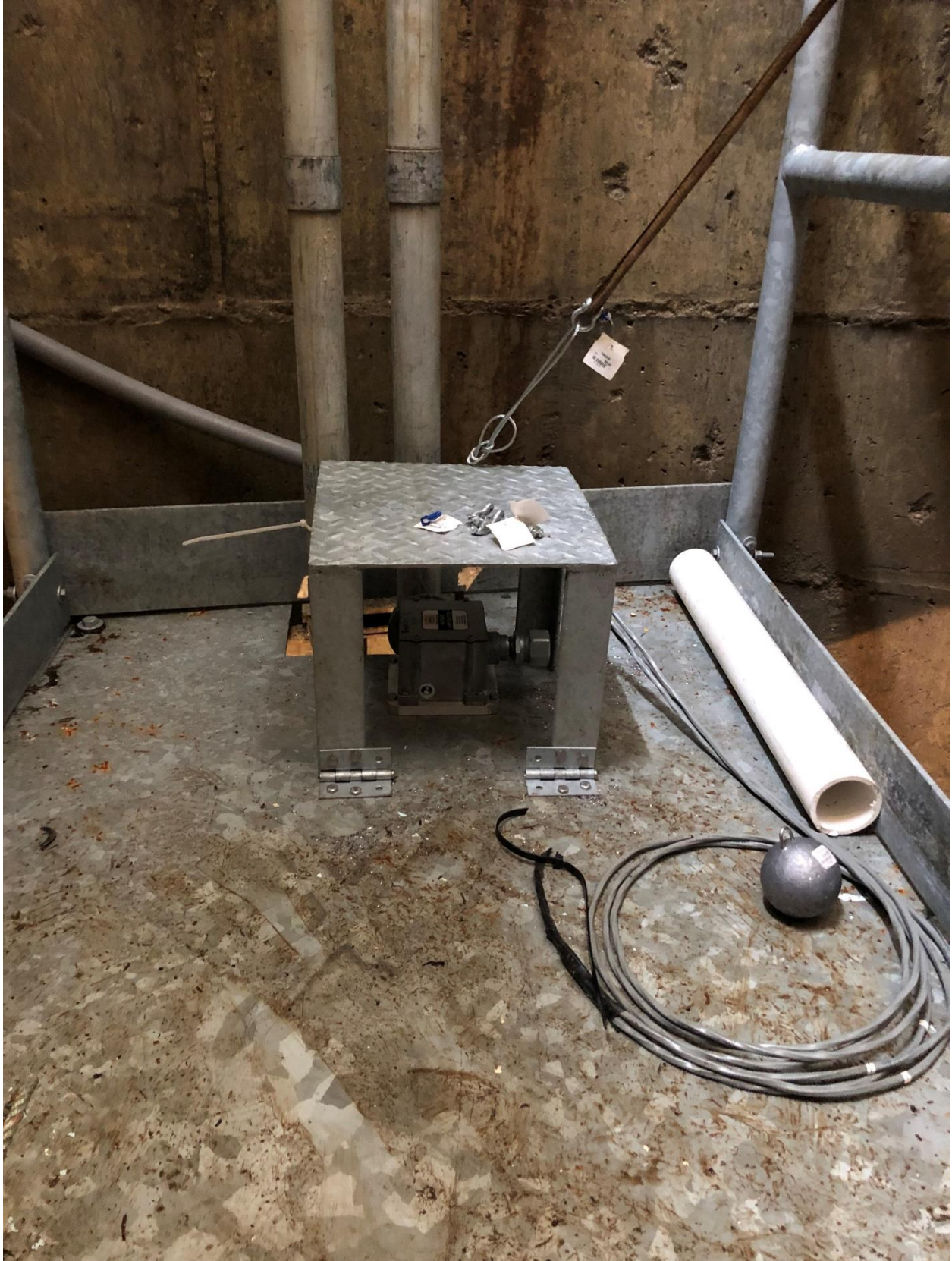
HPU Limit Switch installed at 1610' deck
