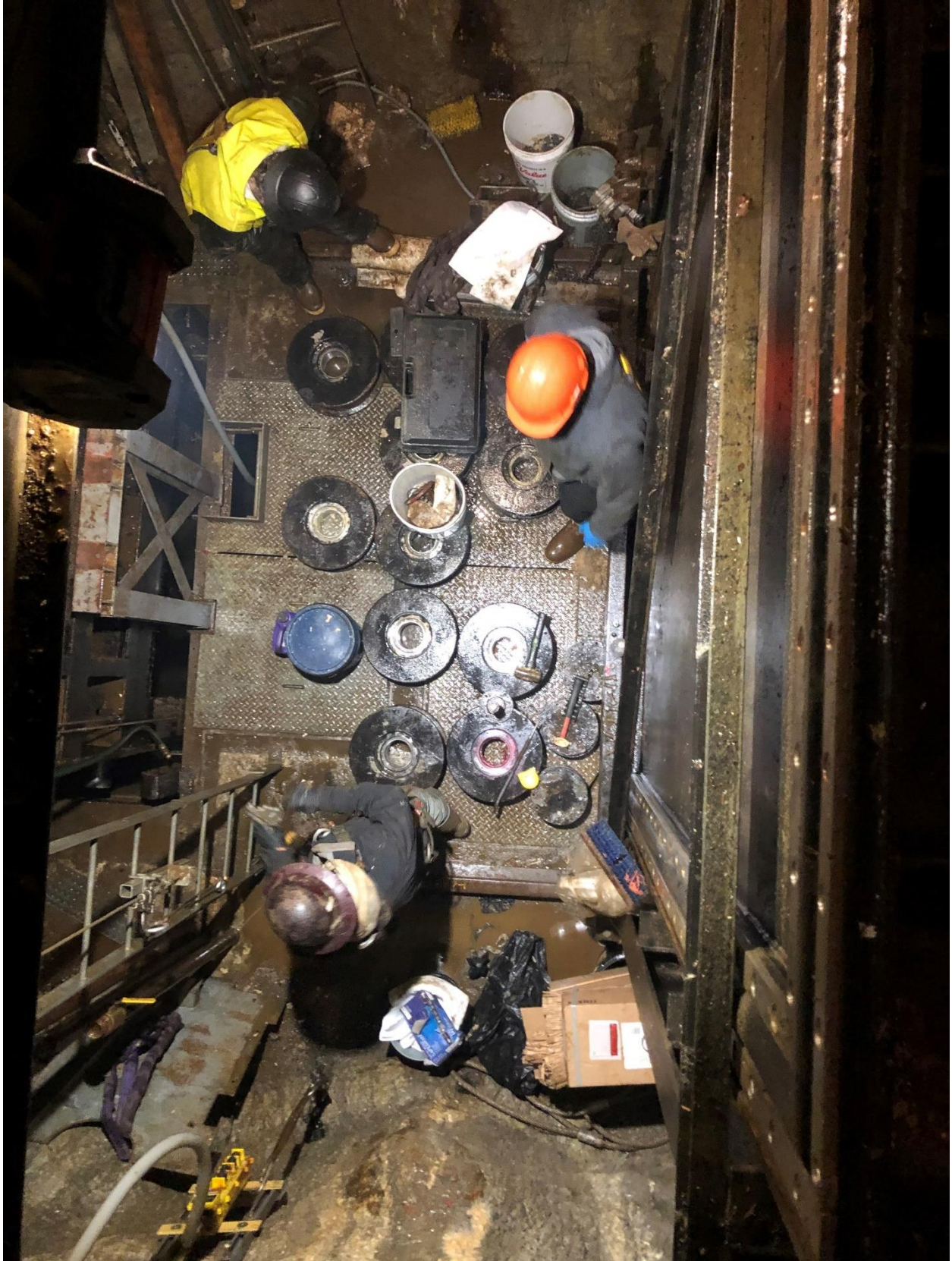
Rebuilding gate guide rollers at elevation 1417' Maintenance Deck
