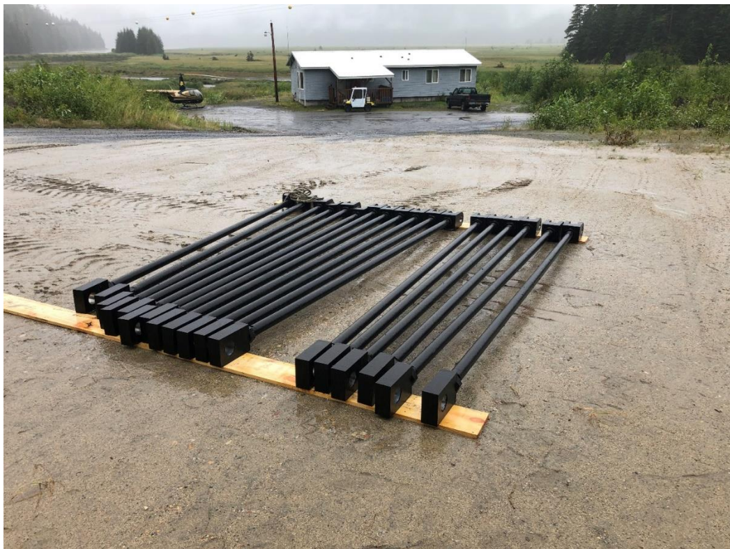
New gate stems staged for transfer via helicopter to the Gatehouse
