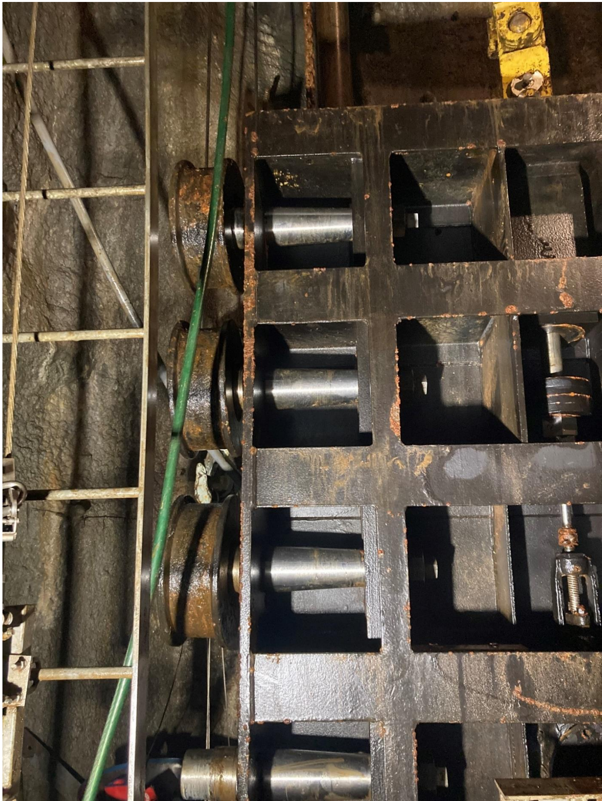
Tyee Gate disassembly of guide rollers
