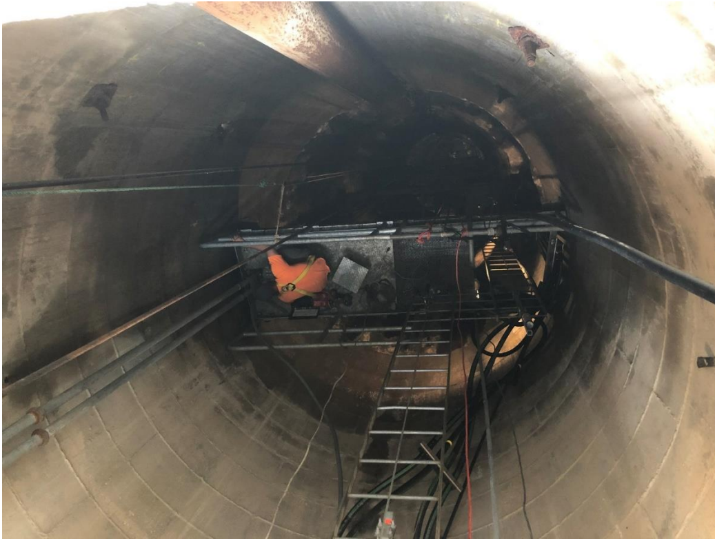
Installing Limit Switch 1610' Deck
