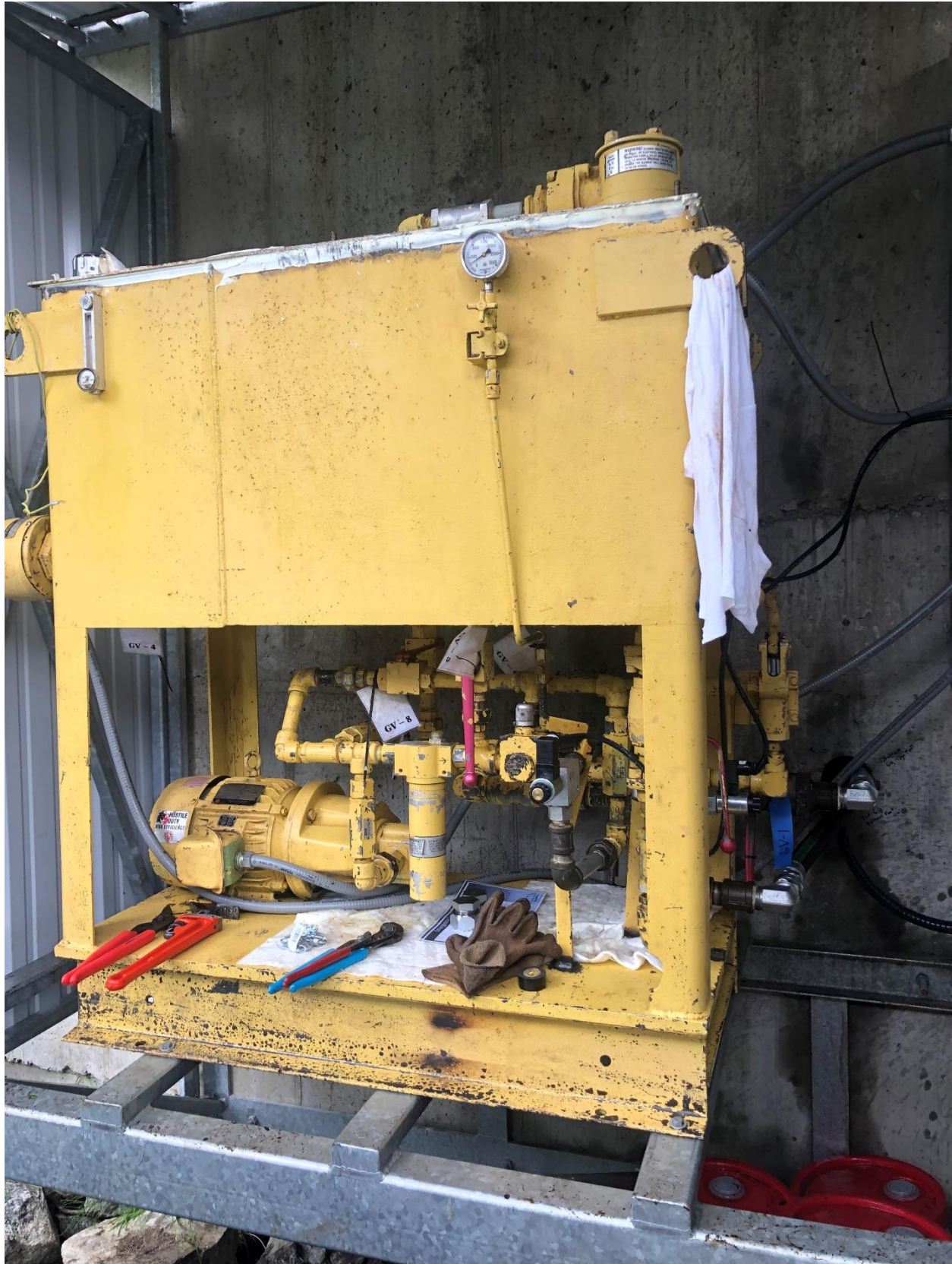
Intake Gate HPU at new ground level elevation 1615'
