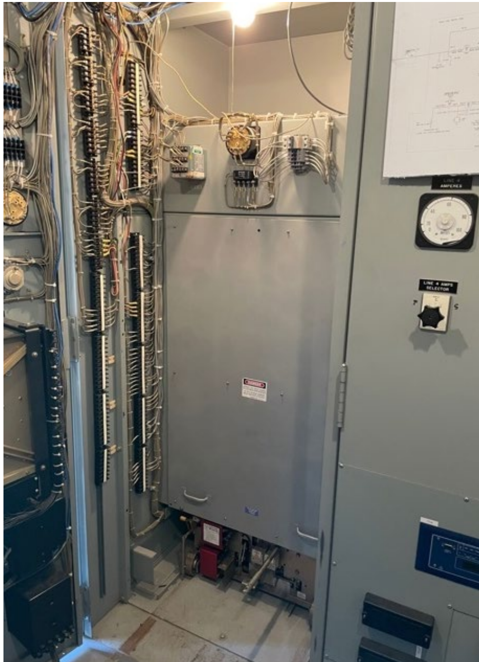
Wrangell Substation Westinghouse Type 150 DHS Circuit Breaker Circa 1983
