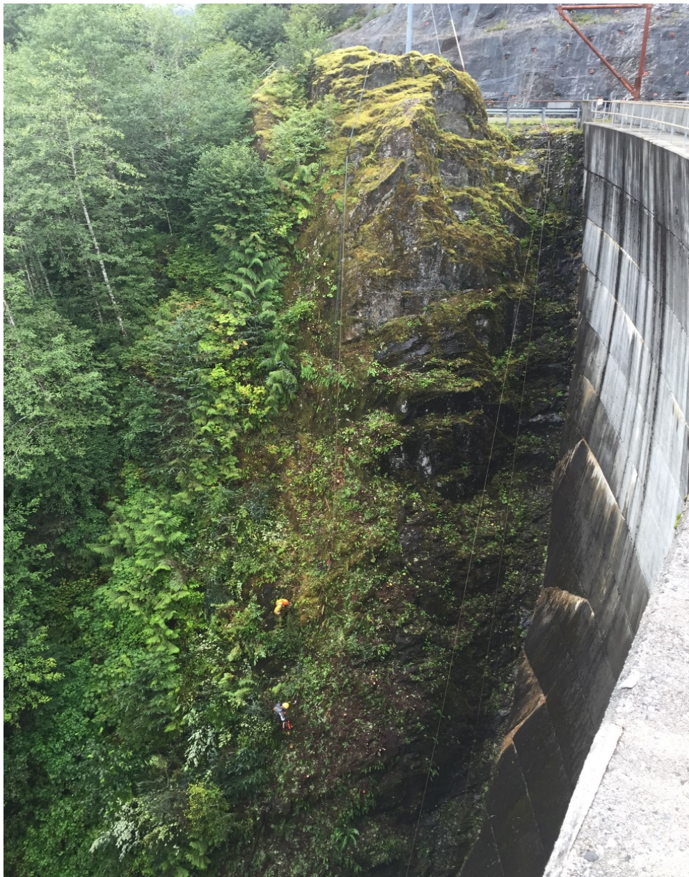
Swan Lake Dam Abutment Clearing 30' from Dam
