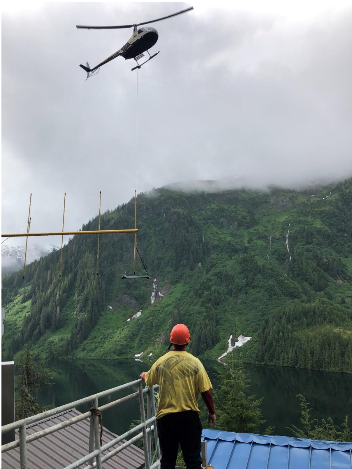
Transferring new gate stems to Gatehouse
