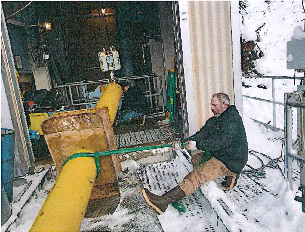
Moving Cylinder from Staging Deck into Gatehouse
