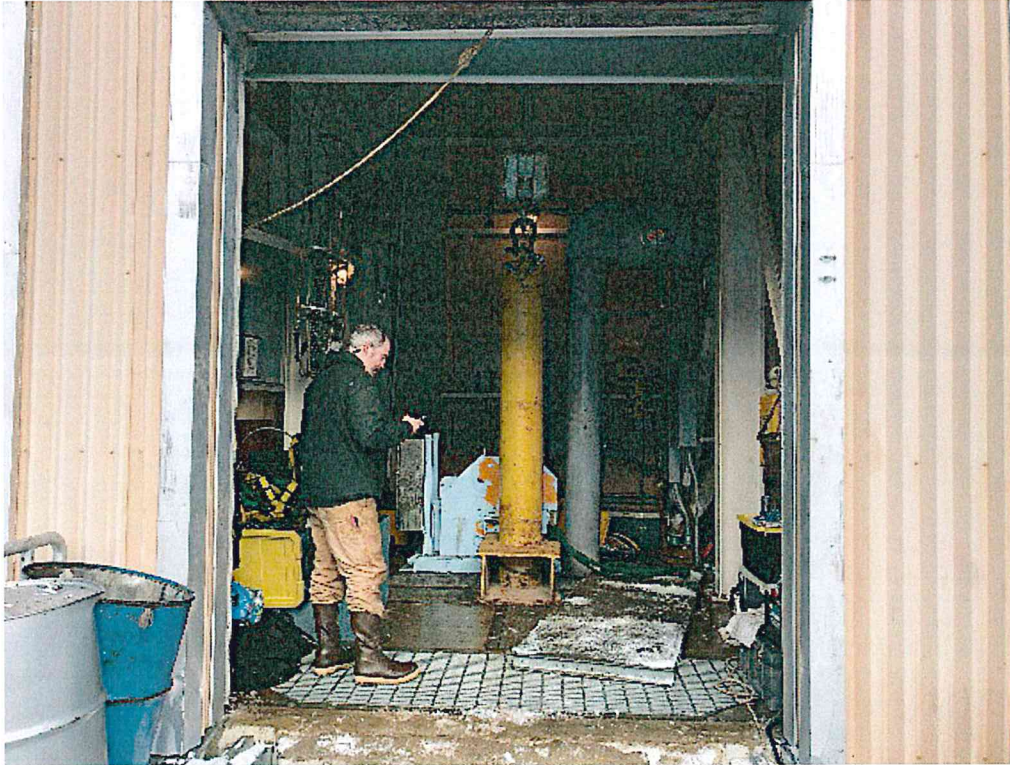
Cylinder started down Gate Shaft
