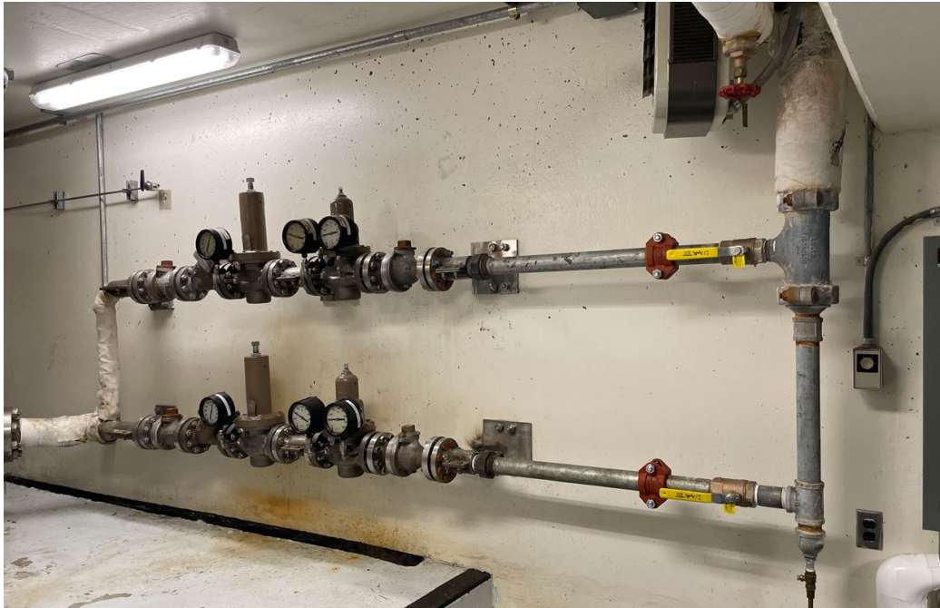
New PRV Valves in place; note high-pressure couplers and new Isolation Valves
