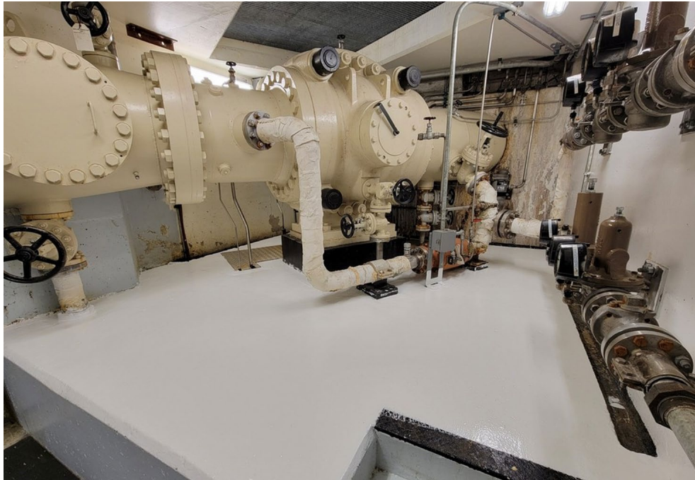
Newly Painted Turbine Shutoff Valve Pit
