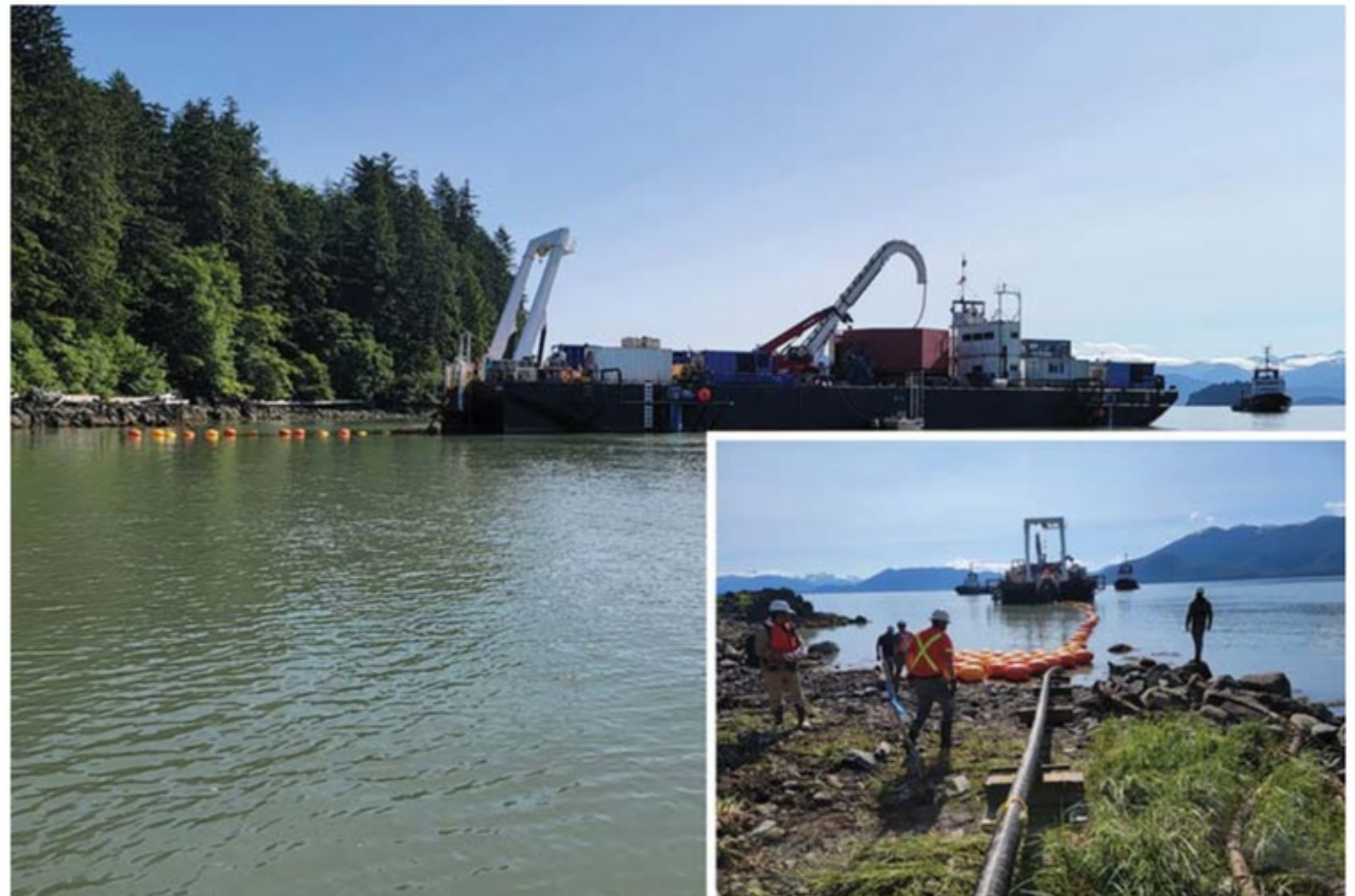
Installation of the 69 kV XLPE insulated cable, Vank Island, Alaska. Photos by SEAPA.
