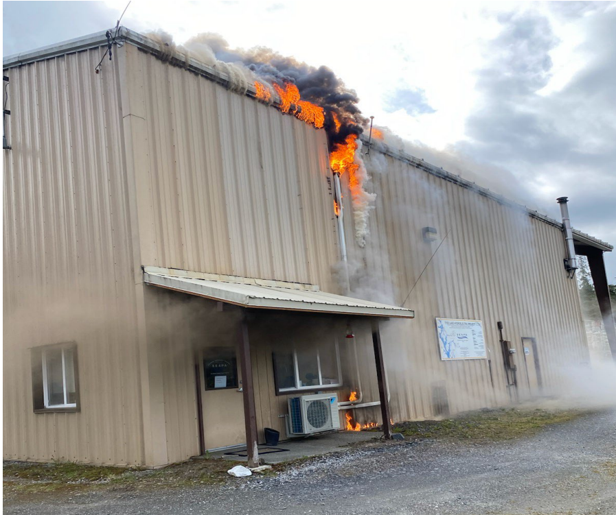
Fire bleeding through to exterior.
