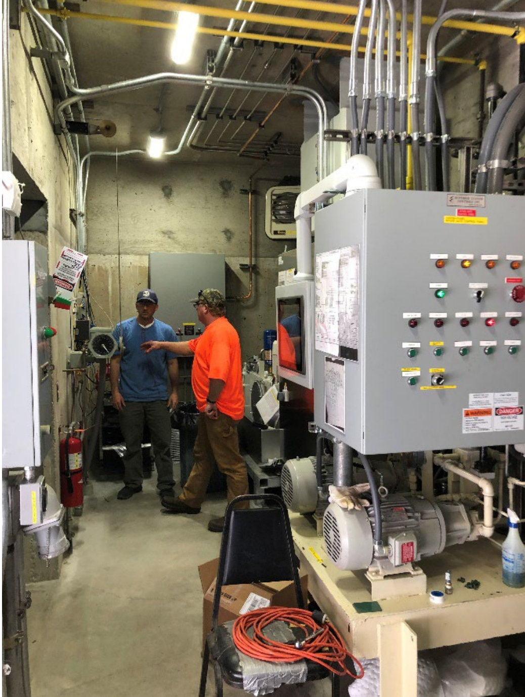
Maintenance Activities, Swan Lake Intake Building
