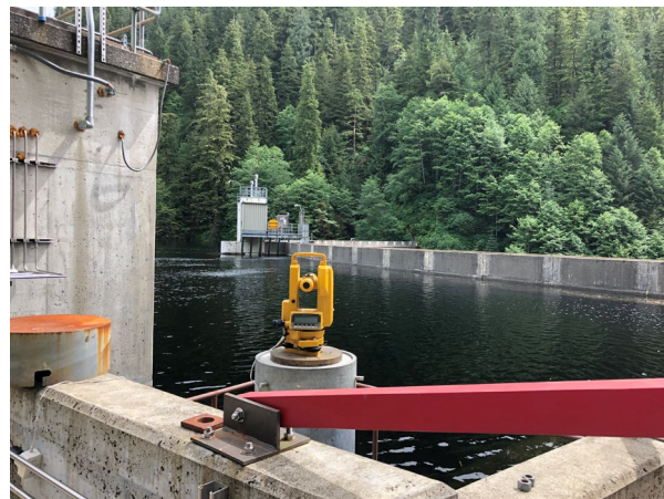
Surveying Dam Deflection 343.0'
