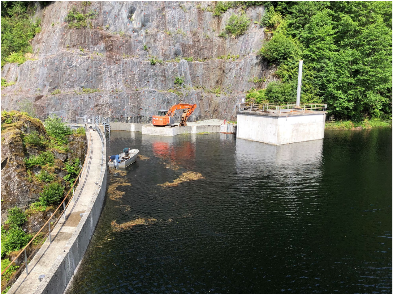
Swan Lake Intake Structure 2021
