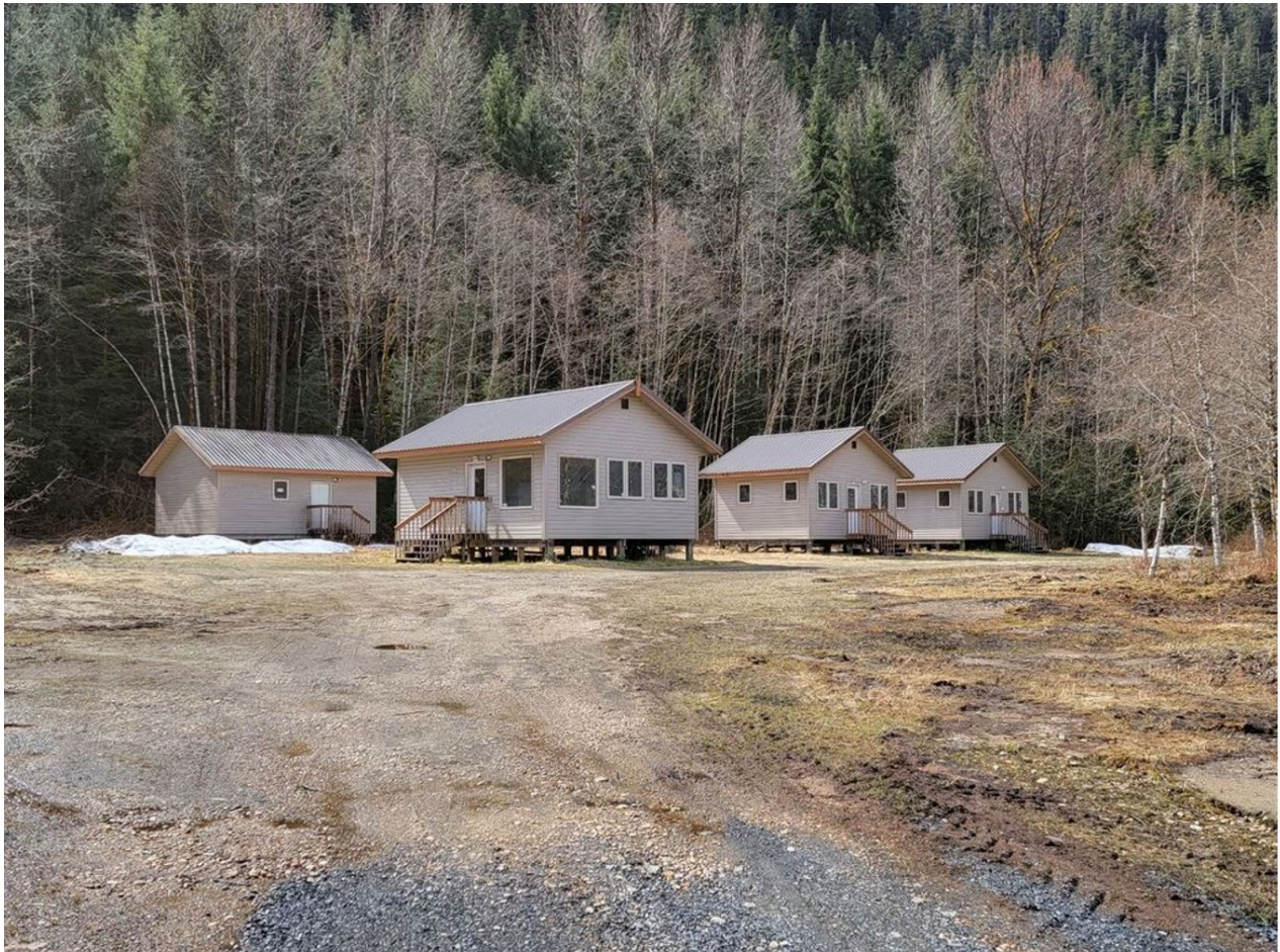
USFS Administrative Cabins at Tye
