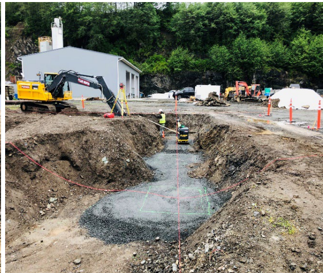
Foundation Bedding Compaction
