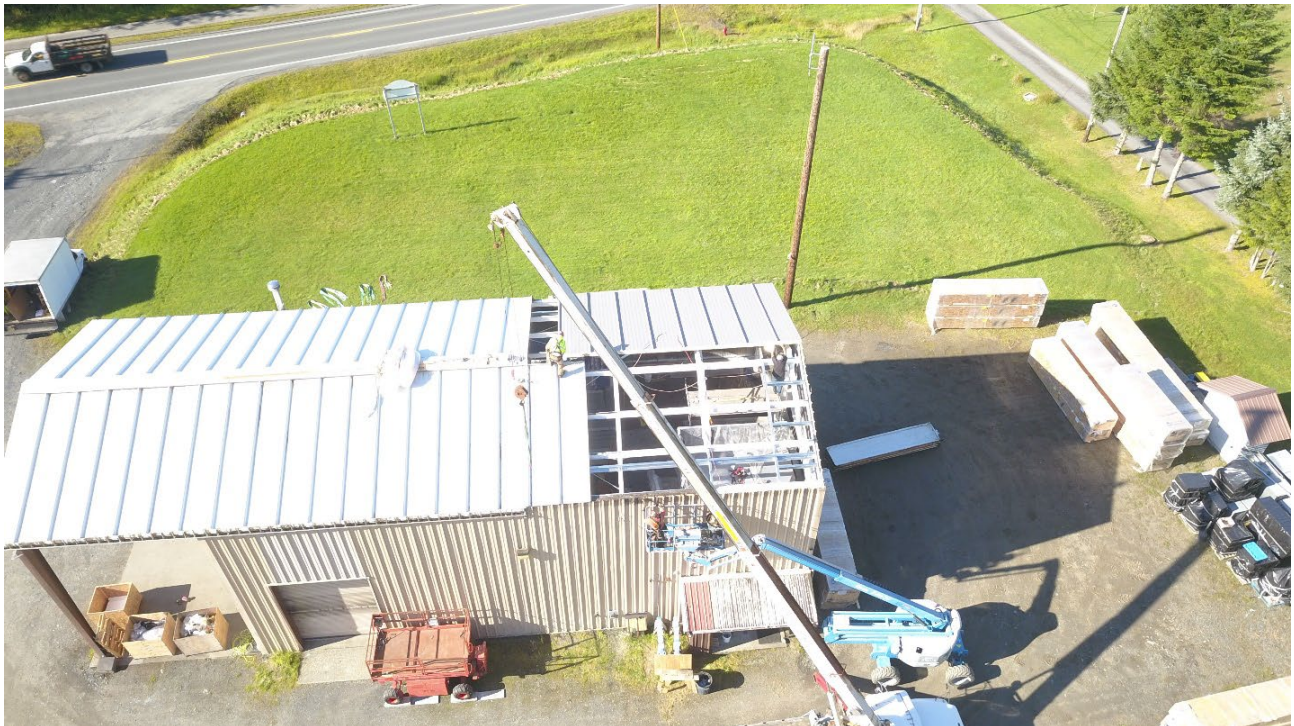
New panels secured on northwest end of building; northeast section panels being removed
