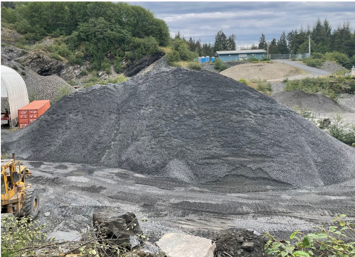
Stockpile of approximately 50% of crushed resurfacing material for Tyee Airstrip
