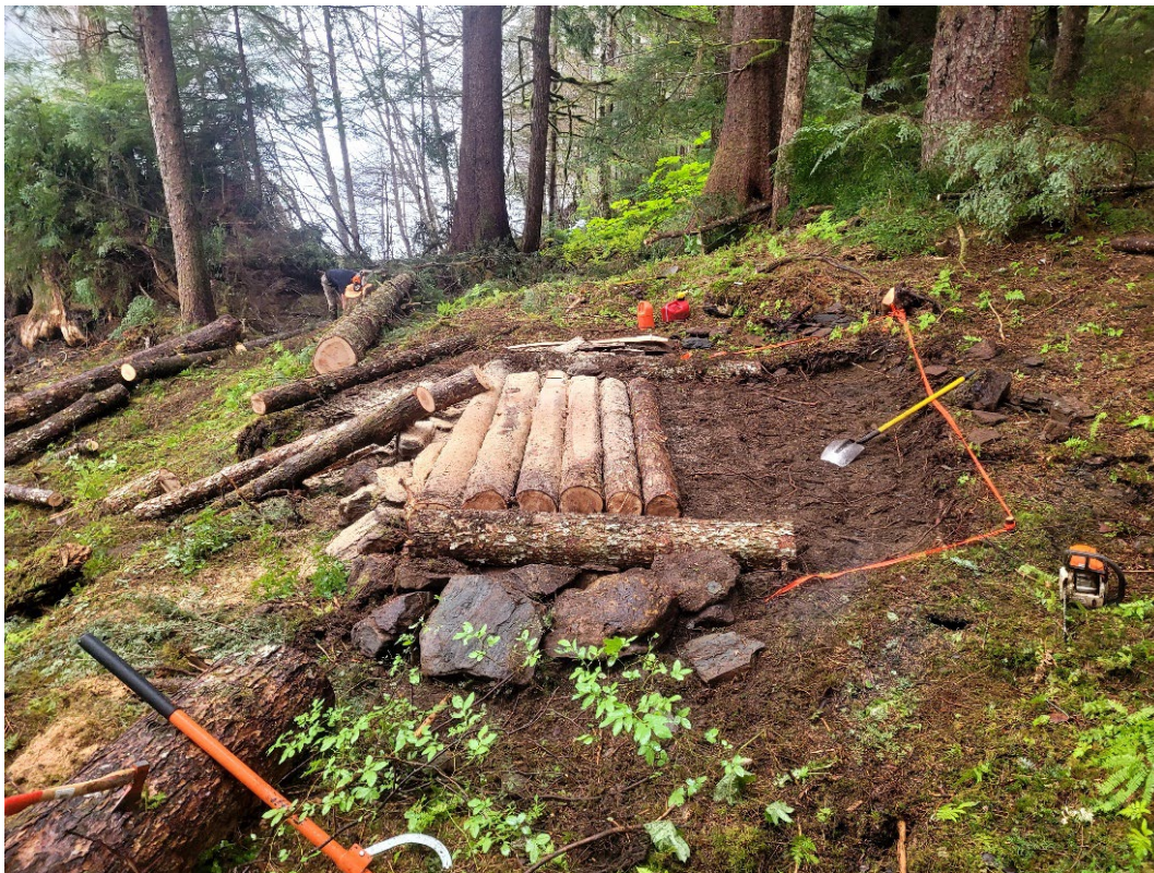
Winch Anchoring Platform under Construction
