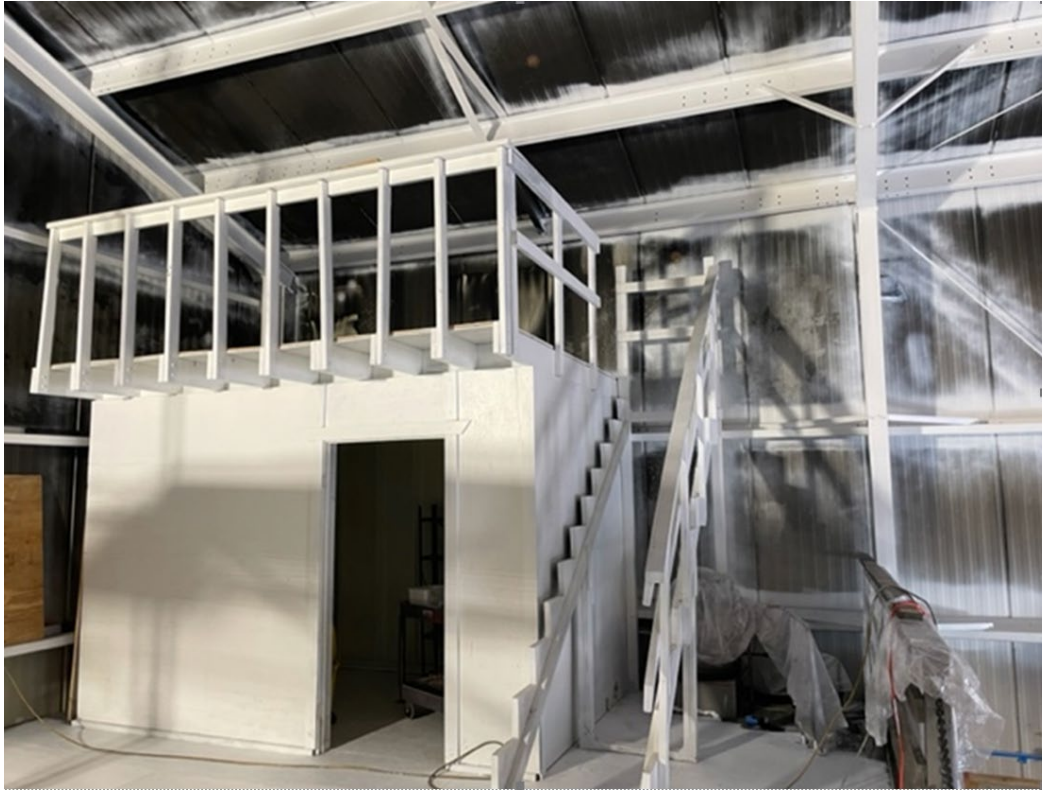
Stair treads were removed in order to clean risers, and replace the smoke damaged treads with new treads.
