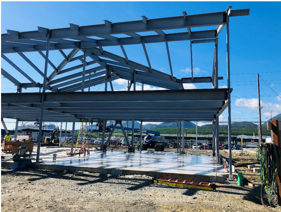
Ground Floor Poured and Superstructure Assembly
