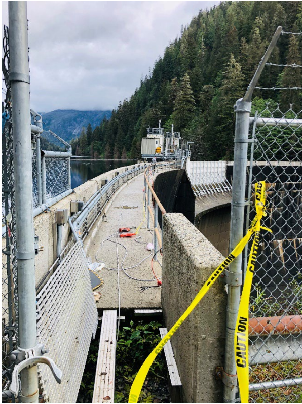
Geophone Installation on Top of Dam
