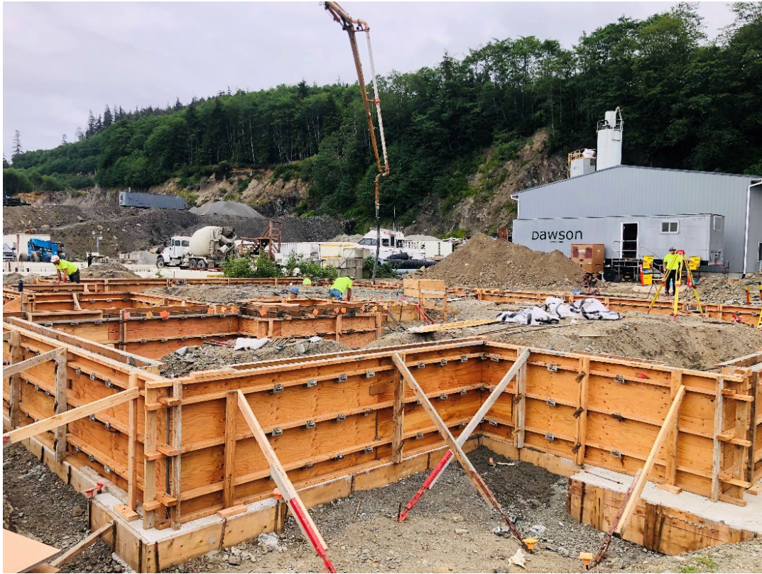
Concrete Placement Foundation Stem Walls
