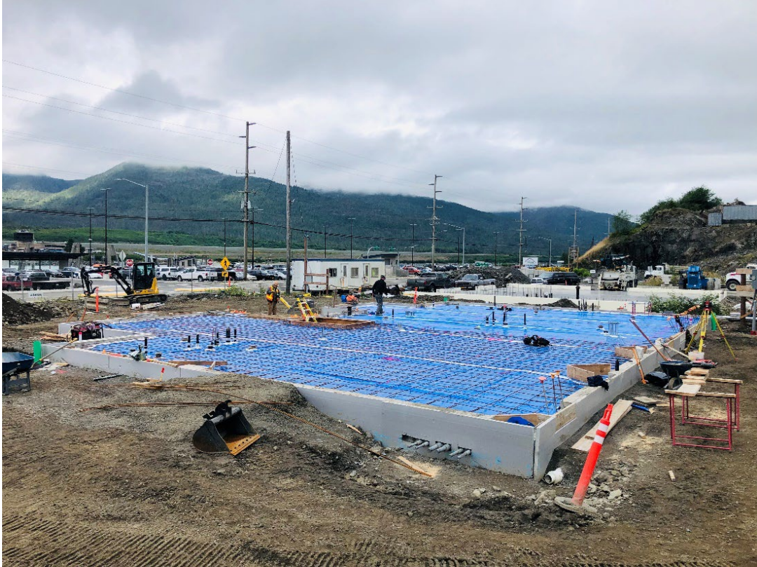
Placement of Concrete Reinforcement Steel for Ground Floor Concrete
