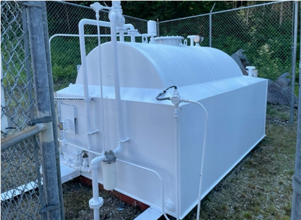
One of two freshly pressure- washed and painted fuel supply tanks.
