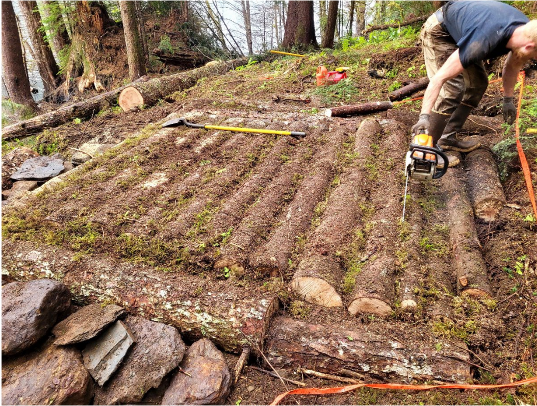
Winch Anchoring platform Complete
