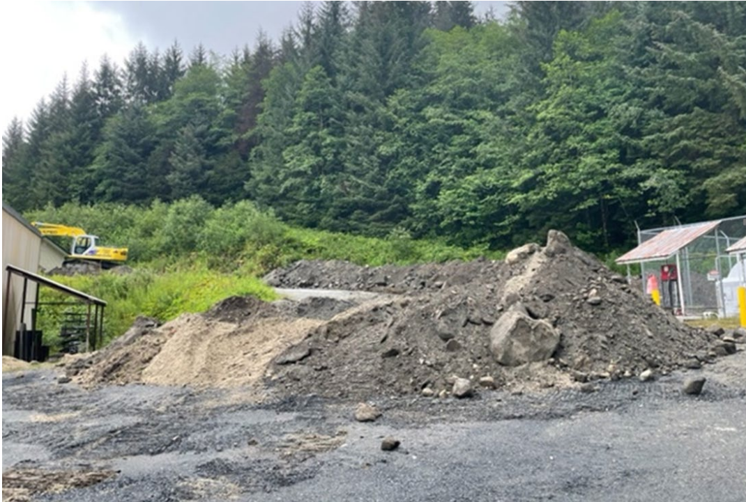
Excavated material was removed to locate the leak and lay new line. Note the size of the bedding material used in original installation.
