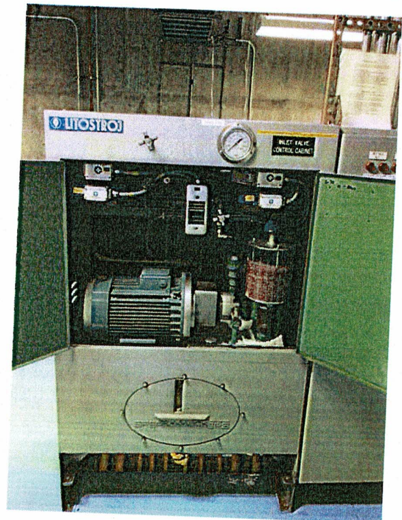
Inlet Valve Hydraulic Power Unit
