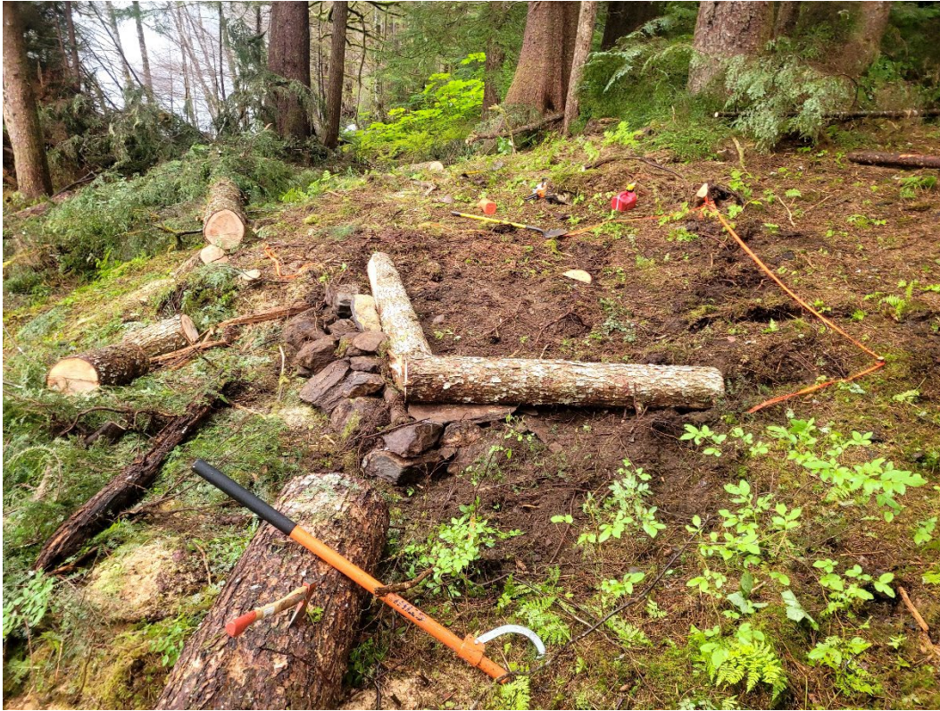
Establishing a Winch Anchoring Platform
