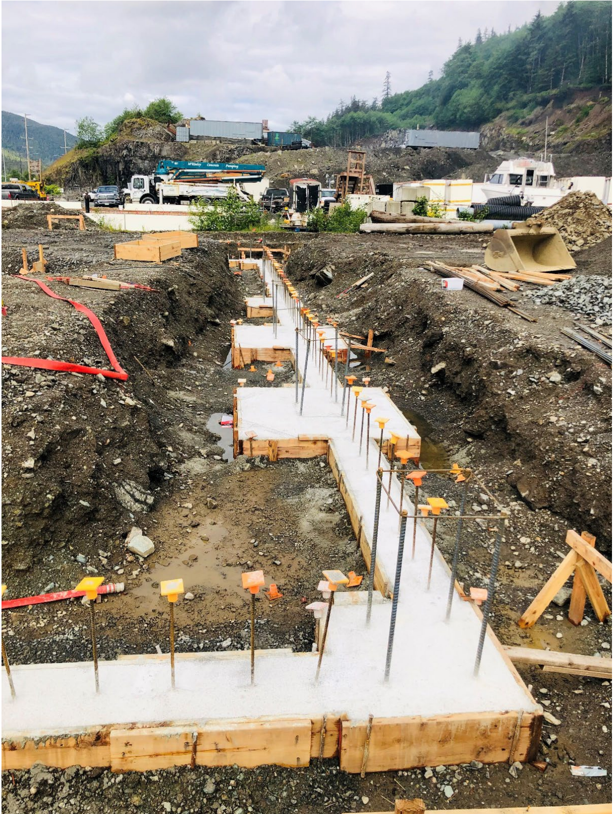
Super Structure Column and Stem Wall Footer
