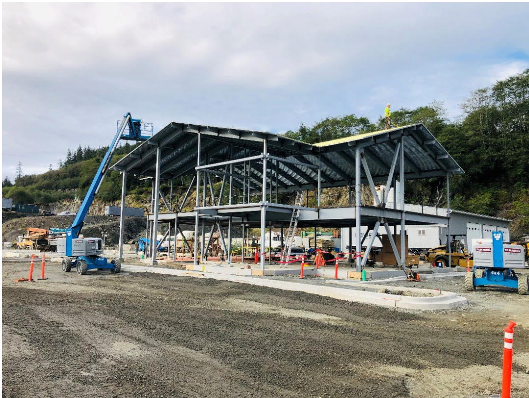
Second Floor and Roof Pan Decking Installed
