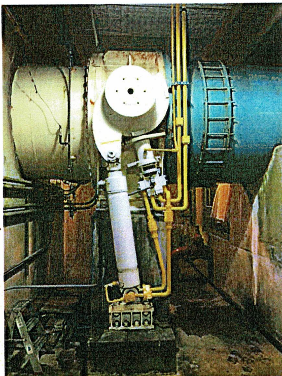
Inlet Valve Hydraulic Cylinder & Locking Pin
