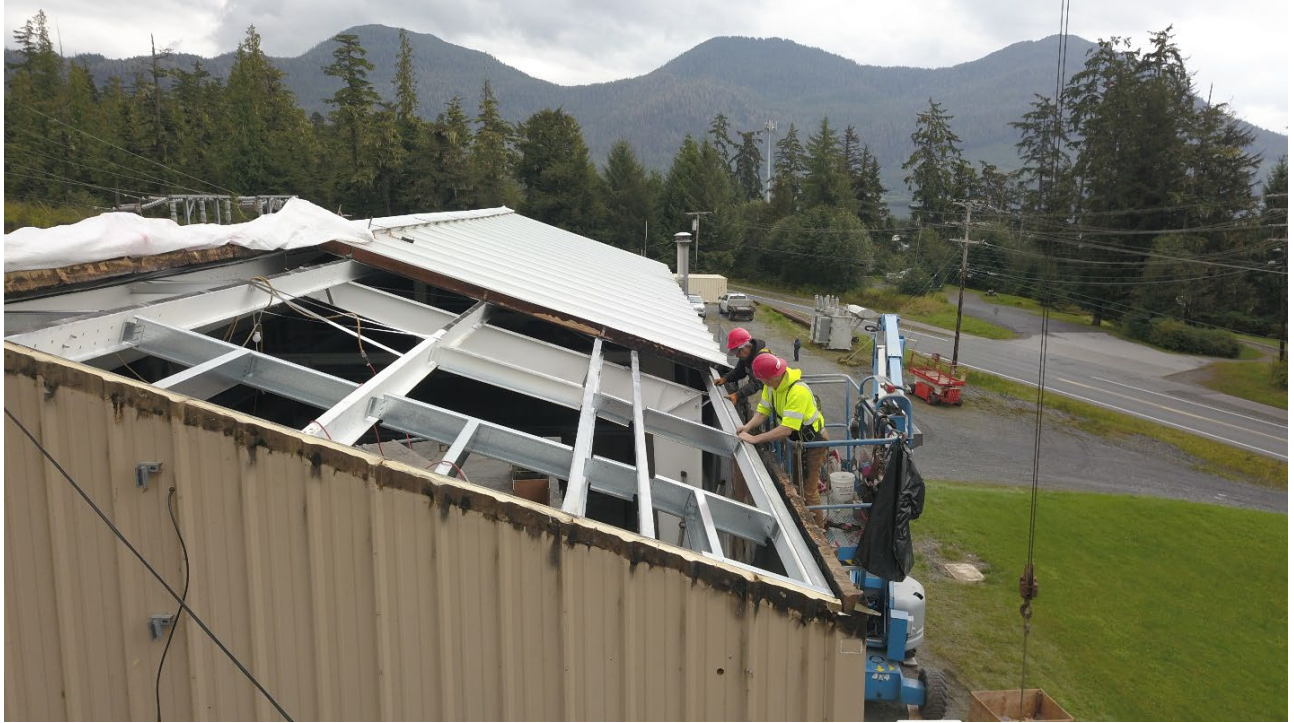
Marble Contruction crew installing new purlins prior to panel placement
