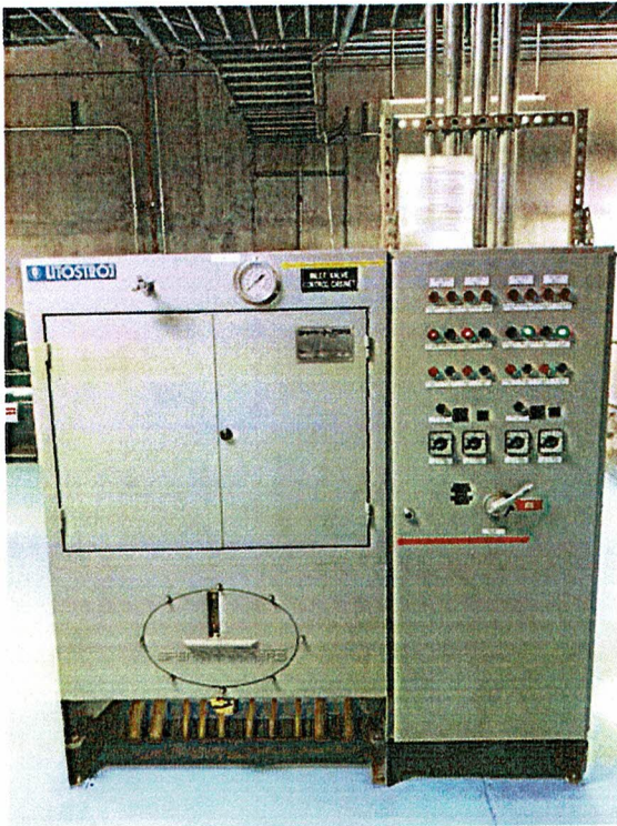
Inlet Valve Hydraulic Power Unit
