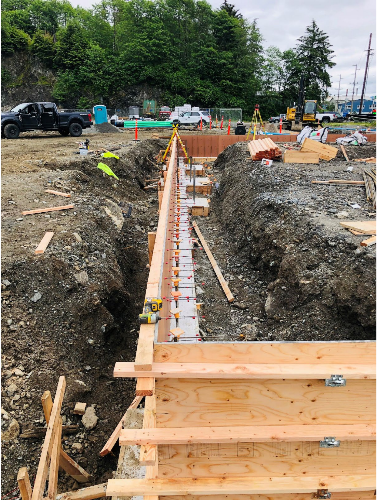
Foundation Stem Wall Forms
