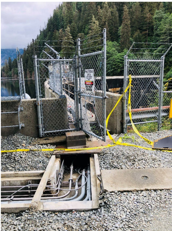
Geophone Coaxial Dam Installation
