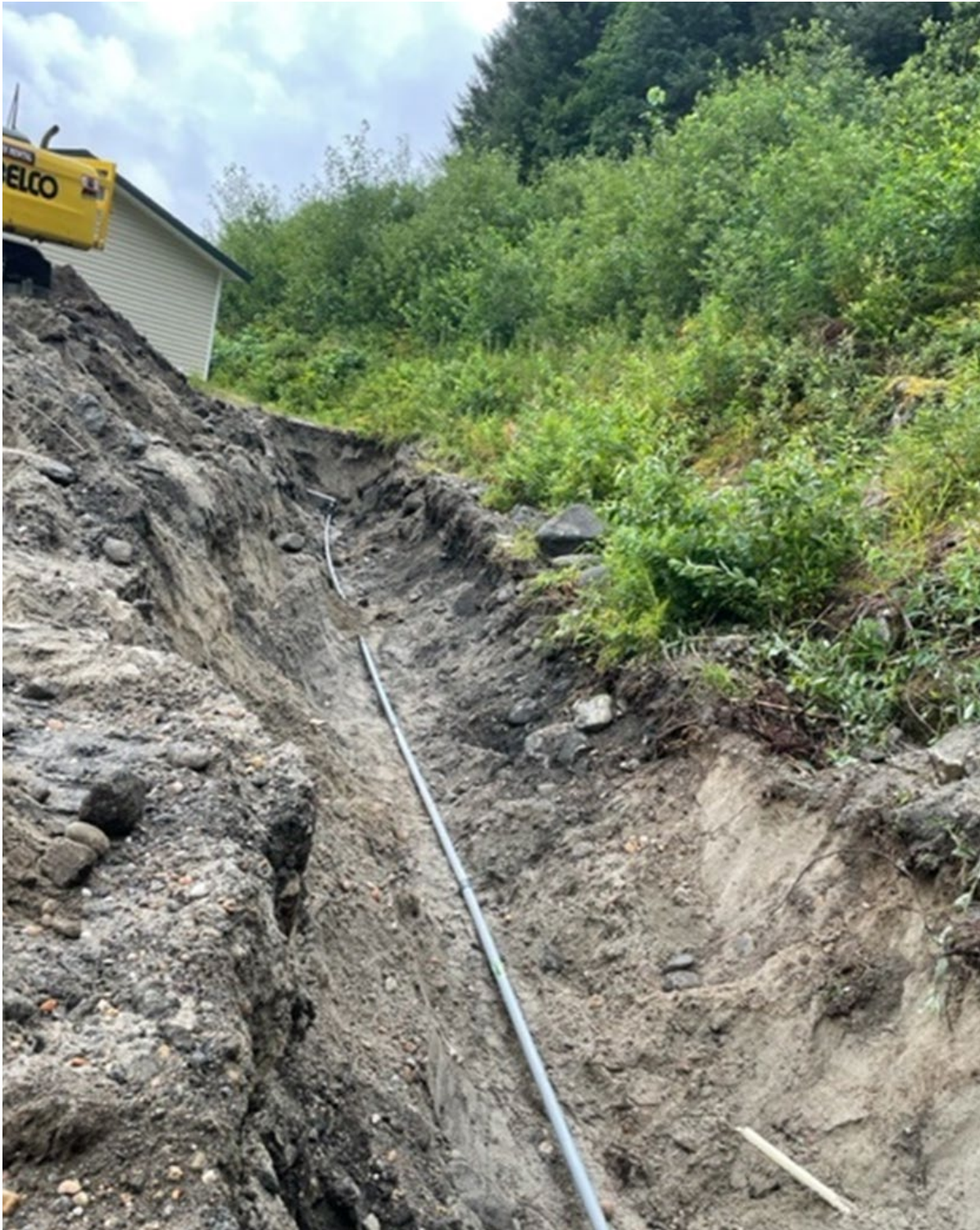
New 2" water main with isolation valve at the end of the ditch line
