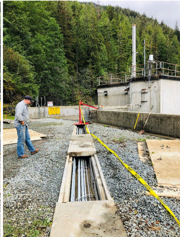
Geophone Coaxial Intake Installation
