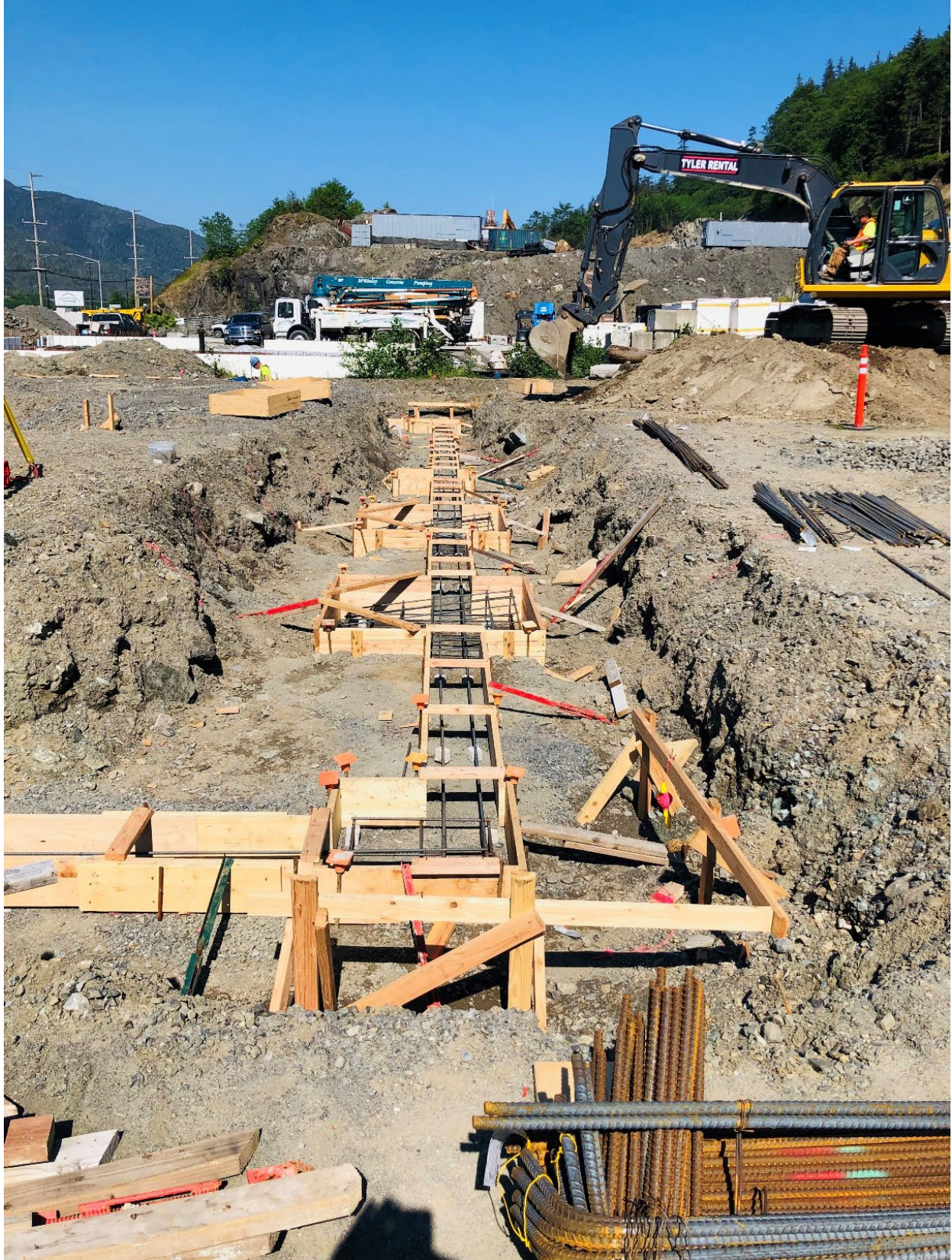
Super Structure Column Foundation and Stem Wall Footer Concrete Forms
