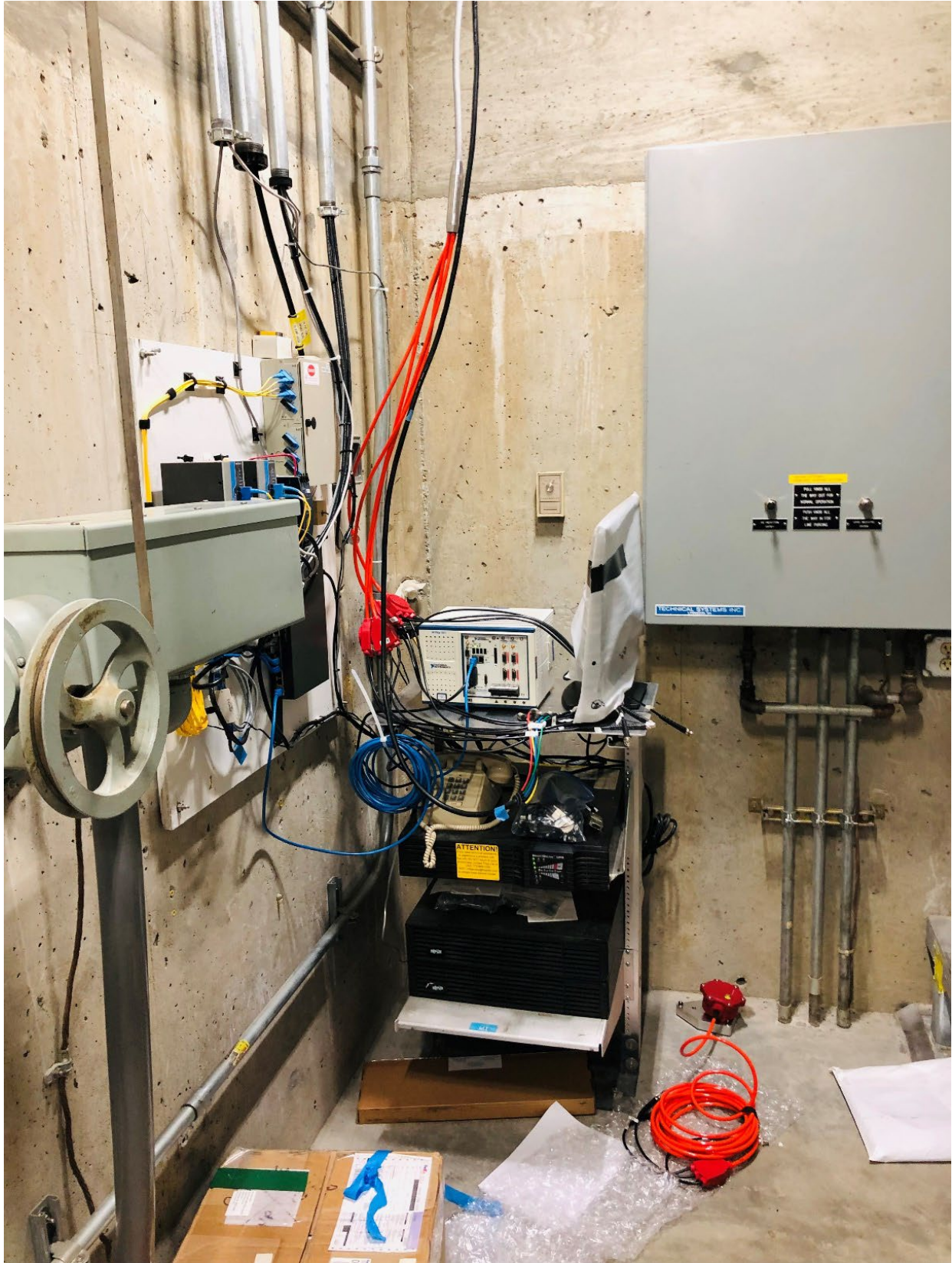
Vibration Geophone Monitoring Computer Installation at Intake Structure
