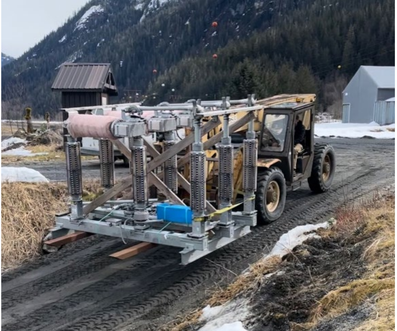
New Tye Circuit Switchers Offloaded at Tye Lake
