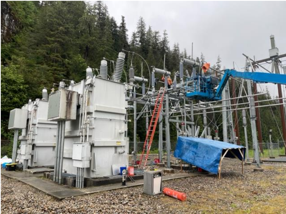
Typee Circuit Switcher Replacement work
