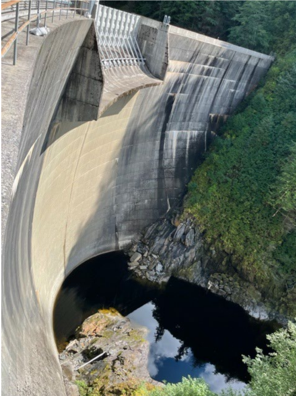
Swan Lake Dam and Plunge Pool
