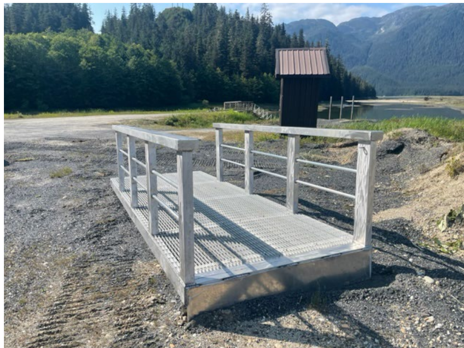
Newly built dock pier to replace aging wood structure at Tyee
