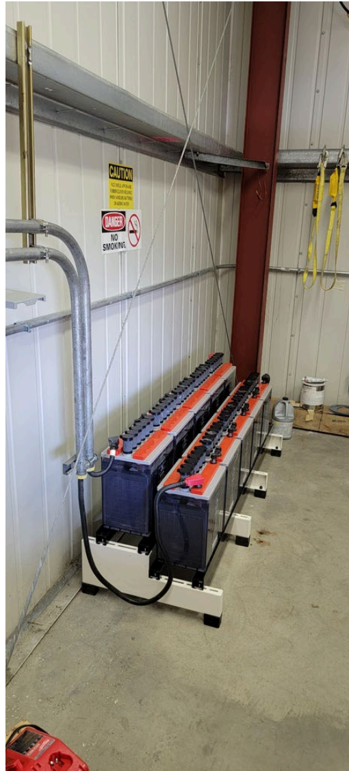
New Yard Lighting and Battery Bank at Petersburg Substation
