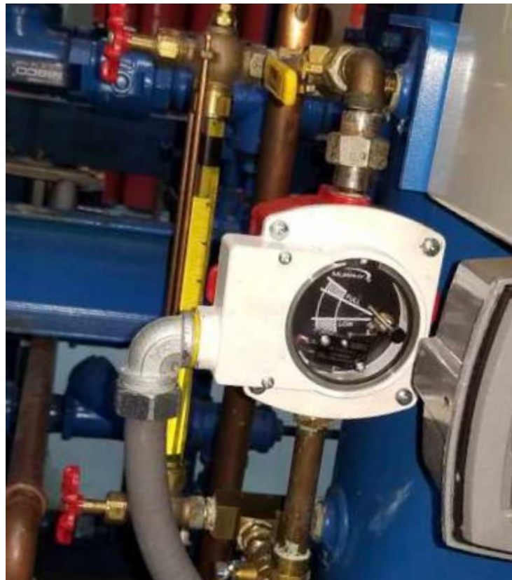
New Murphy Switch installed Swan Unit S-1 Bearing Cooler Glycol Level
