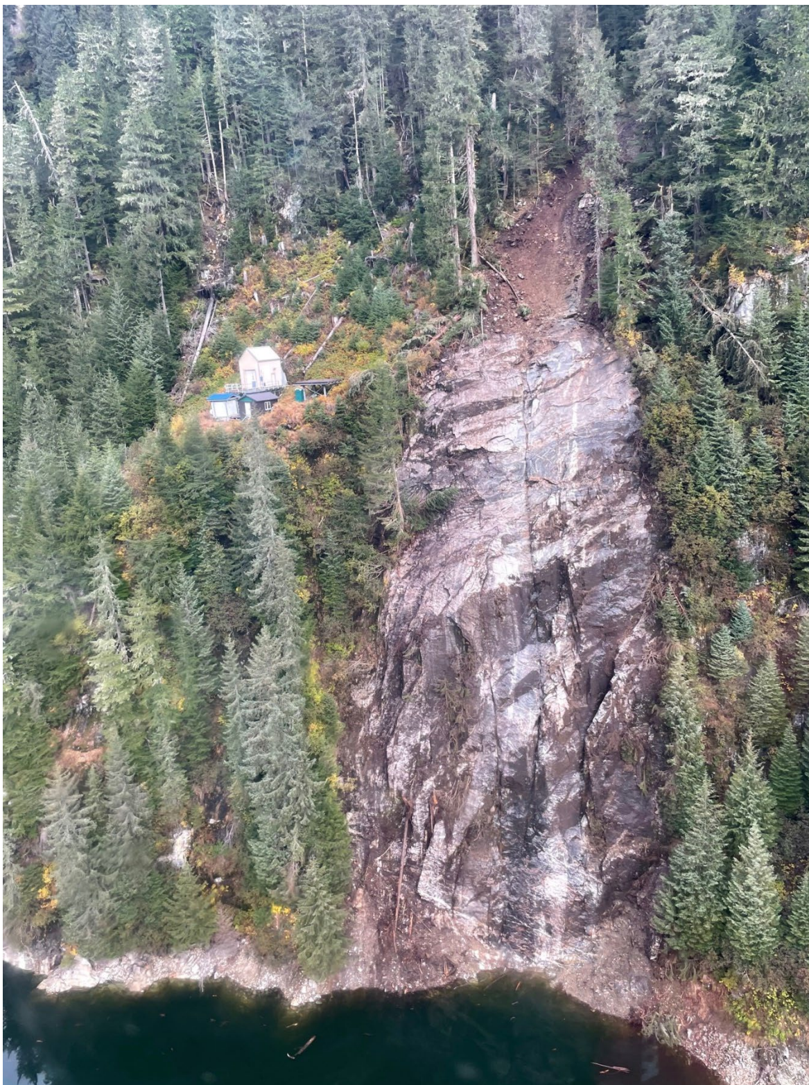
New Land Slide Adjacent to Tye Gate House
