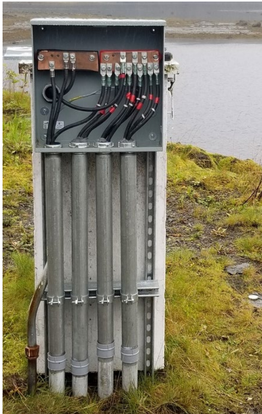
Newly Installed Swan Cathodic Protection Junction Box and Conduit
