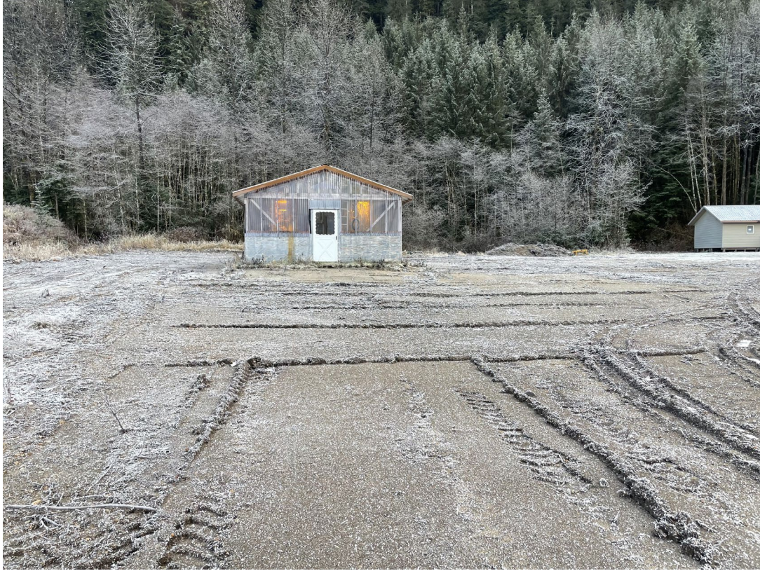
Tyee Green House with old fencing removed and ground cleared
