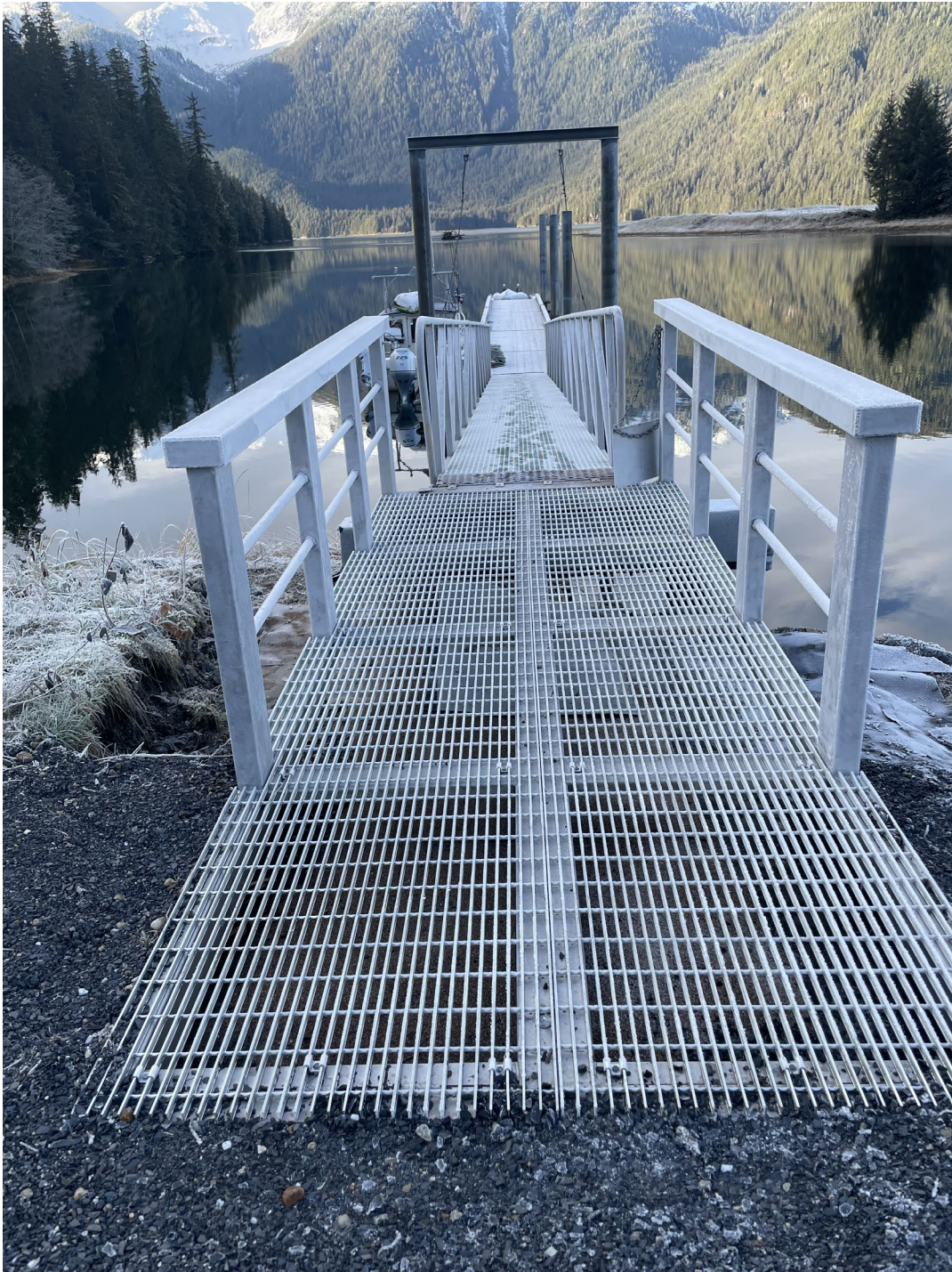
New Tye Dock Pier and Walk Ramp with New Fiberglass Decking
