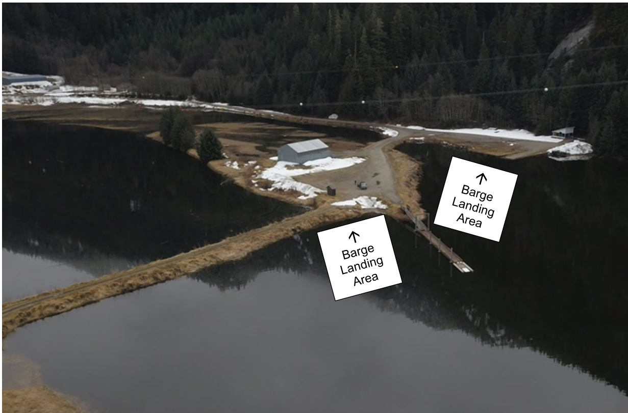
Photo of Barge Landing Areas (Note: Access by Barge is dependent upon tides.)
