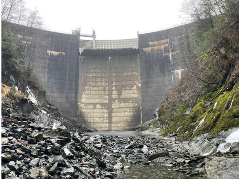
Diversion Tunnel Entrance and Diversion Plug downstream of Swan Dam:
