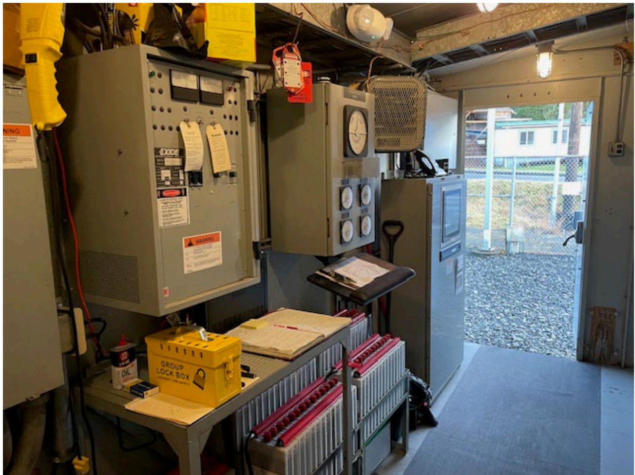
Wrangell Substation Battery Bank and Charger
