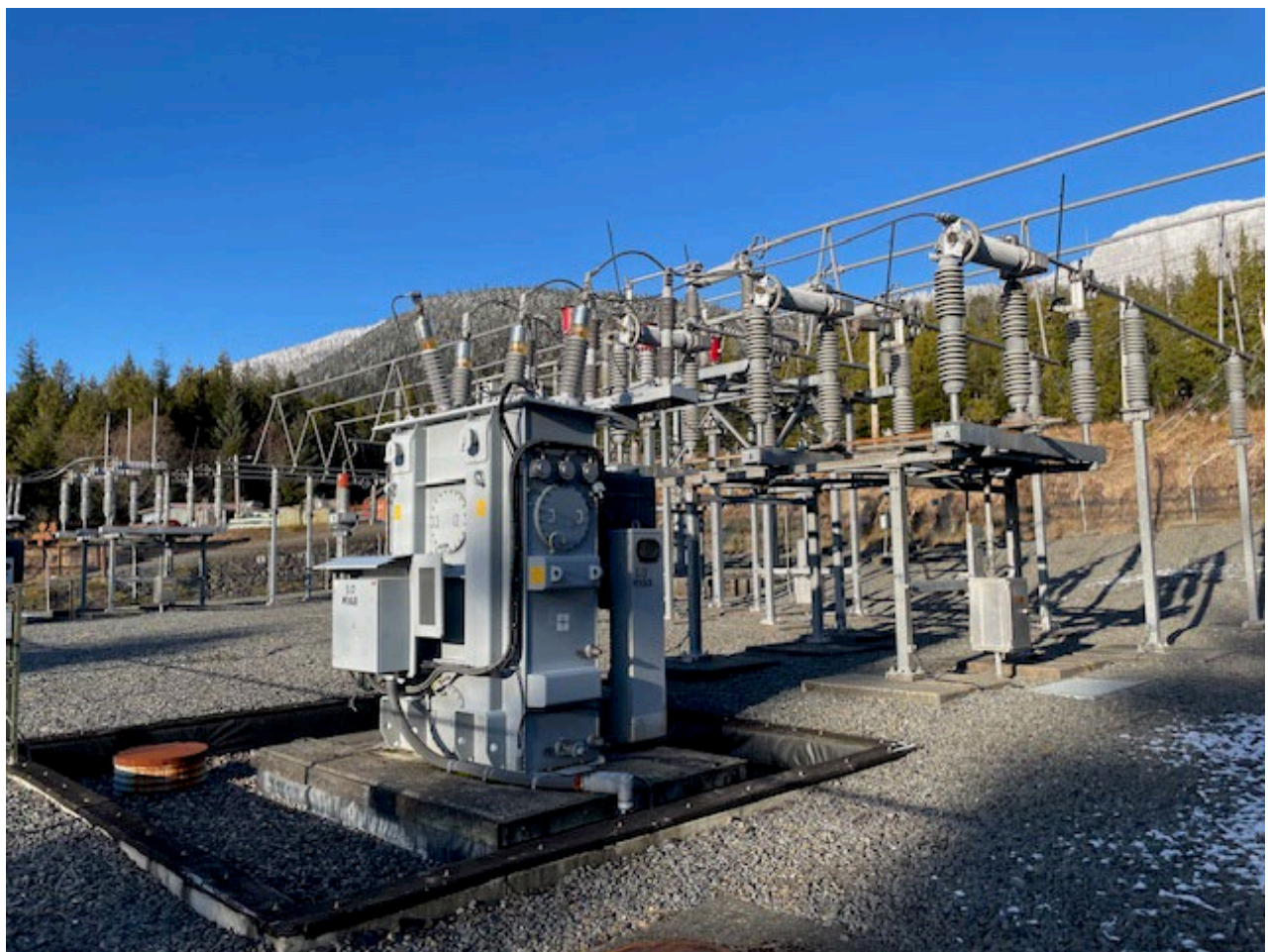
Wrangell Switchyard 5 Mvar Reactor and attached Circuit Switcher
