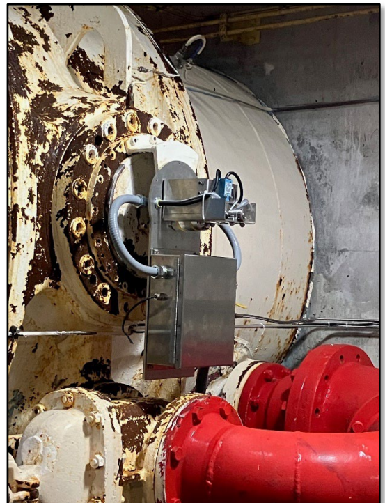
New Position Indicators Installed
