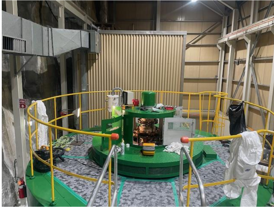
Tyee Single Unit outage Work: Brush Change and Winding Megger Testing
