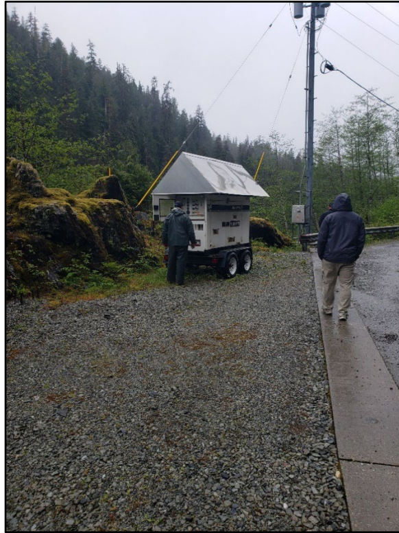
Emergency Power Operating Fixed Wheel Gate
