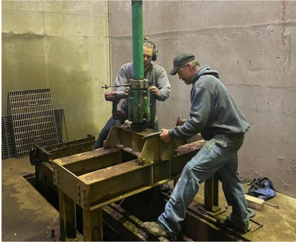
SEAPA crew preparing Swan Gate Stem for picking Penstock Gate
