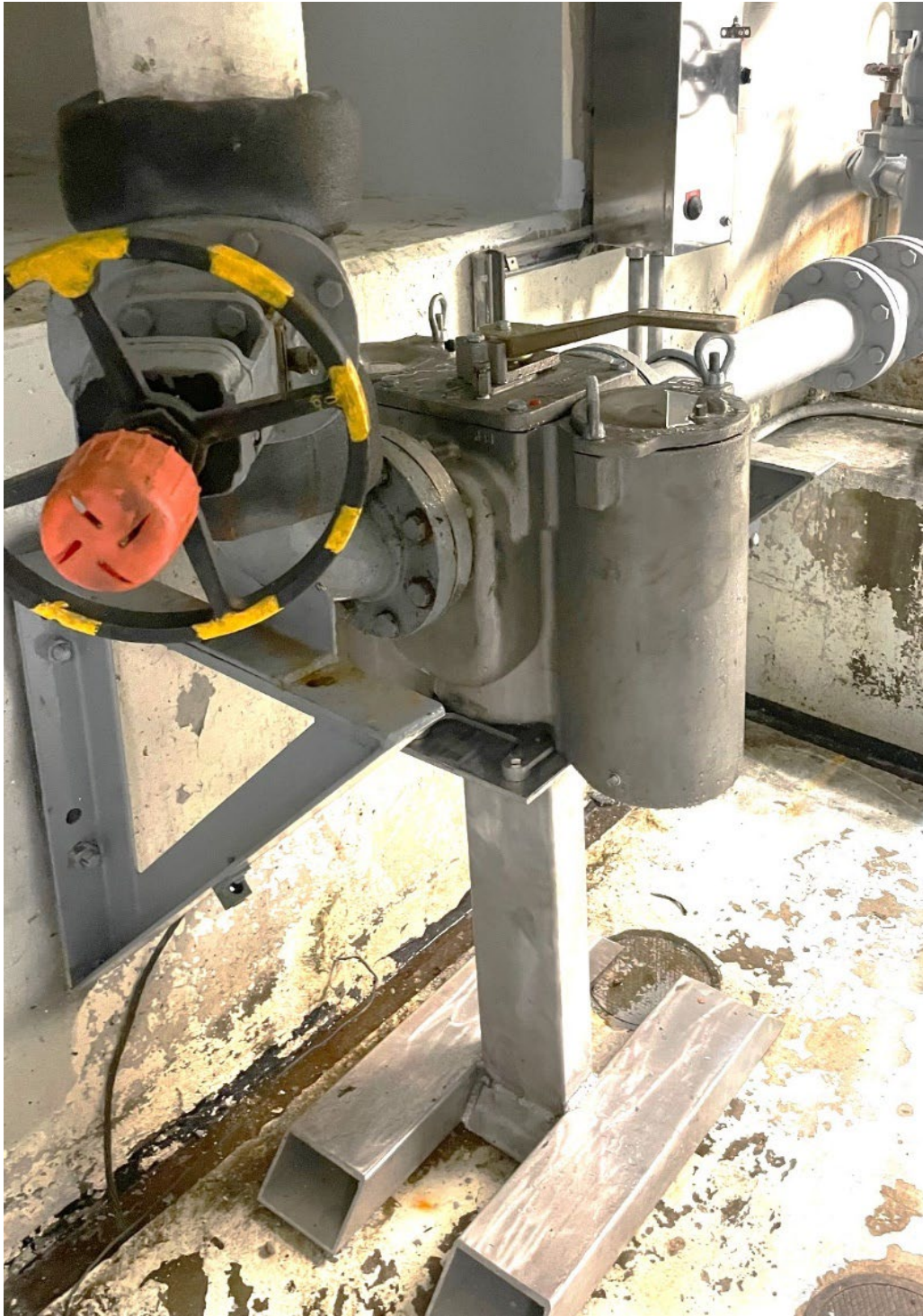
Typical installed strainer
