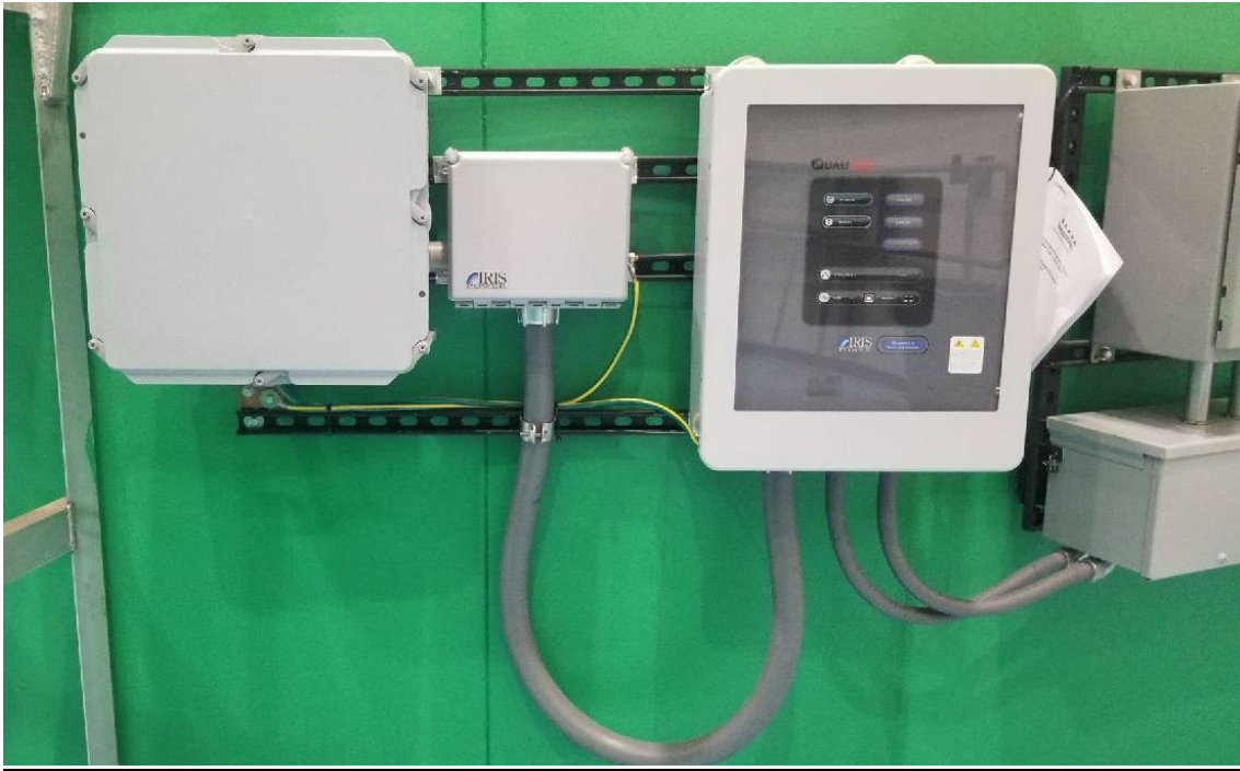
Partial Discharge Monitoring Equipment completed on outside of Unit 2
