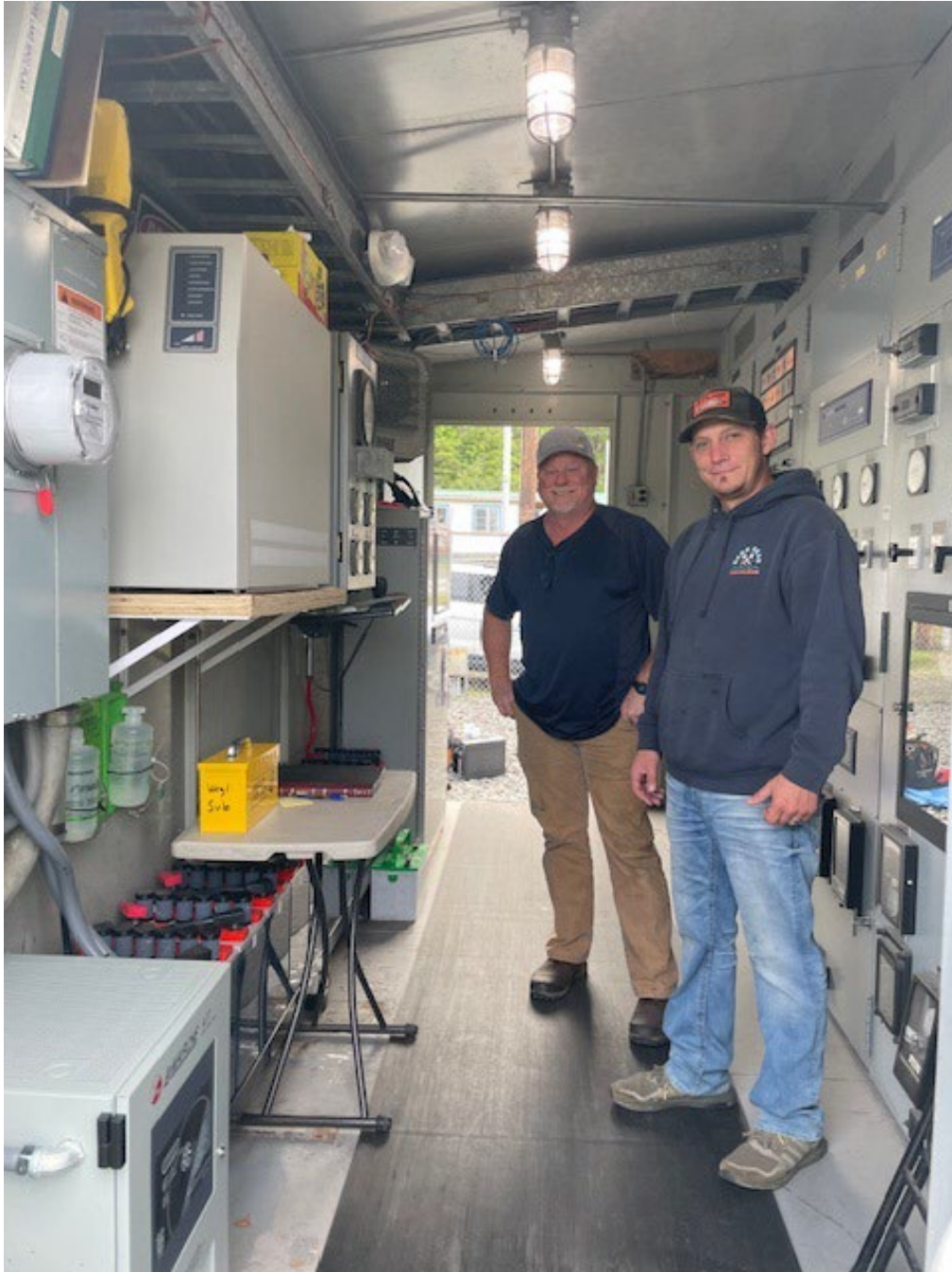
Tyee Electricians Nathan Stewart and Ashley Goyne with new Batteries, Charger and Inverter at Wrangell Substation (RR24392)
