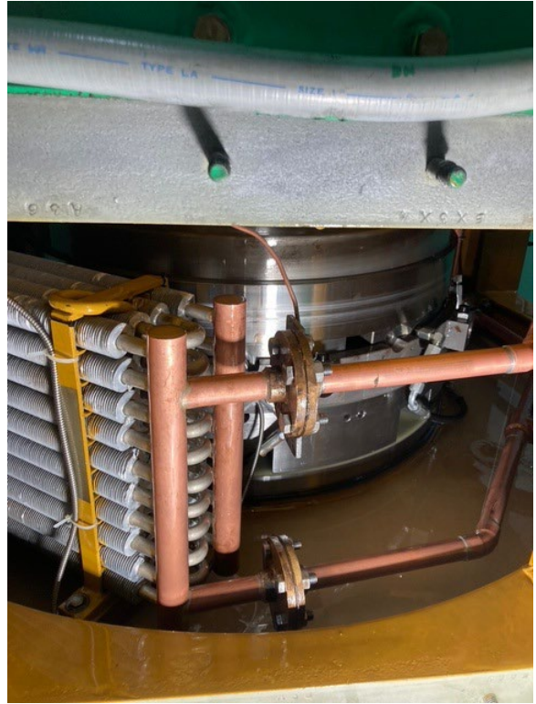
Cooling Water Leak located and repaired, Swan S-1 Generator Bearing Oil Compartment
