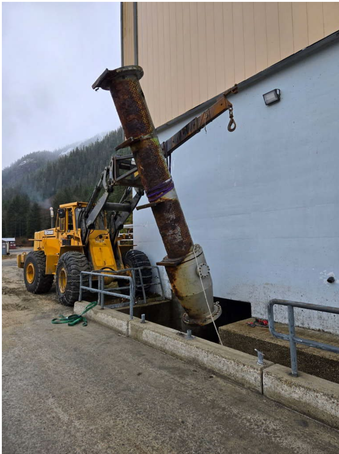
Breaking Ground on 3 rd Turbine Work Removal of Diffuser Pipe From end of Grove Valve to Accomodate Valve Function Test Equipment in 3 rd Bay
