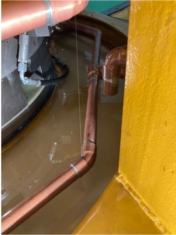
Cooling Water Leak located and repaired, Swan S-1 Generator Bearing Oil Compartment
