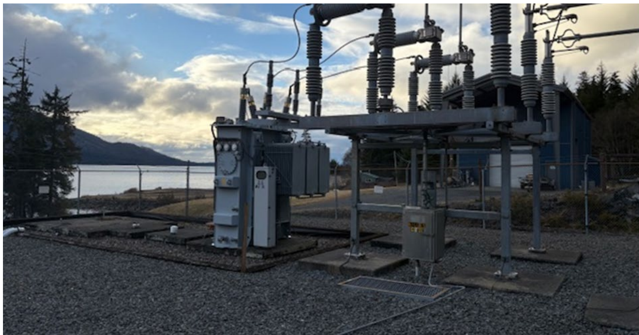
Wrangell Switchyard Reactor Circuit Switch
