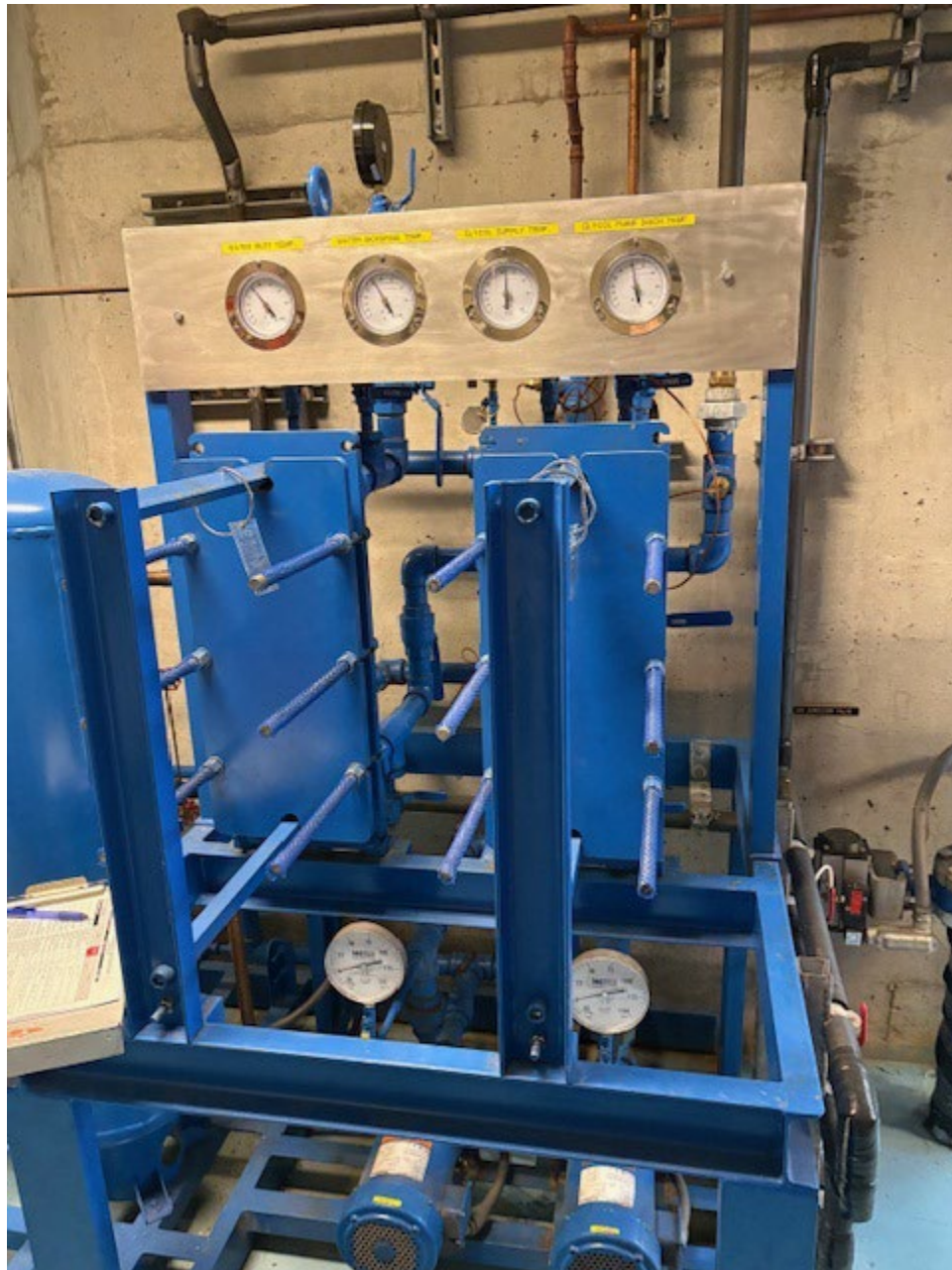
New Swan Turbine Oil Cooling Station Guage Panel
