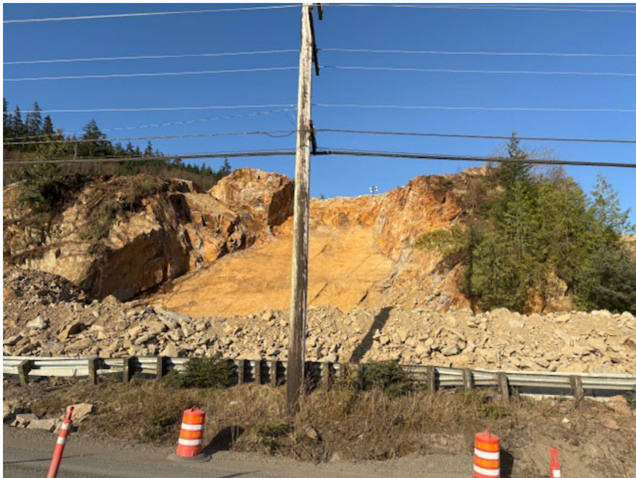
SEAPA pole inside recent Tongass Highway slide zone. Slide mitigation efforts insured no damage was done to pole structure
