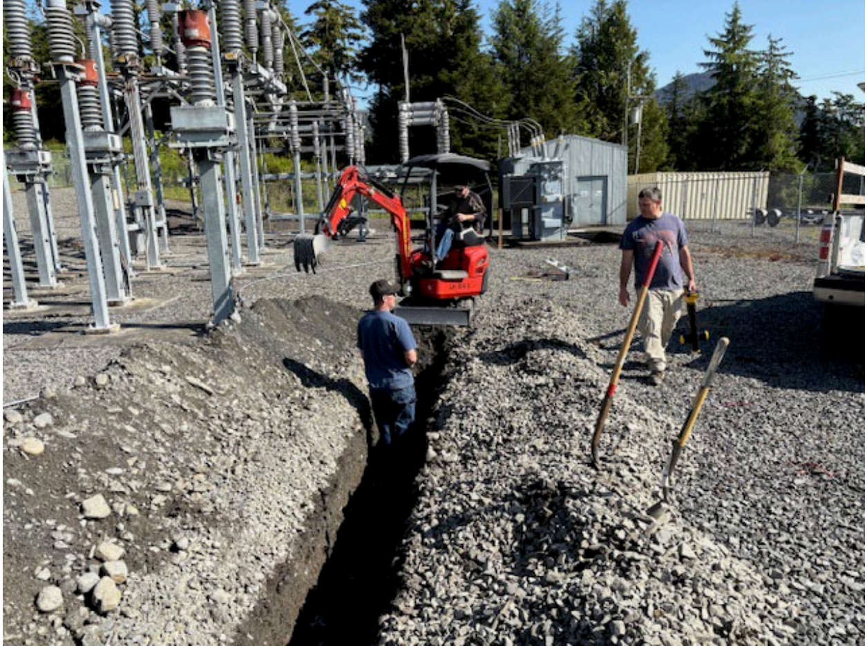
SEAPA crew, Andy Cowan and Dan Rohr, laying ditch for new conduit placement in Wrangell Switchyard. SEAPA Electrical Controls Engineer, Kris Womak, supervises to facilitate smooth operations. The yard was de-energized and crew is replacing a failed circuit switcher power supply to CST-27
