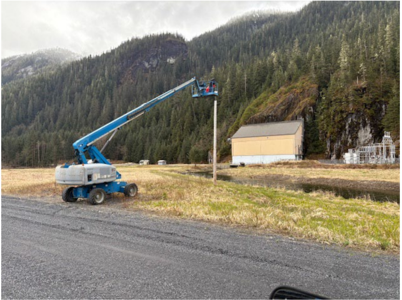
Wind Sock Replacement at Tyee Lake Airstrip. The Socks were weather-beaten and typically only last about 4-5 years
