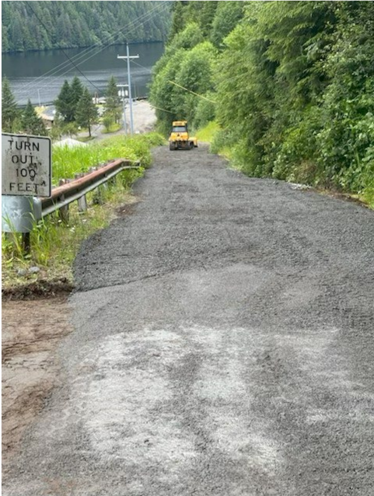
Swan Crew Spreading Gravel With Cat On Service Road Project
