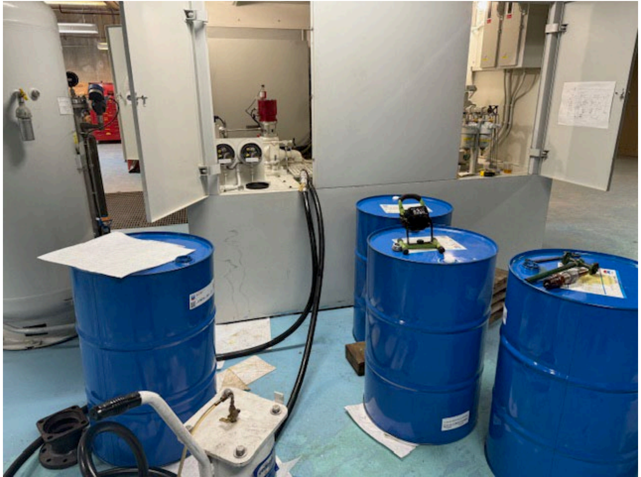
Swan Lake crew uses this portable filtering station to clean hydraulic oil in S-2 Governor Station. The ability to remove water and particulates from the oil extends the service life of the oil at great savings to SEAPA.
