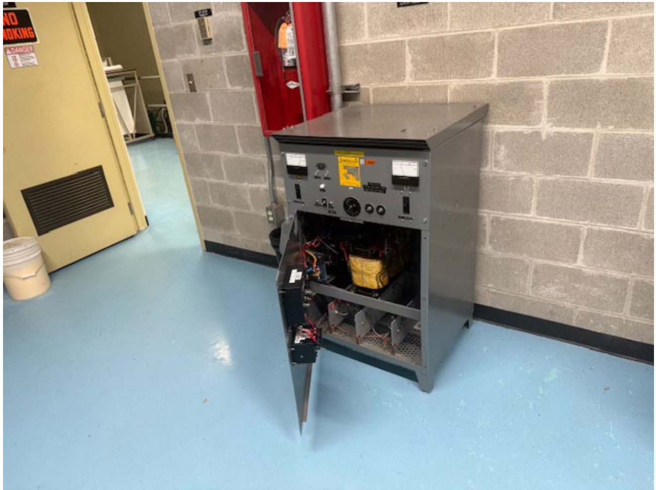
Large industrial sized battery charger used for maintaining Swan Lake main plant battery bank. One of two chargers, this one is opened up so electricians can test and validate alarm set points.
