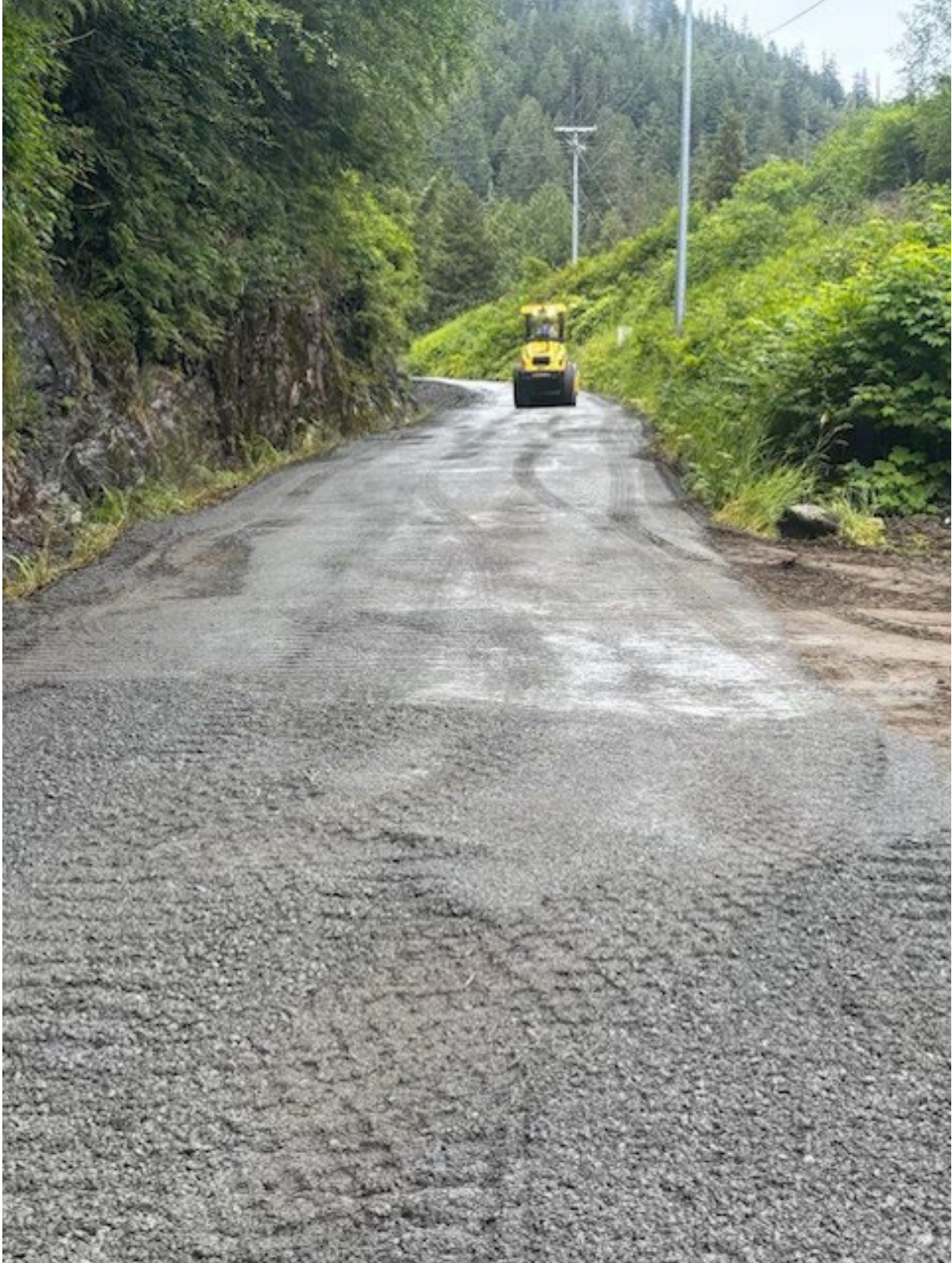
Swan Crew Compacting gravel On Road Service Project
