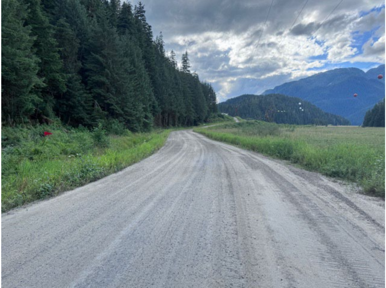
Recently graded and compacted Tyee Service Road - ready for Summer Service
