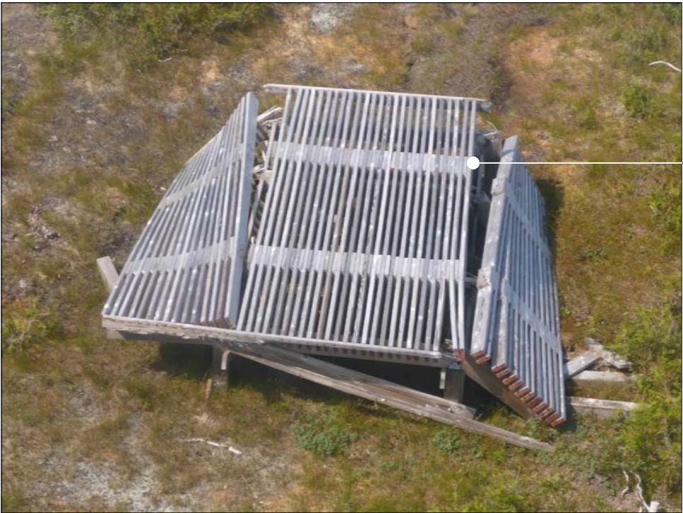
2 TYPICAL EXISTING 14x14 WOOD HELIPAD NOT TO SCALE – USE DIMENSIONS TYEE 06-02, P1110383
