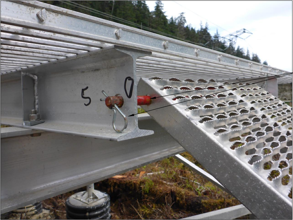
4 HELIPAD DECK ACCESS RAMP CONNECTION NOT TO SCALE - USE DIMENSIONS
