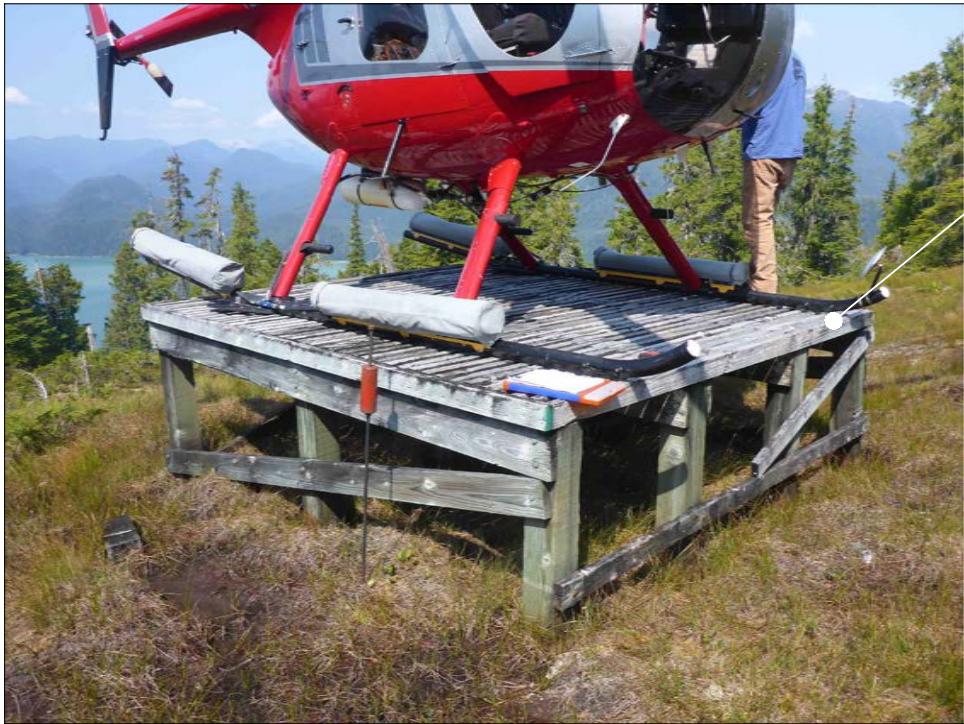
1 TYPICAL EXISTING 10x10 WOOD HELIPAD NOT TO SCALE – USE DIMENSIONS TYEE 05-01, P1110367
