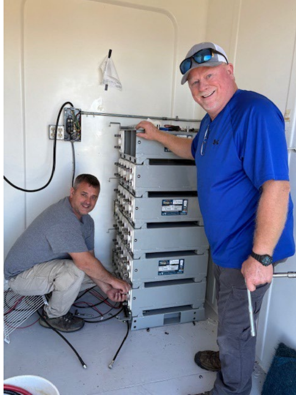
SEAPA Electrical Controls Engineer, Kris Womak, and Tye Electrician, Ashley Goyne, disassemble Battery Bank at Burnett Peak.
