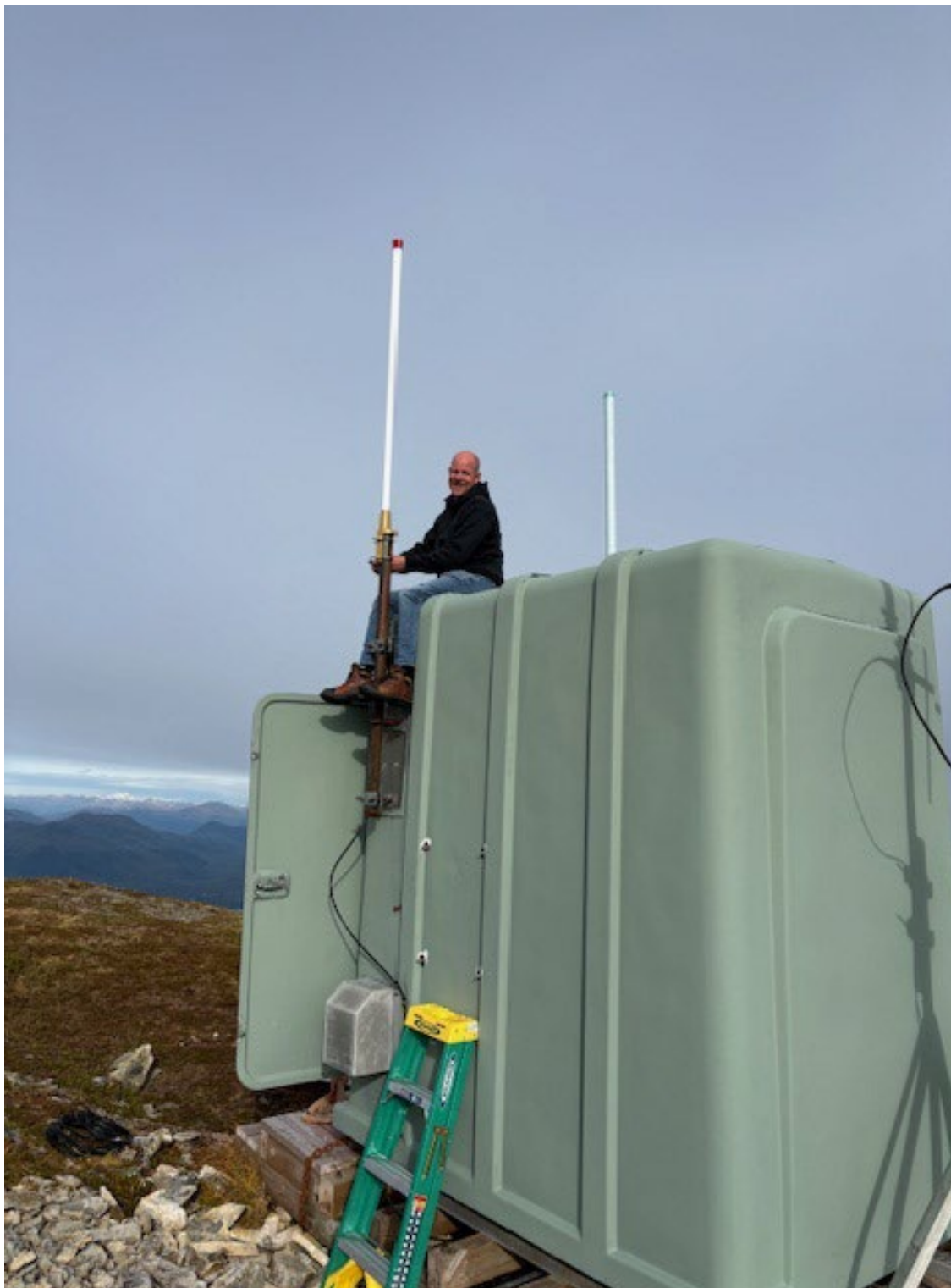
Rare photo of Robert "The Boss" Siedman getting some time out in the field! Robert is assisting with replacement of a failed marine terminal radio antenna at Burnett Peak.
