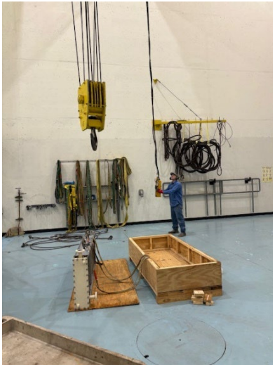
Swan electrician, John Stanley, positions the crane for removal of the old cooler
