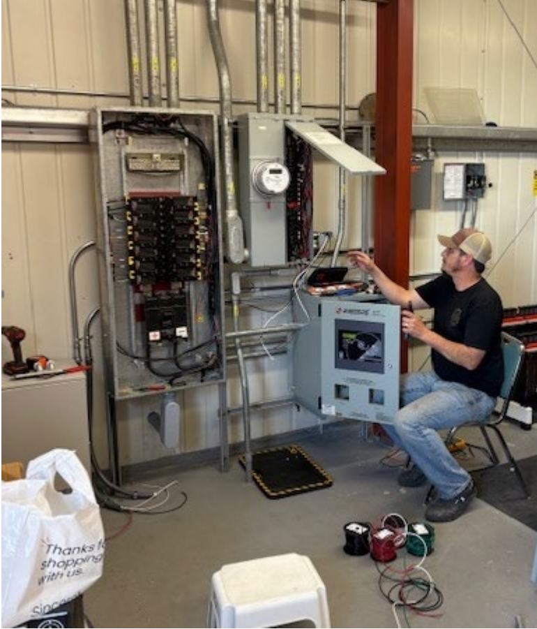
Tyee Electrician and Plant Foreman Nathan Stewart Wiring up new Batteries and Charger for Wrangell Switchyard
