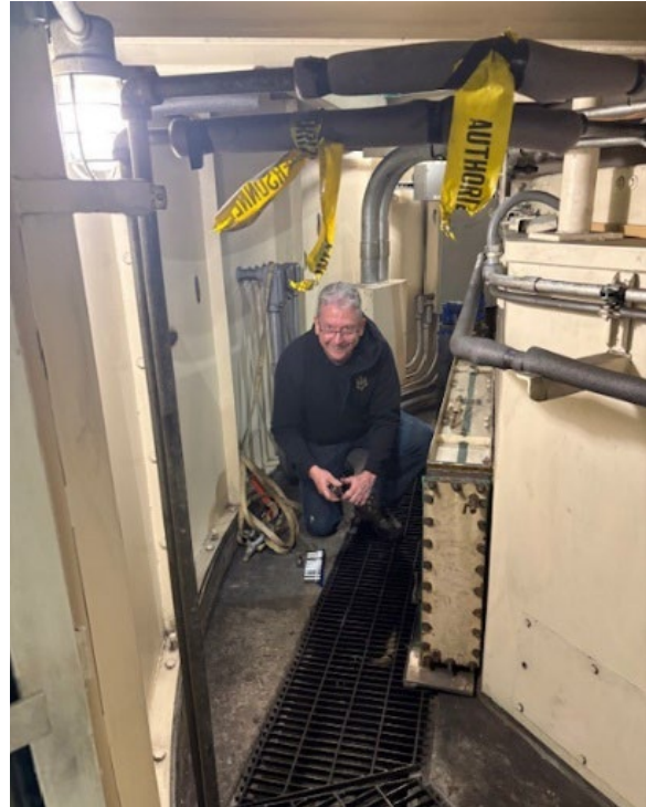
Engineer, Mark Hilson, helps with removal and prepping for the pick.
