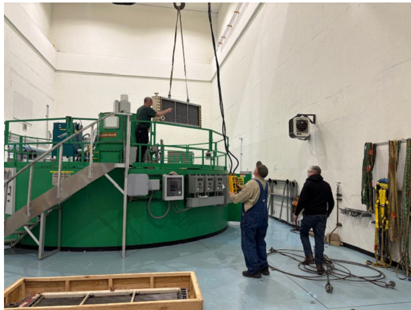
Swan Mechanic, Brett Blasingame, helps position new cooler over access hatch while Electrician, Chris Barnett, operates the Crane to lower it in place. Mark Hilson looks on to help make sure all goes smoothly.
