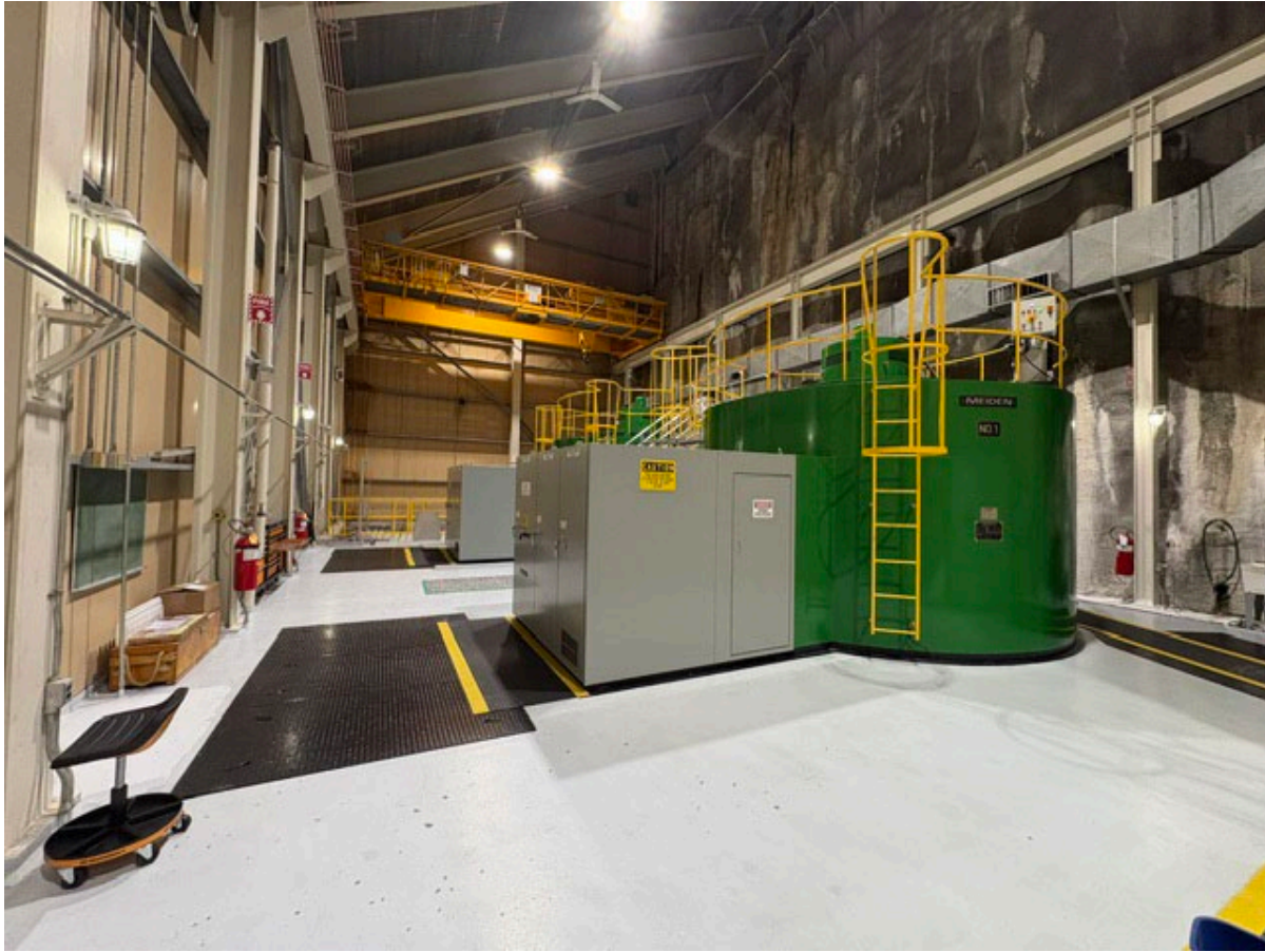
Above: Tyee Generator Deck Getting Prepped for Single Unit Outage
