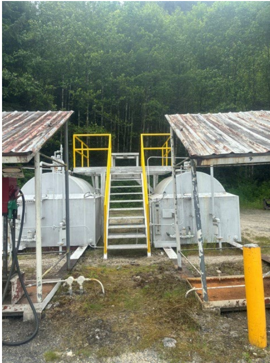
Above: New Fuel Offloading Station with Stair and Handrails At Tyee
