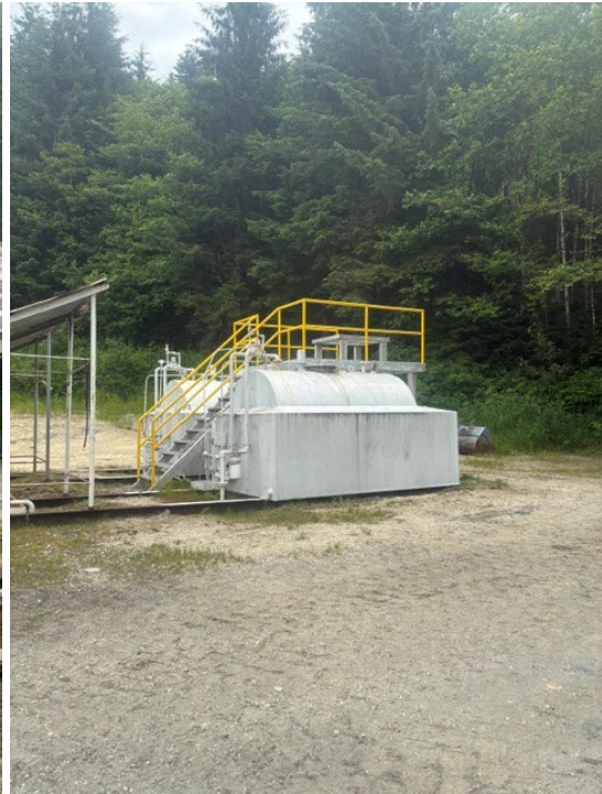
Above: New Fuel Offloading Station with Stair and Handrails At Tyee
