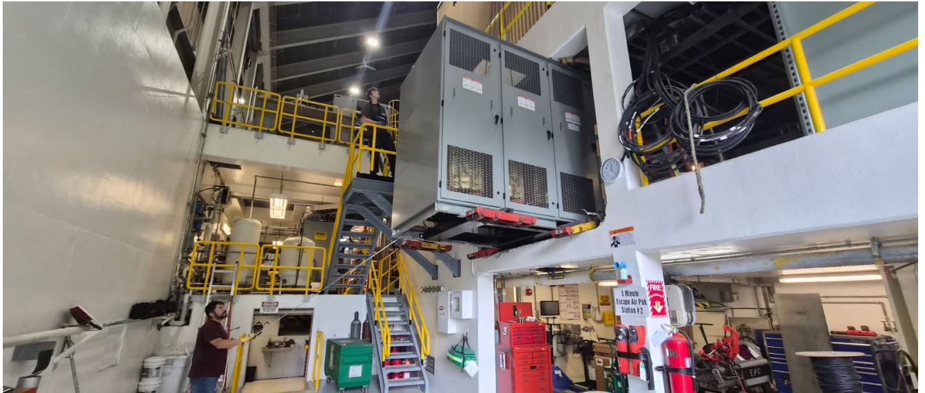
Above: Tyee Lake Station Service Gear being installed at Tyee Governor Deck Level
