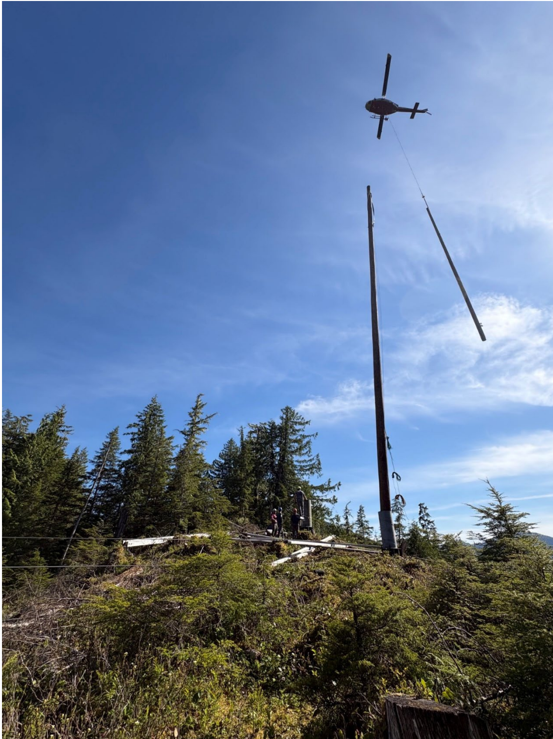
EPC Line Crew setting 85' tall pole on Tower #194 Swan/Bailey Line
