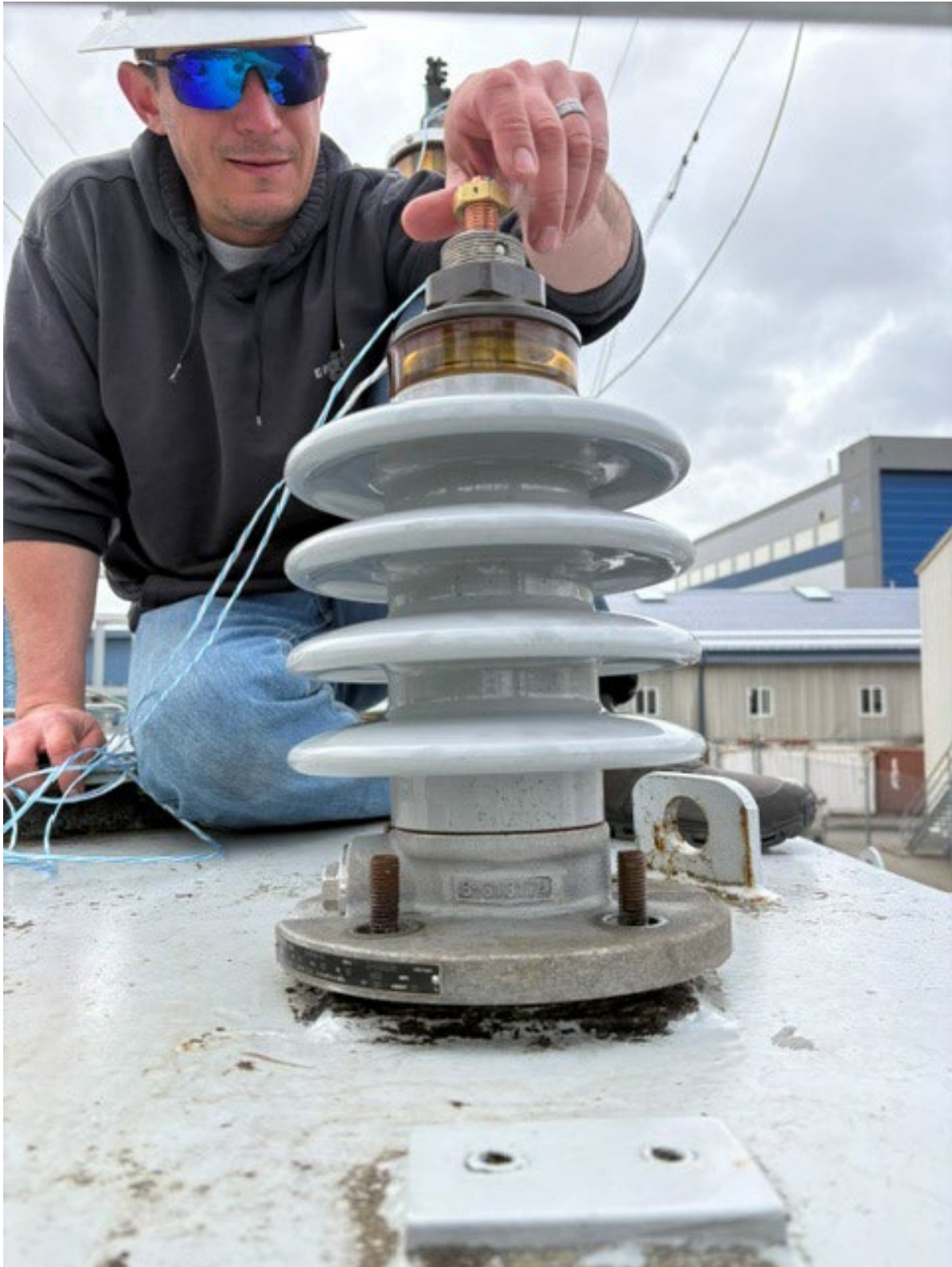
Above: SEAPA Electrician, Nathan Stewart, installing Neutral Bushing at Bailey Substation
