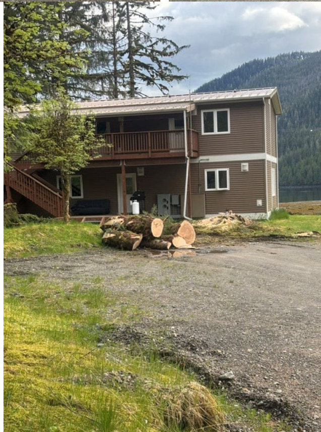
Above: Swan Lake Tree Removal from Camp area, no more clogged gutters
