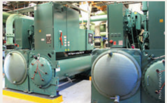
New, high efficiency chillers
