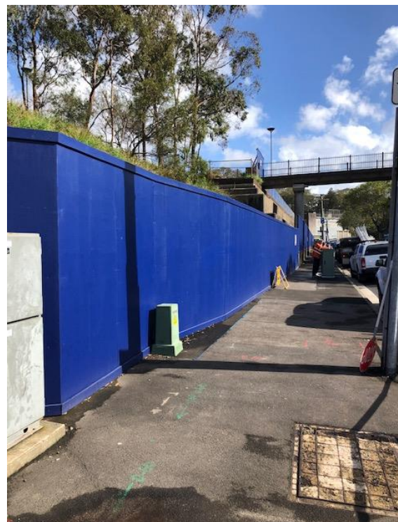
Photo 6: Perimeter hoarding along the Lincoln Crescent site boundary
