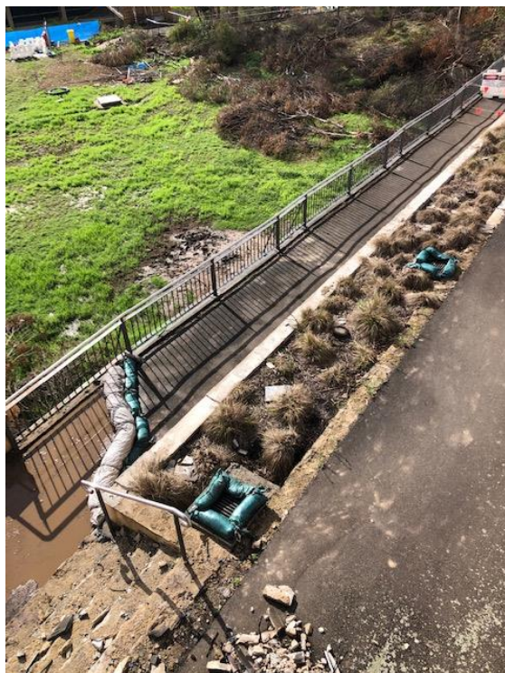
Photo 5: Erosion and sediment controls down-gradient of stockpiles and around stormwater outlet
