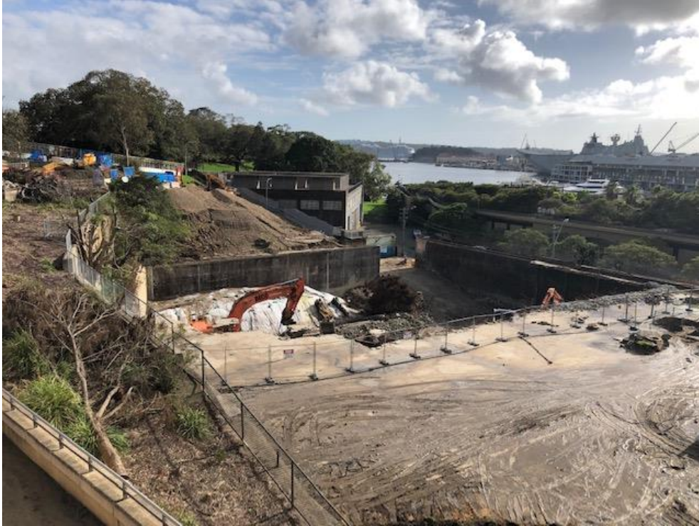
Photo 1: Demolition and excavation, former fuel bunkers. Evidence of tree removal
