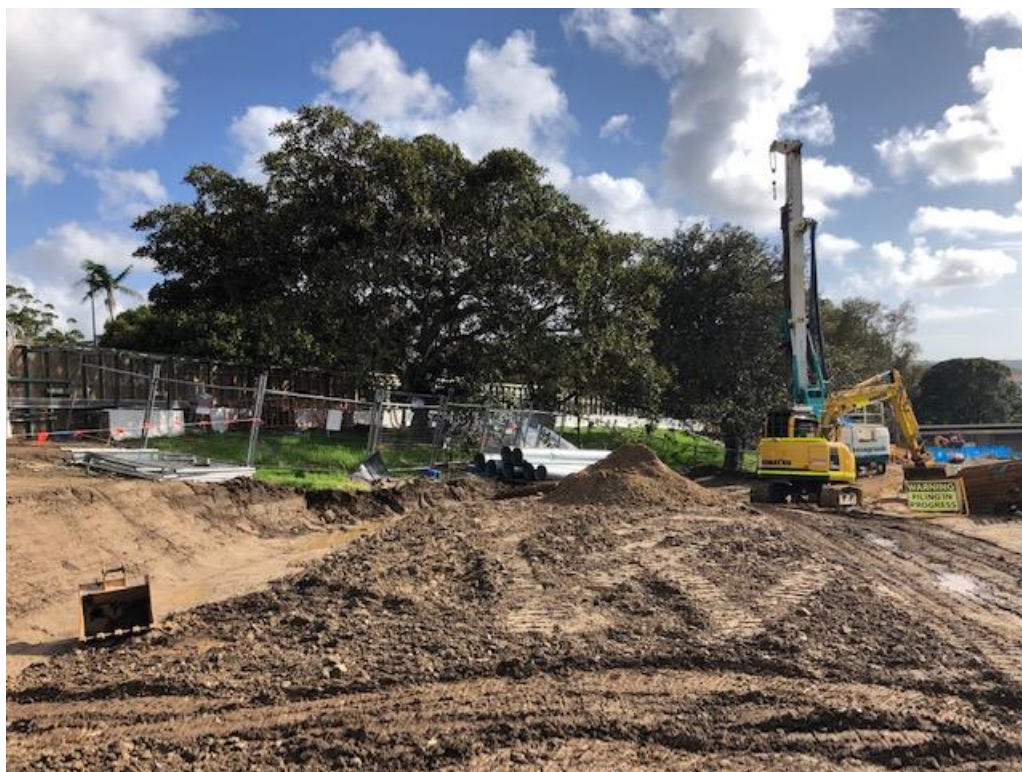
Photo 8: Tree protection fencing around the fig tree on the eastern site boundary
