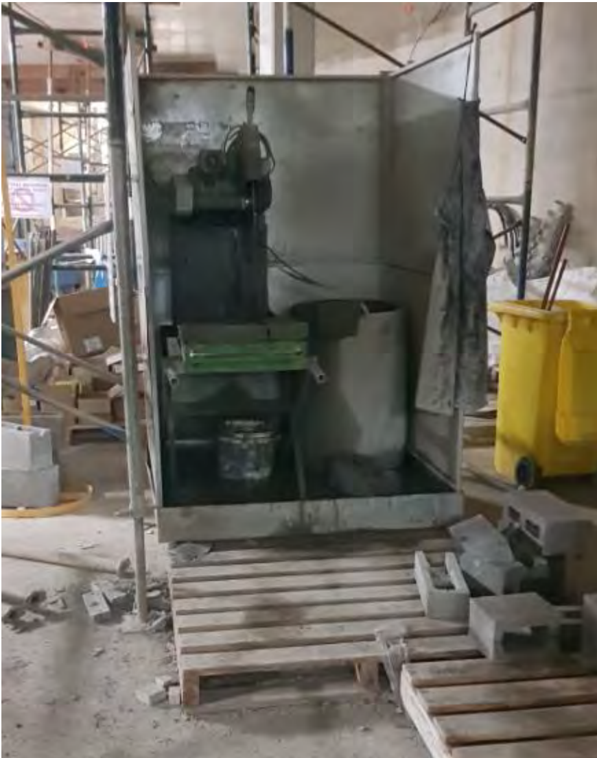
Photo 14: Wet saw slurry collection
