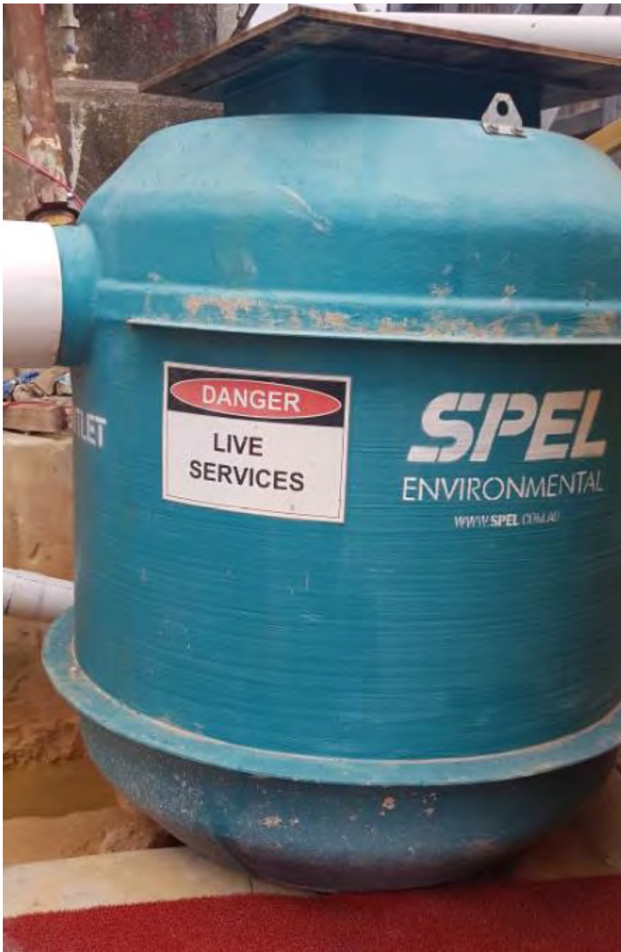
Photo 11: Water treatment plant
