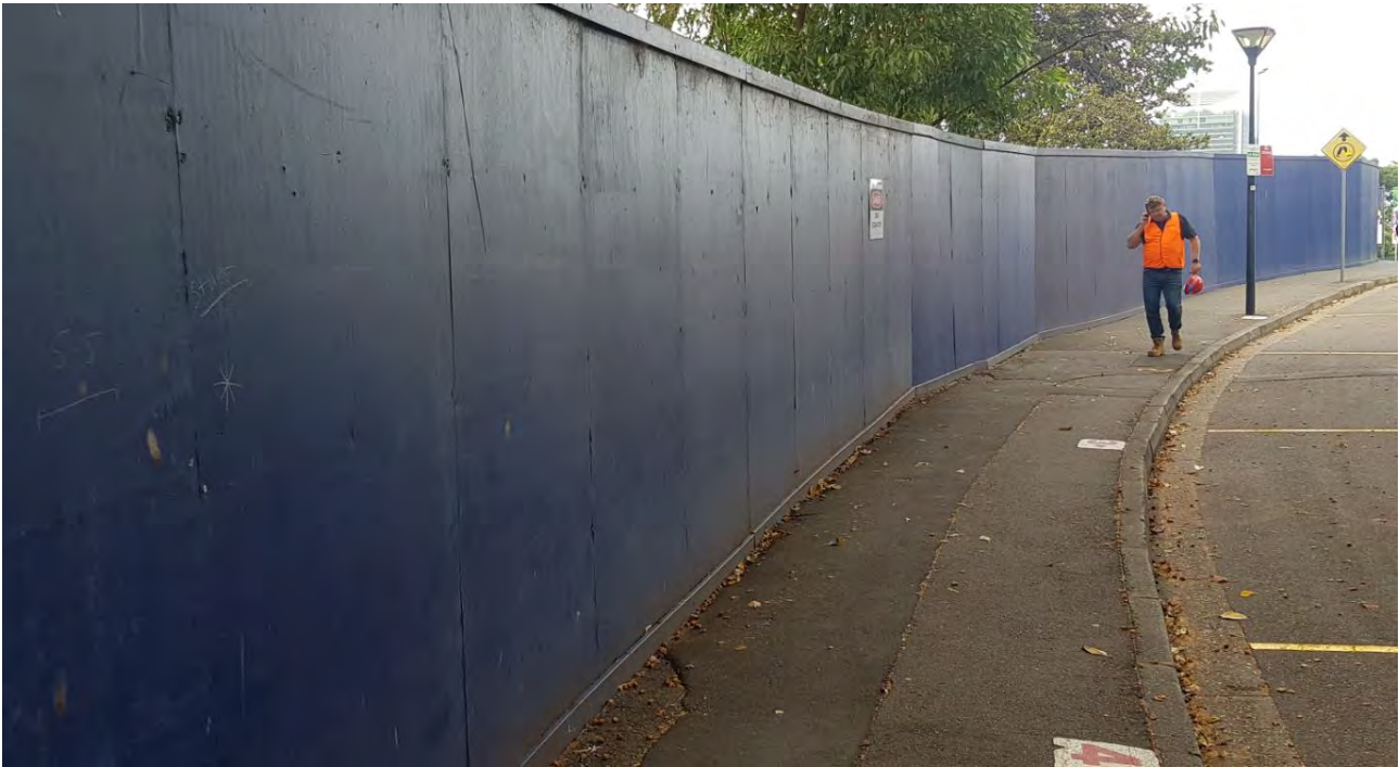
Photo 6: Site hoarding free of graffiti and advertising material
