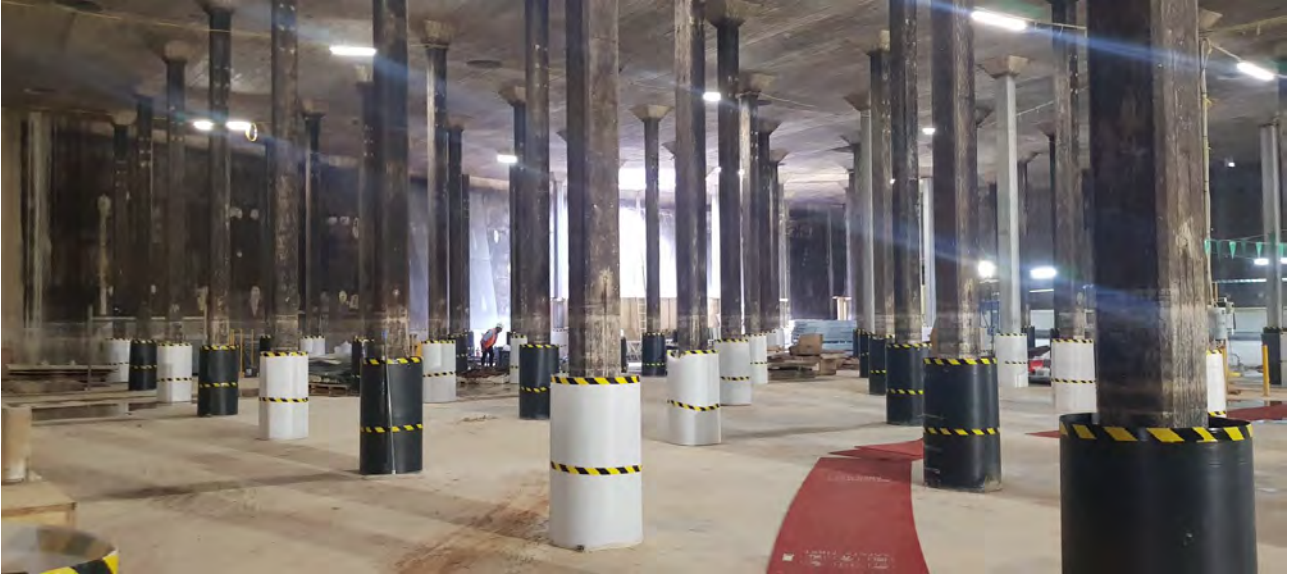
Photo 12: Fuel bunker refurbishment, with pier protection in place.
