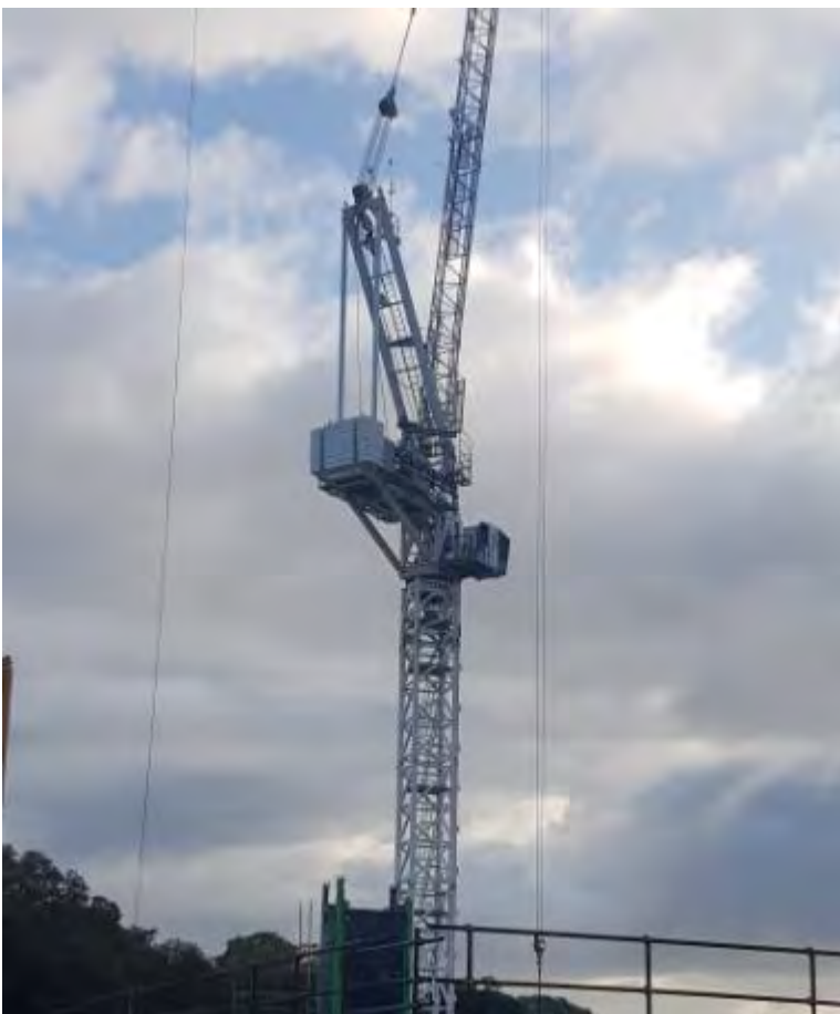
Photo 3: Electric powered tower crane in use.
