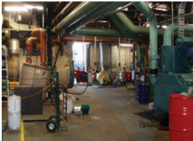
Roof Plant Image: JPW
