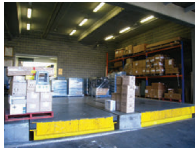
Loading dock does not allow for separation of artwork and general goods Image: JPW
