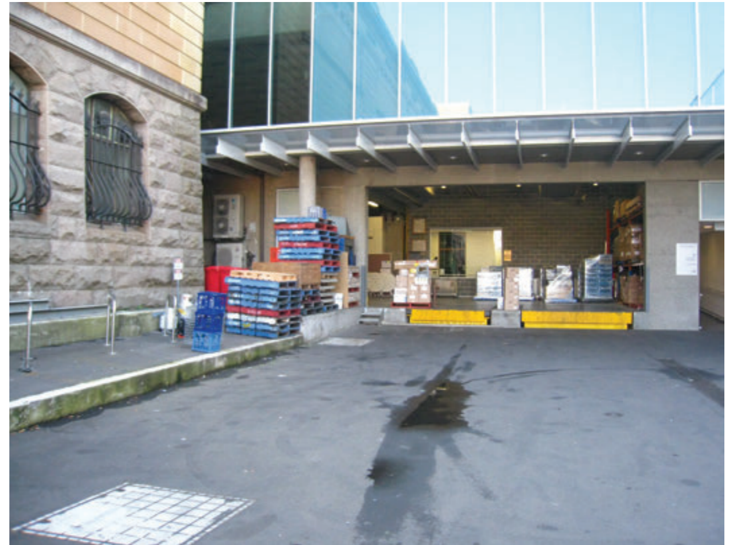
Loading dock with limited protection for trucks and unloading Image: JPW
