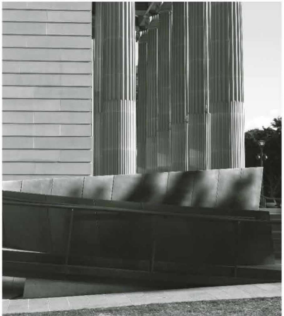
New access ramp entrance, Art Gallery of New South Wales
