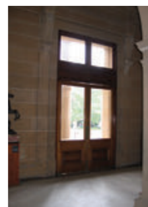
The entry doors limit the size of the only public entrance, Vestibule, GF Image: AGNSW
