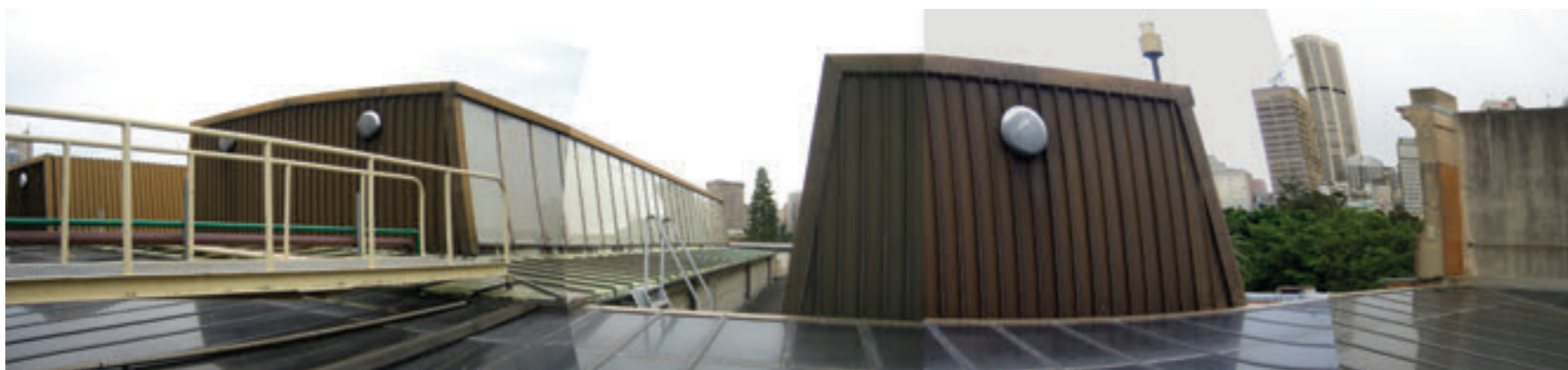
Vernon Gallery Lanterns, Vernon Wing, Roof Level. These lanterns originally provided natural light to the gallery space, but this has ceased due to conservation considerations. The lantern now house the artificial lighting necessary for the Vernon Galleries.
