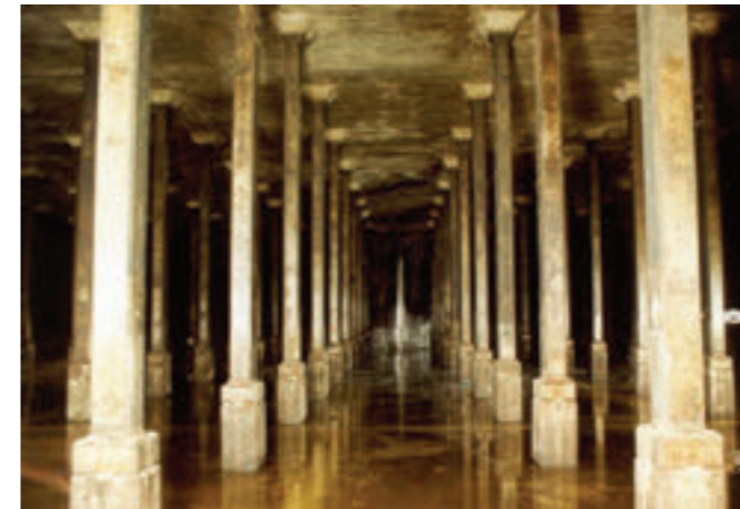
Interior View of the Disused Fuel Tanks Image: Source Unknown
