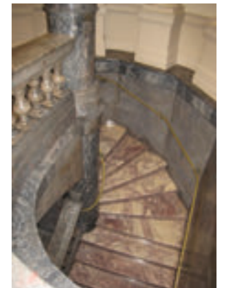
The south-west stairs from Gallery 13 to the Library in ornamental stone work with Borenore Marble treads, Vernon Wing, Ground Floor Image: JPW
