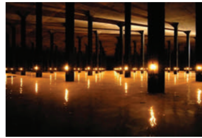
Interior View of the Disused Fuel Tanks Image: http://www.uer.ca/locations/show.asp?locid=21910
