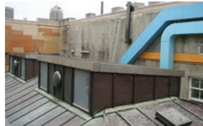
Clerestory windows of lead-light sky-lights, Vestibule, Roof Level Image: JPW
