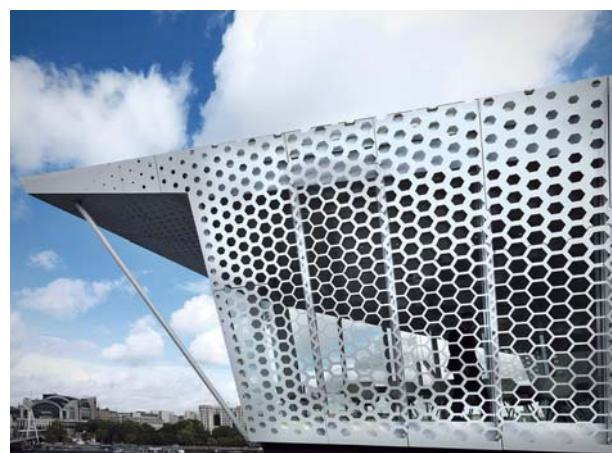
*The laser cutting creates a texture with geometric patterns that cover the entirety of the external surface. The total surface area of the restaurant is 140 sq.m.; this is split into a large open space with a kitchen in full view of the diners and a panoramic terrazzo of 50 sq.m. The design of the interiors is extremely minimal with a predominance of white contrasting with the dark wood used in the flooring. (A. C.; ph: Andrea Martiradonna)*
