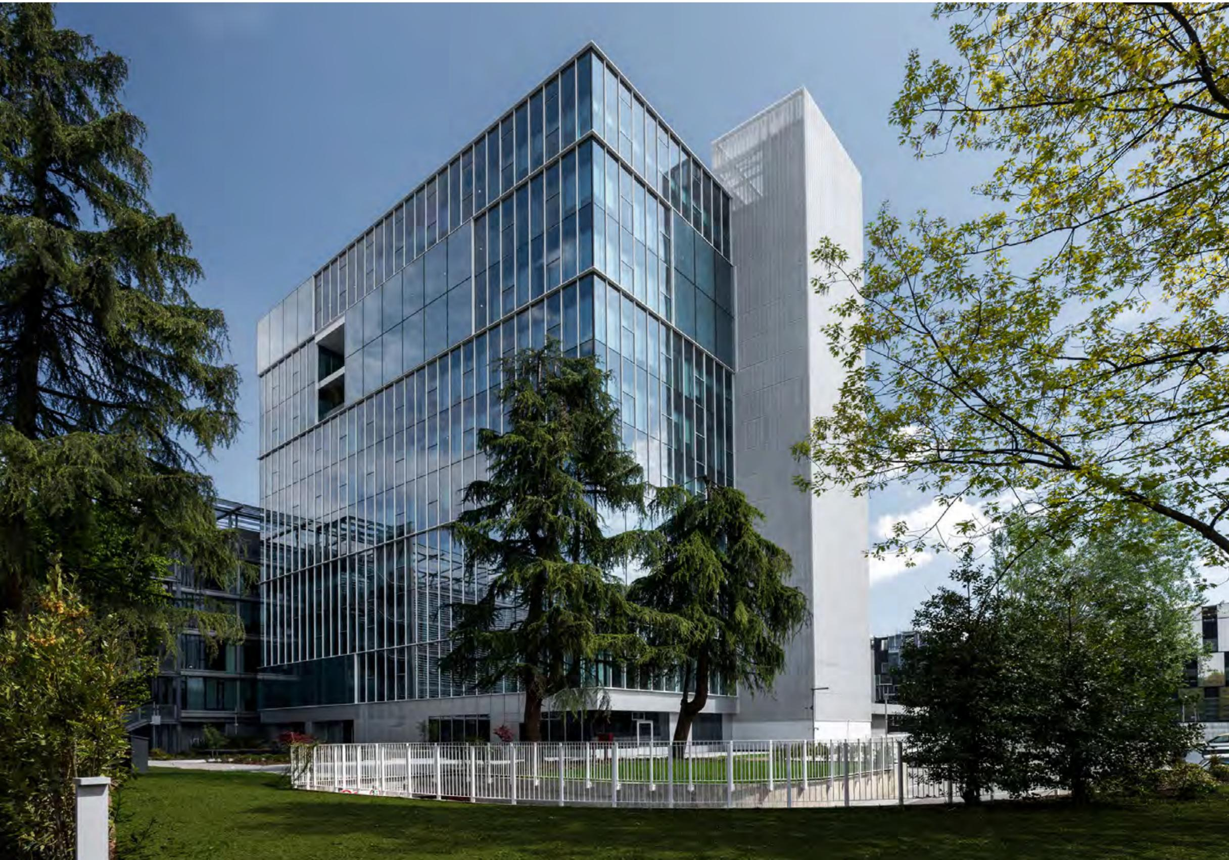
**THE BUILDING WAS STREAMLINED BY REMODELLING AND REBUILDING THE FAÇADE. THE ALTERNATION OF TRANSPARENT GLASS SECTIONS AND SCREEN-PRINTED GLASS PANELS SEPARATED BY METAL PILASTER STRIPS OUTLINE GLAZED SPANS THAT REFLECT LIGHT DIFFERENTLY. THE SURFACE'S UNIFORMITY IS BROKEN BY DOUBLE-HEIGHT LOGGIAS THAT CREATE A SENSE OF THREE-DIMENSIONALITY.**
