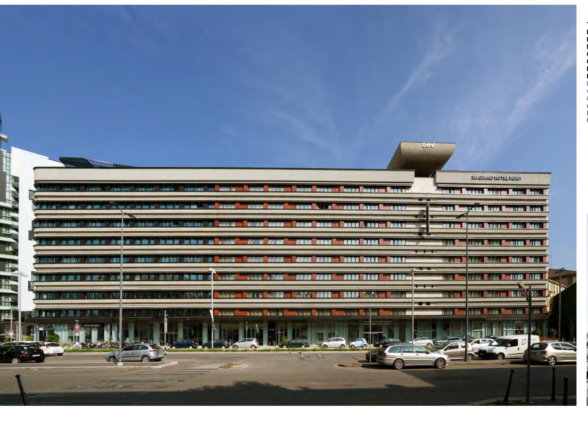
THE RHYTHM OF THE GLAZING INSIDE IS HIGHLIGHTED BY FINS IN EXTRA-CLEAR GLASS THAT INCREASE FLEXIBILITY BY ENABLING THE INSTALLATION OF MOBILE PARTITIONS AS DESIRED, WHILE ON THE OUTSIDE BY THE ALTERNATION OF FINS IN EXTRA-CLEAR GLASS AND COLOURED GLASS IN LIGHT-GREY. IN FRONT OF THE COLUMNS ARE BOXES IN MICRO-PERFORATED BENT-PRESSED STEEL.
