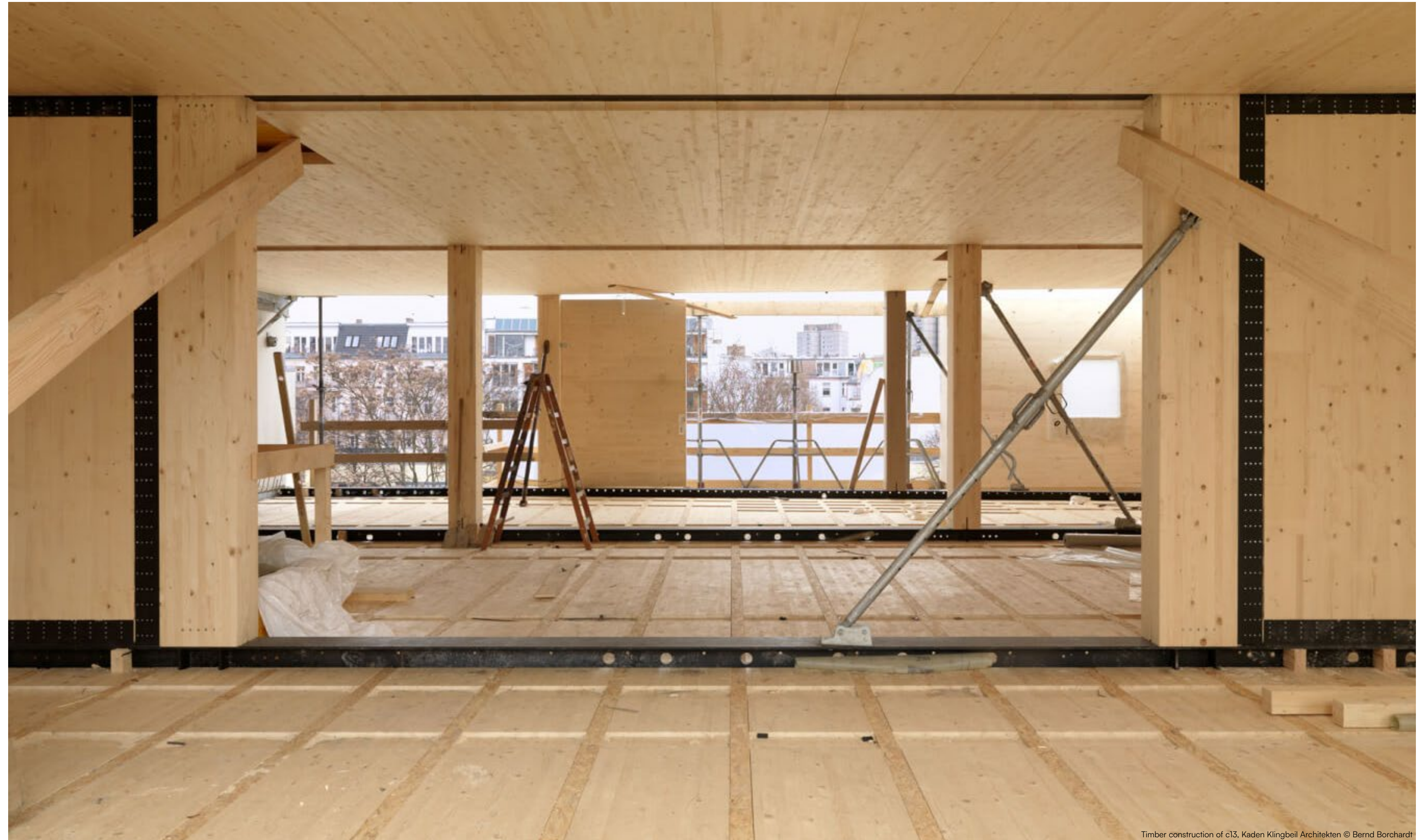
Timber construction of c13, Kaden Klingbeil Architekten © Bernd Borchardt
