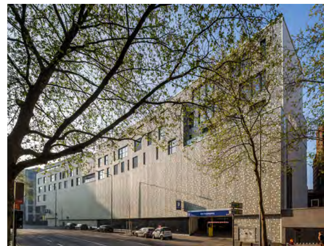
Abb.6: Magnus 31 © Wilkin & Hanrath Bauphasen
