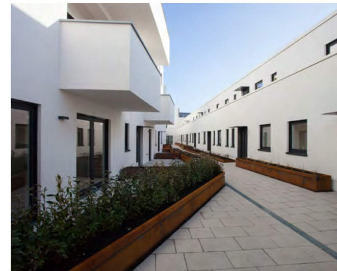
Abb. 8: Magnus 31 © Wilkin & Hanrath Bauphasen
