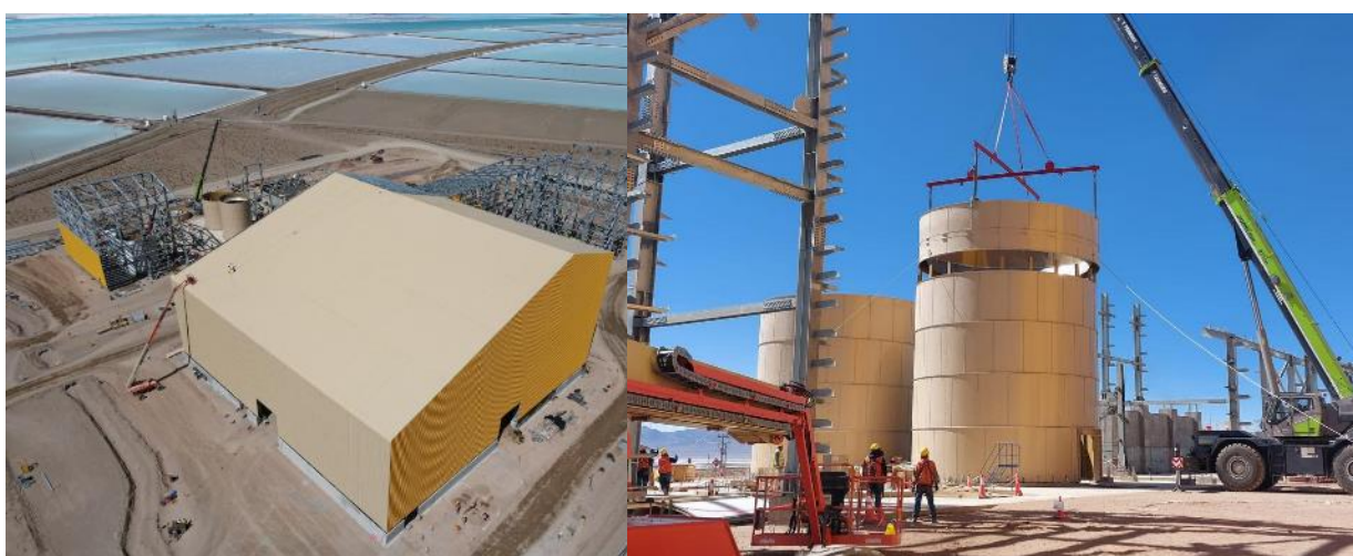
Figure 1: Olaroz Stage 2 - construction 77% complete
