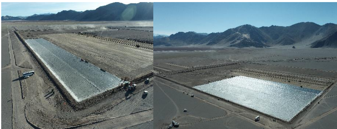
Figure 2: Sal de Vida – pond construction underway
