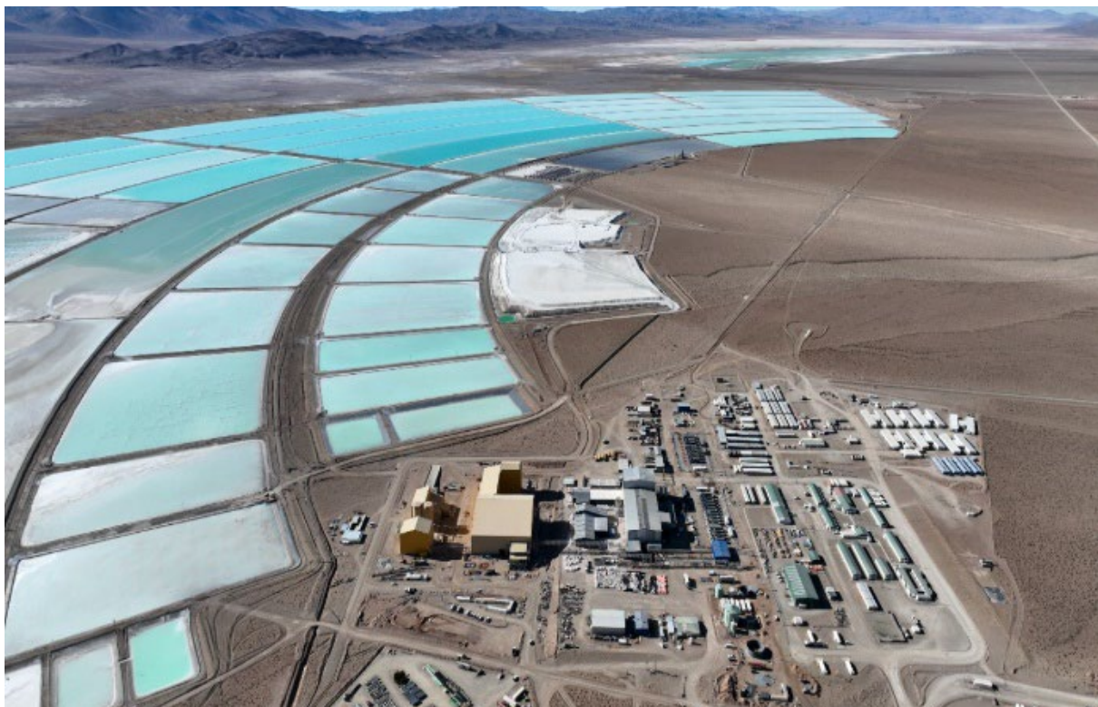
Figure 1: Olaroz Stage 2 - ponds fully commissioned
