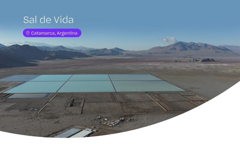
Sal de Vida is designed to produce battery grade lithium carbonate through an evaporation and processing operation located in Catamarca Province, Argentina, approximately 200km from Olaroz. Stage 1 of this project will deliver an initial 15ktpa operation that will be expanded to ~45ktpa through Stage 2.
