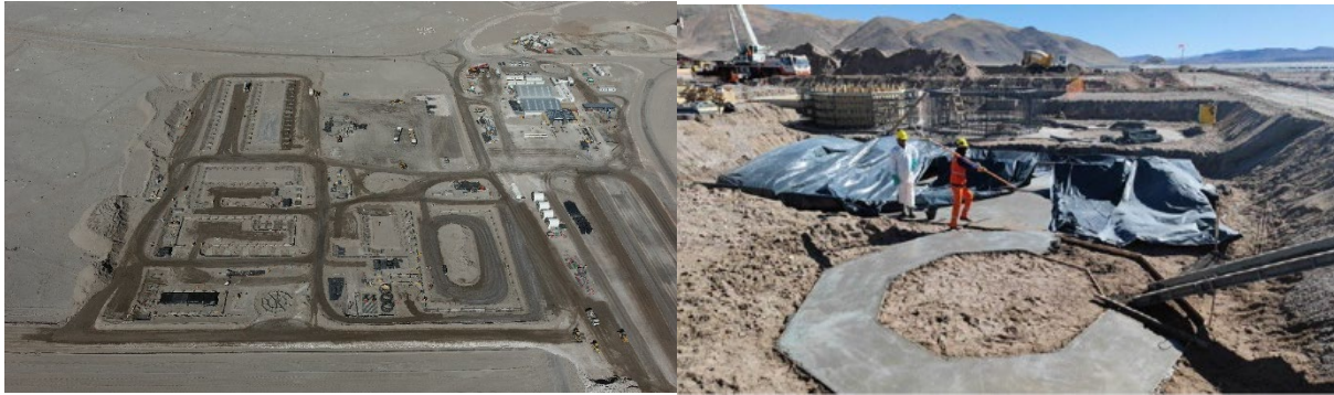
Figure 3: Process Plant overview (left) and concrete foundations (right)
