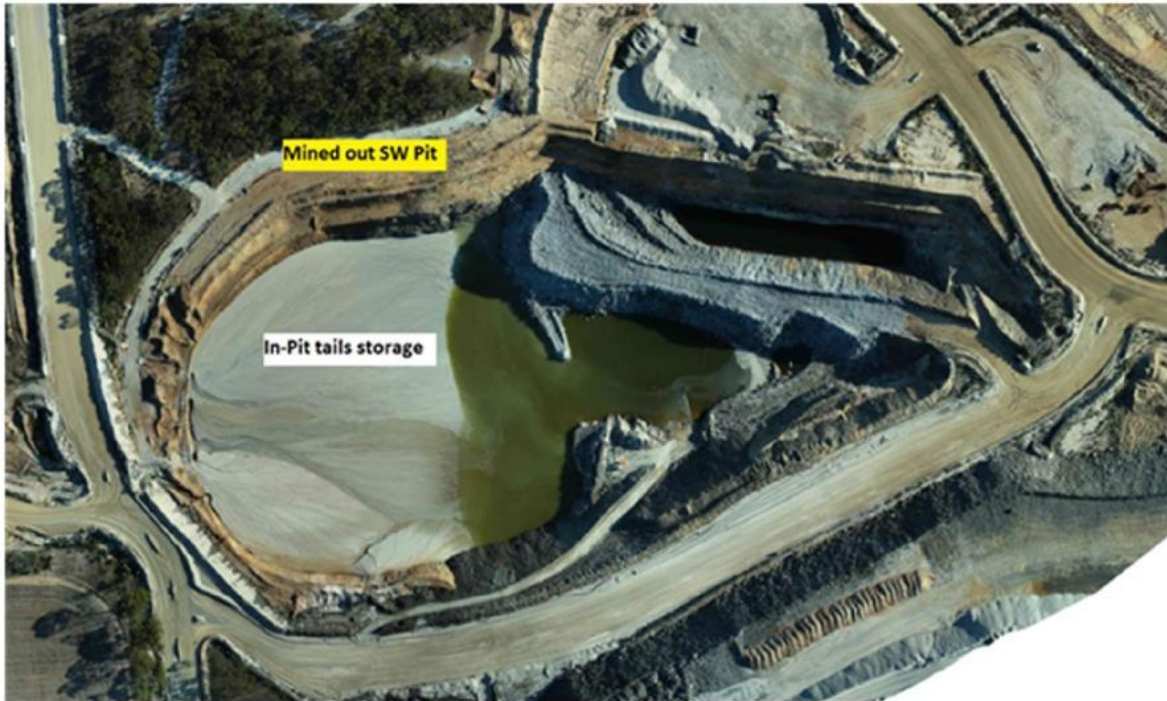
Figure 18-4 Aerial image of the existing in-pit tailings storage as of March 2021
