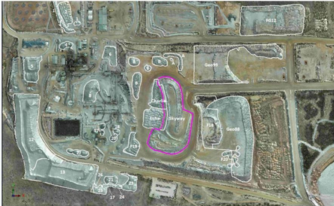
Figure 18-2 Aerial Image of the ROM Pad and Ore Stockpiles as of 31 March 2021
