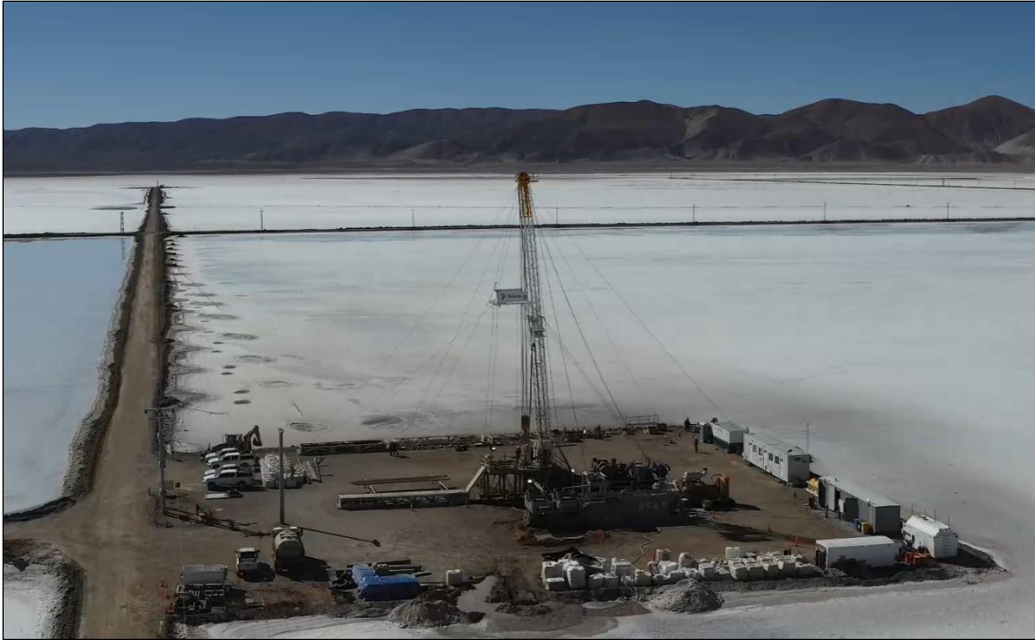
Figure 10-2 – Drilling rig at Olaroz, on 650m deep production well.
