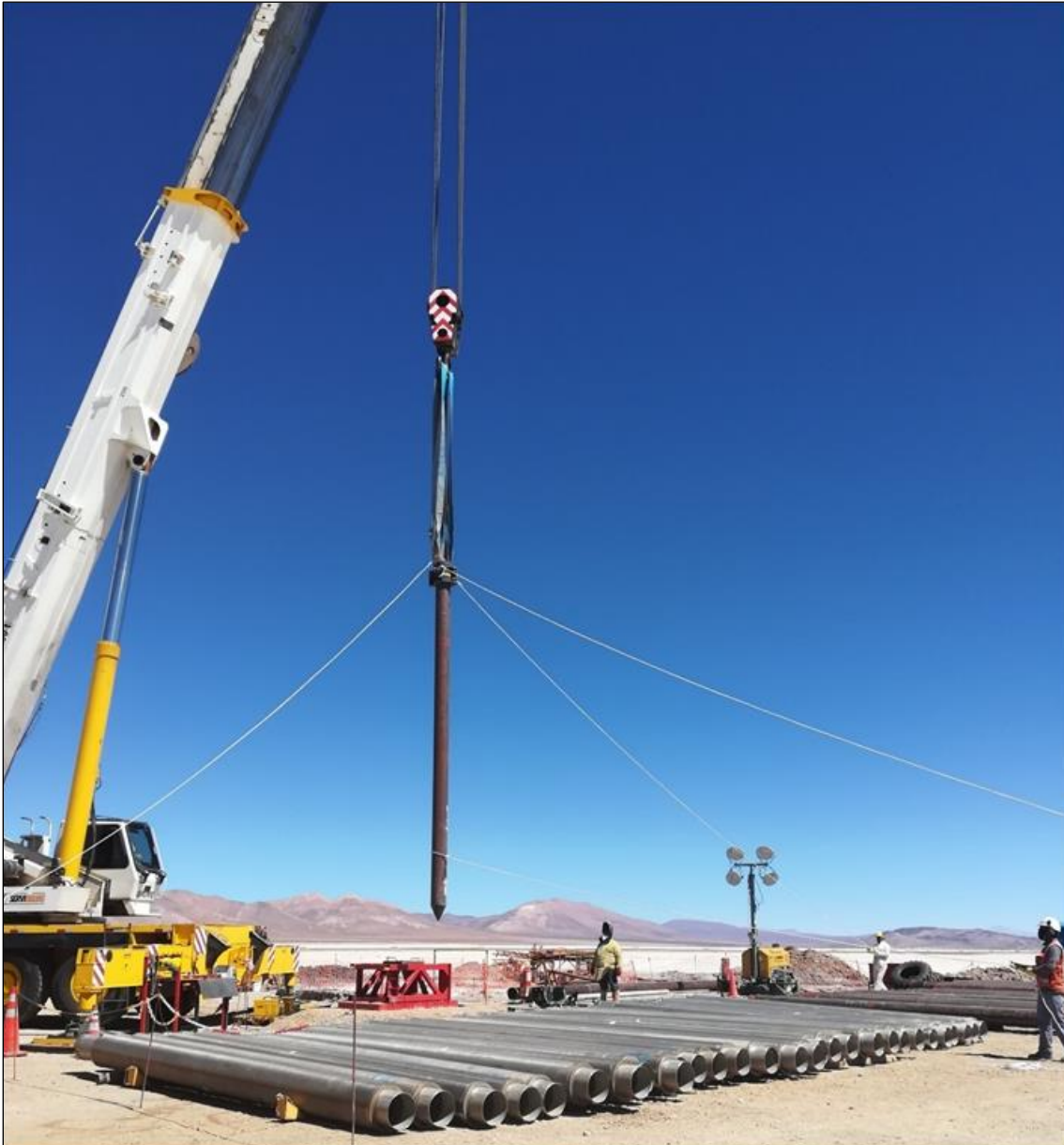
Figure 10-4 – Installation of filters in a production well at Olaroz.
