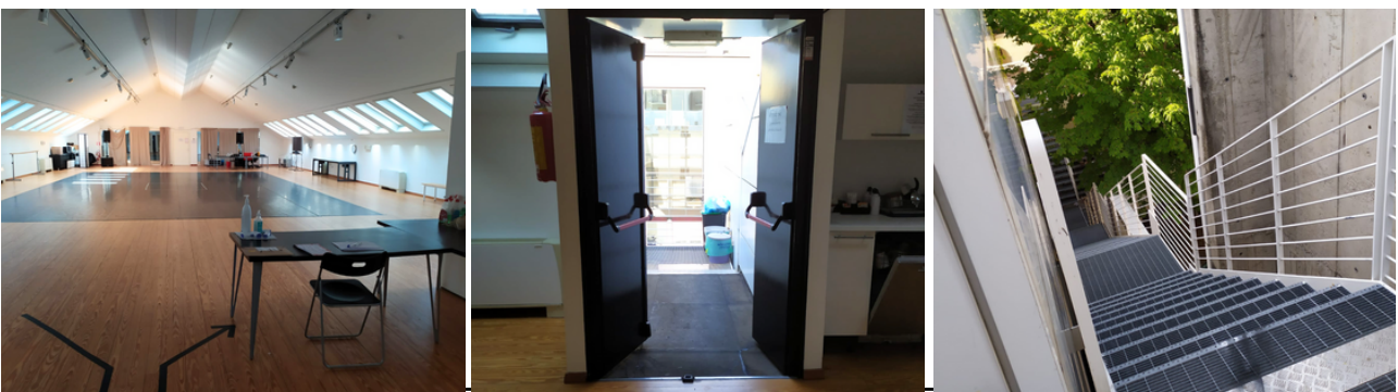
Second floor room details and emergency exit
