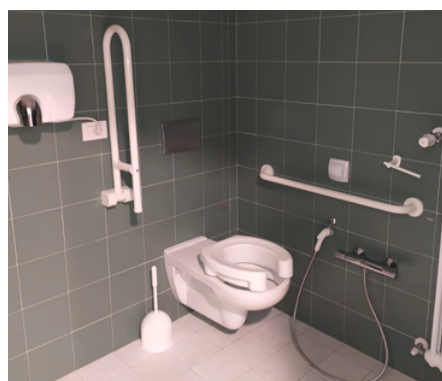
Accessible bathroom and shower facilities
