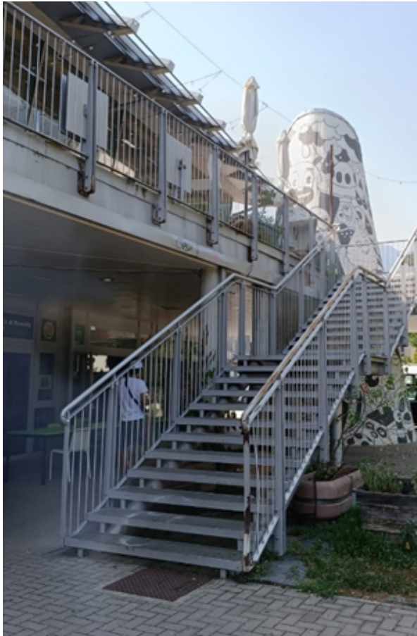
Entrance from the back with 24 steps
