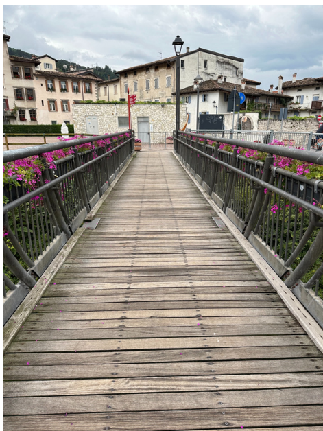
Wooden walkway from Via Lungo Leno Destro
