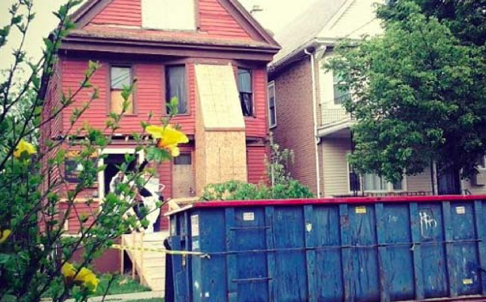
An asbestos removal project in PUSH Buffalo's Green Development Zone.
