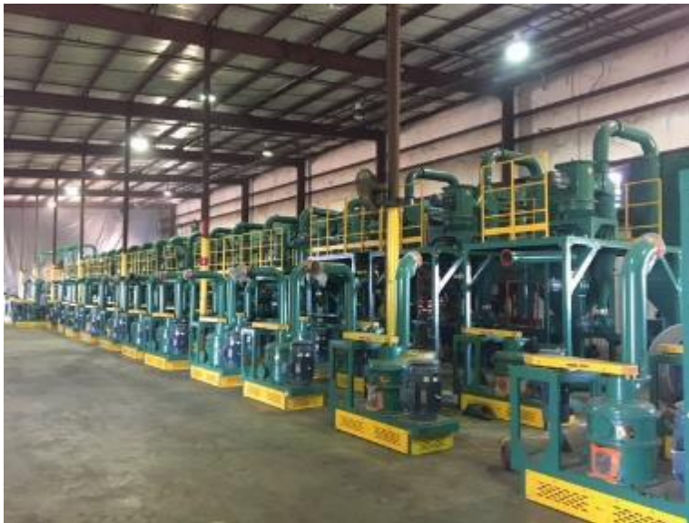
Assembling milling equipment on site at Vidalia
