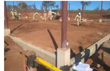
Balama Training Centre construction commenced
