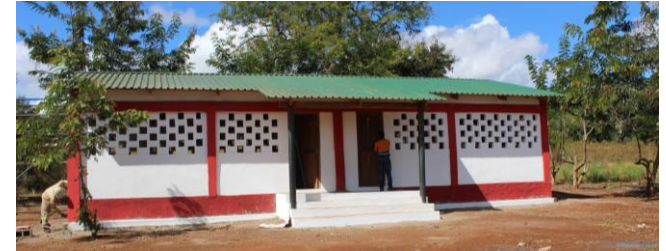
Local school refurbishment
