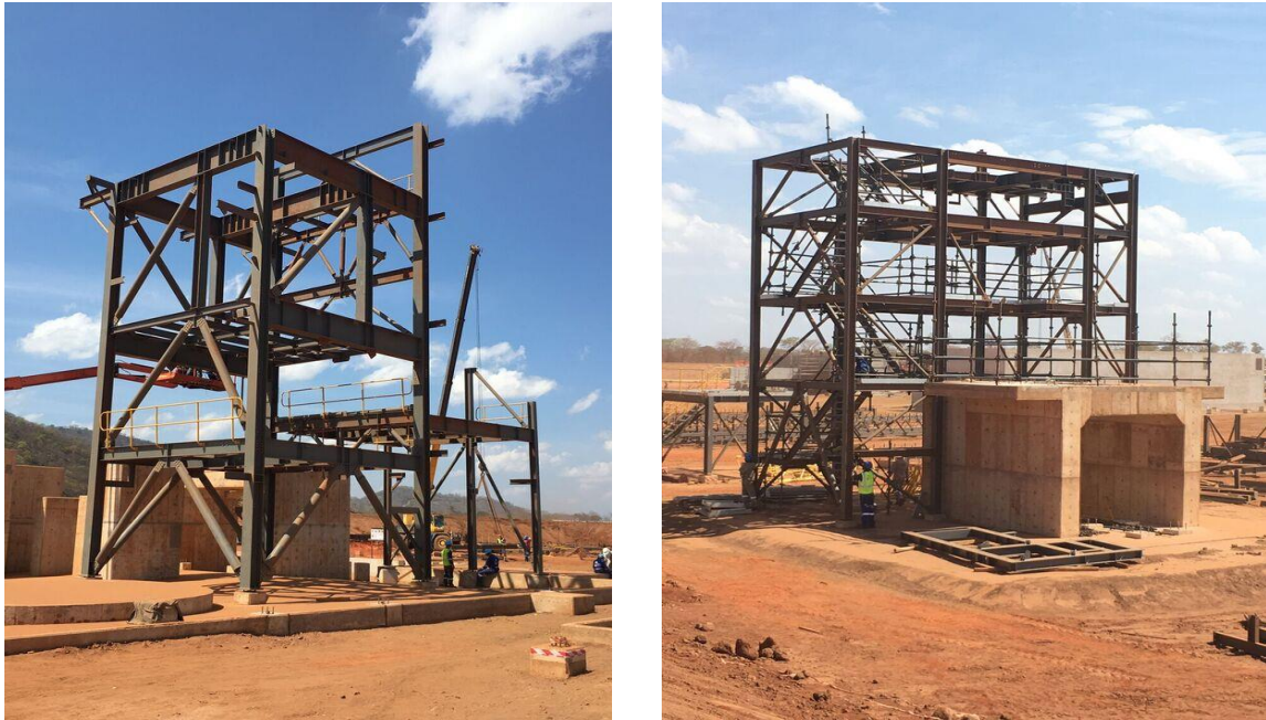
Figure 6 - Primary milling (left) and recycle crusher (right)
