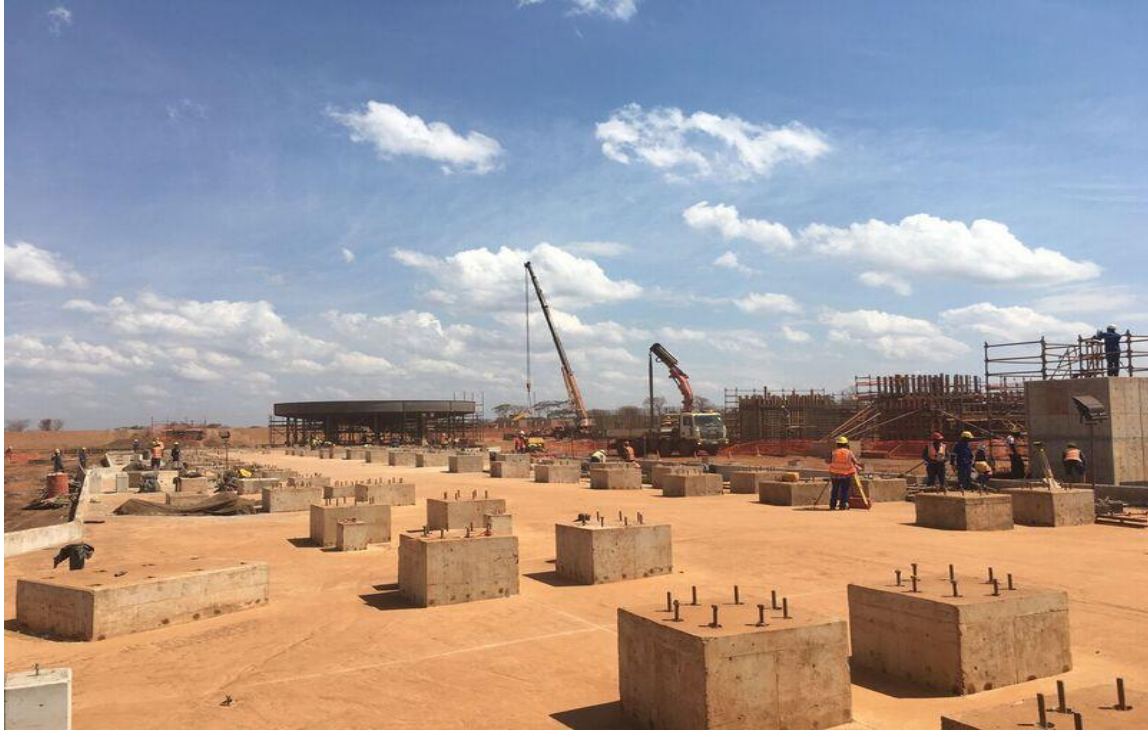
Figure 1 – Flotation footings
