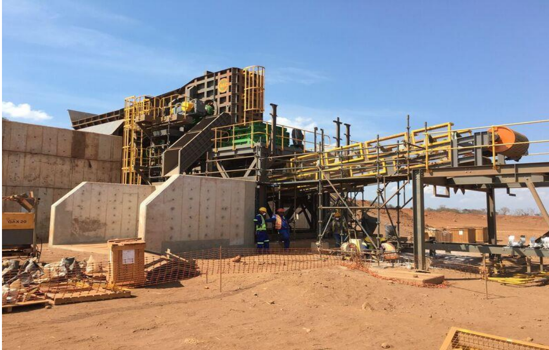
Figure 4 – Primary crusher
