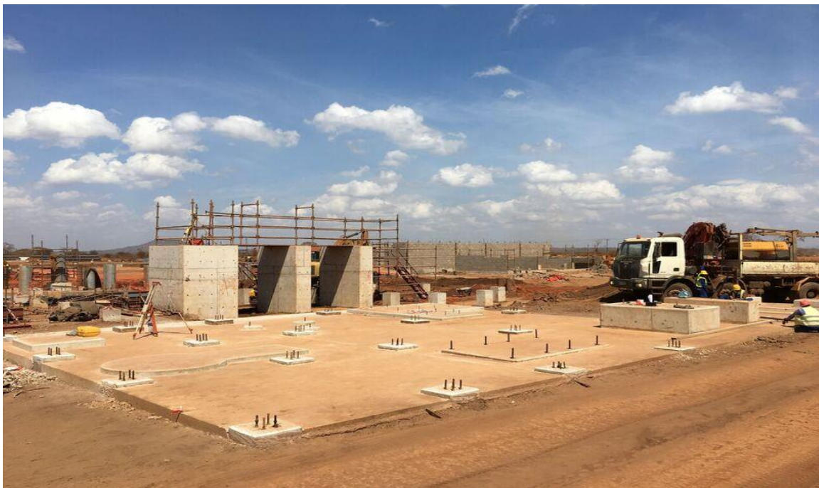
Figure 2 – Slabs for the flake dryer area
