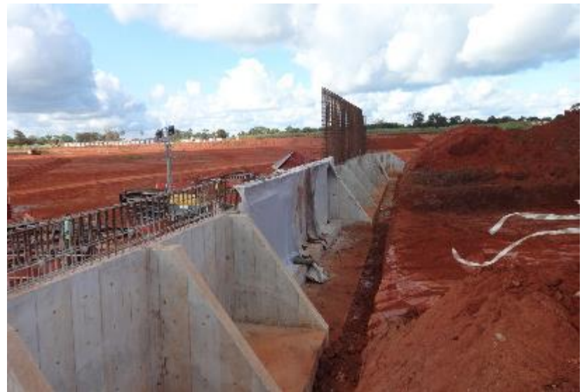
Balama crushing facility foundations (left) and ore bin back wall (right)
