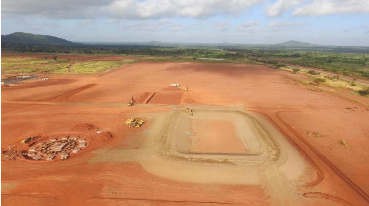
Process water dam (right) and thickener footings (left)
