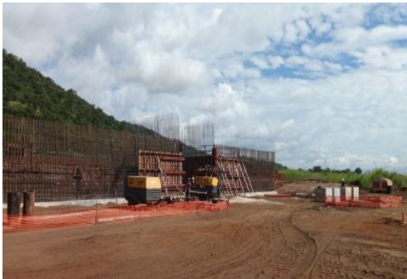
Balama crushing facility foundations (left) and ore bin back wall (right)
