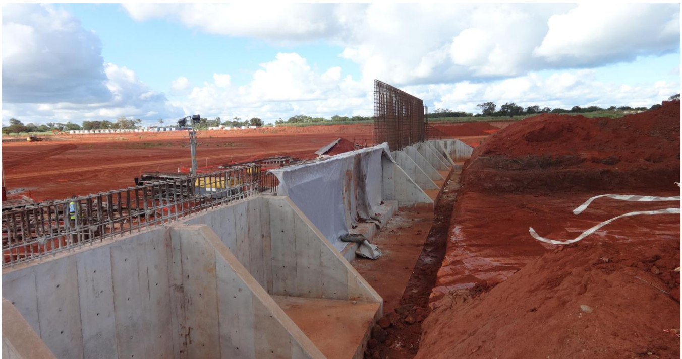
Figure 5 – Balama ore bin back wall
