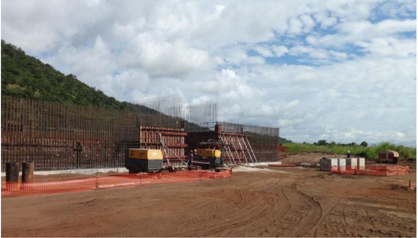
Figure 4 – Balama crushing facility foundations
