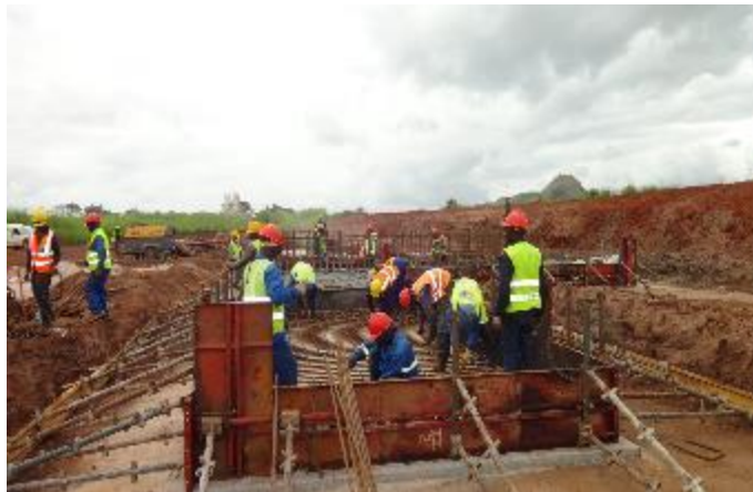
Concrete pour for the ore bin retaining wall (top left), crusher wall (top right) and fixing rebar for the primary milling circuit (bottom) at the Balama process plant site
